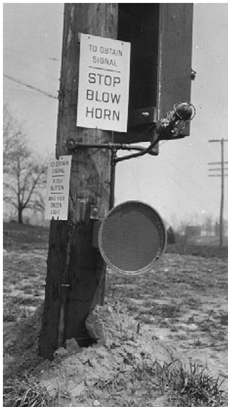
"To Obtain Signal - Stop Blow Horn," traffic-actuated signal light, Charles Adler, Jr. Collection, ca. 1920-1980
