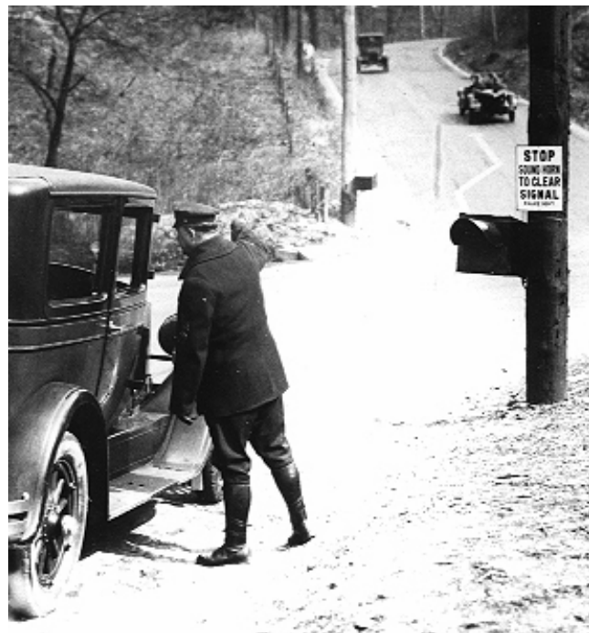
Traffic-actuated (by the sound of a car horn) signal light Charles Adler, Jr. Collection, ca. 1920-1980
