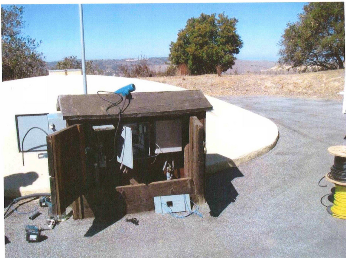
Photo 24: PLC and SCADA installation at Vista Dorado Tank
