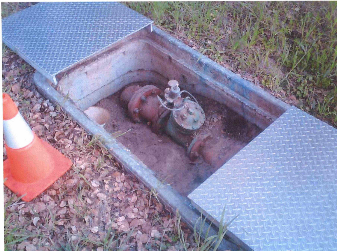
Photo 24: Toro regulating station (not in service)
