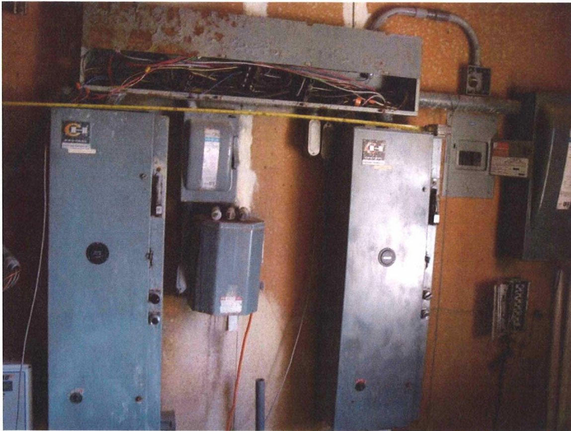
Photo 7: Controls for Wells No. 1 & 2 showing significant corrosion
