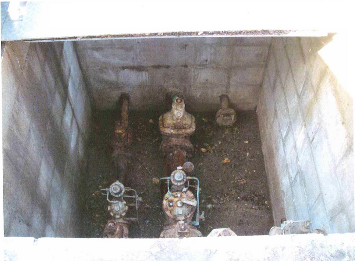
Photo 20: Toro regulating station with heavy corrosion and missing valve
