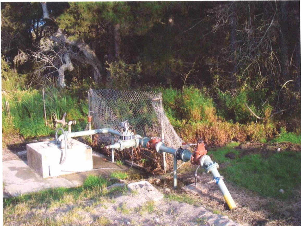
Photo 24: Toro well No. 2 with new wellhead piping
