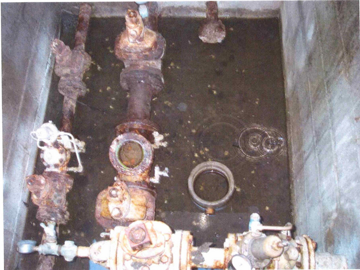
Photo 21: Toro regulating station with heavy corrosion and missing valve
