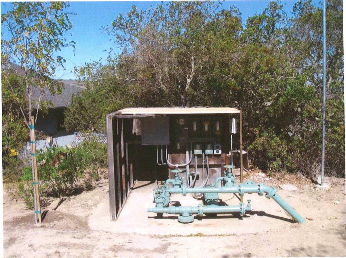
Photo 19: Cordillera pump station with temporary rain shelter
