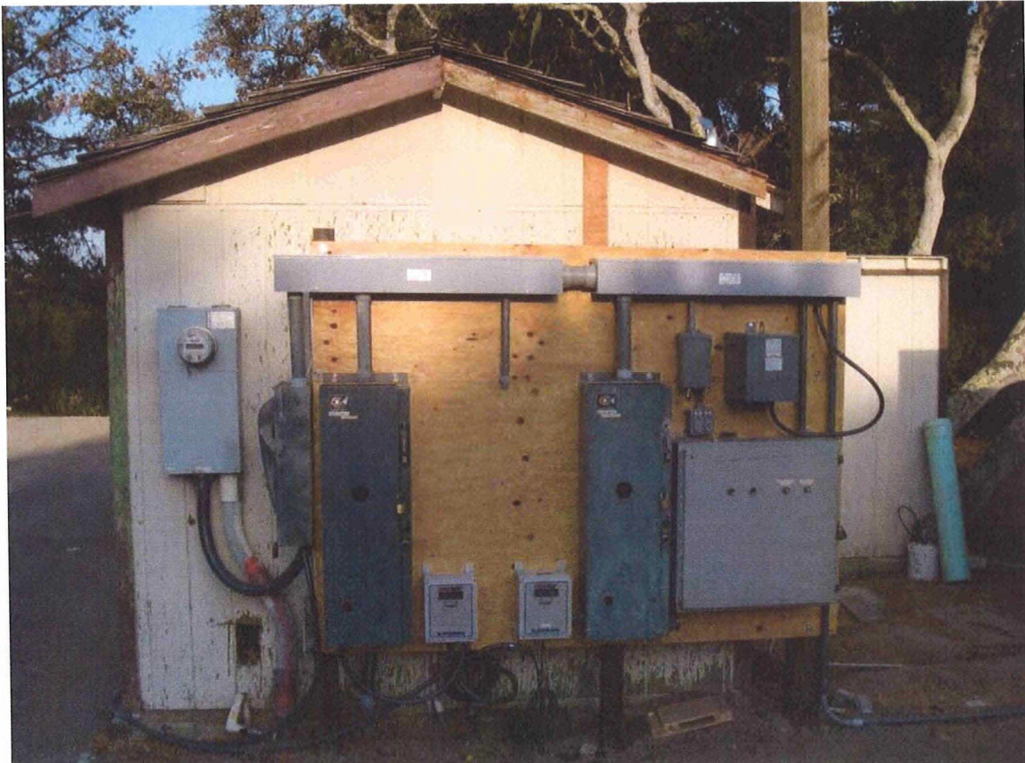
Photo 24: Toro control equipment moved outside during rehab of control building
