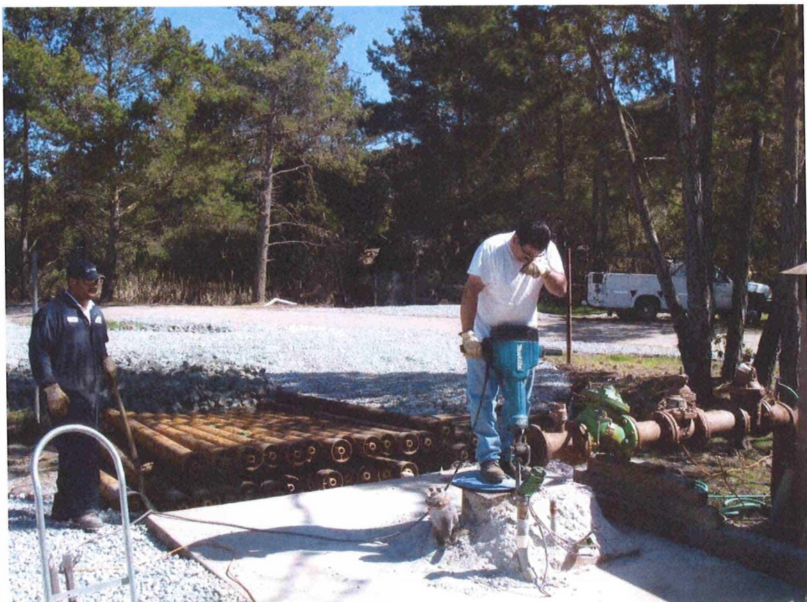
Photo 24 Well No. 1 during foundation rehab
