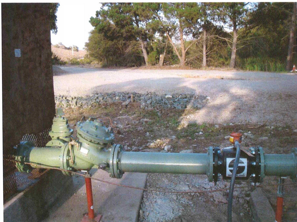
Photo 24: Welll No. 1 with new discharge piping
