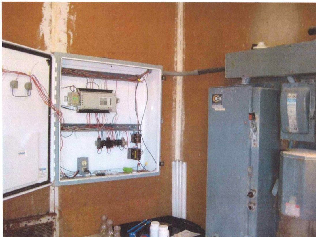
Photo 8: PLC prior to Cal Am's operation of facility
