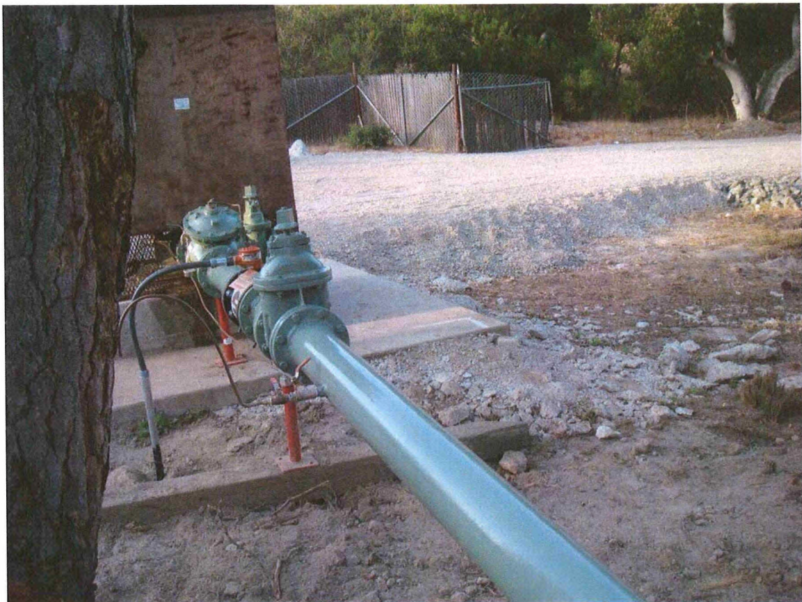
Photo 24 Welll No. 1 with new discharge piping
