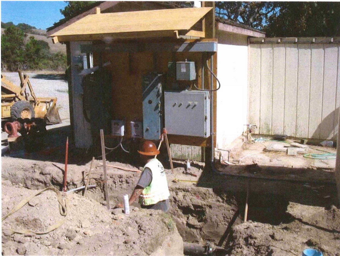
Photo 24: Toro yard piping rehab and control building
