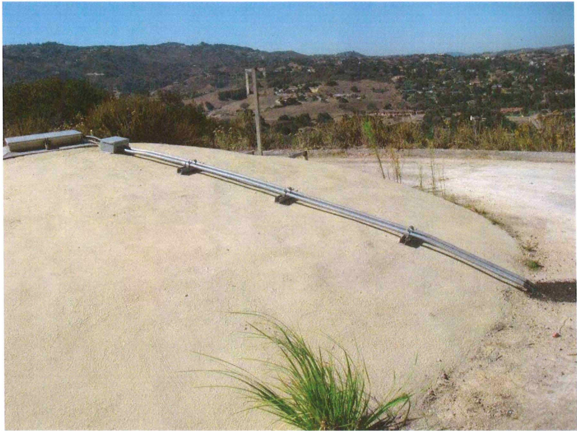
Photo 24: Conduit and wiring for tank level sensors and alarm system
