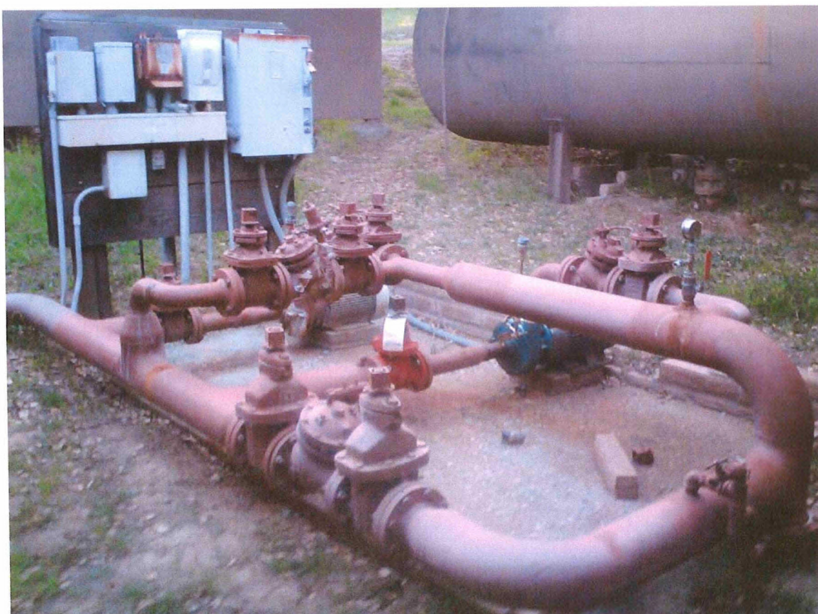
Photo 18: Upper Markham pump station showing corrosion and leakage
