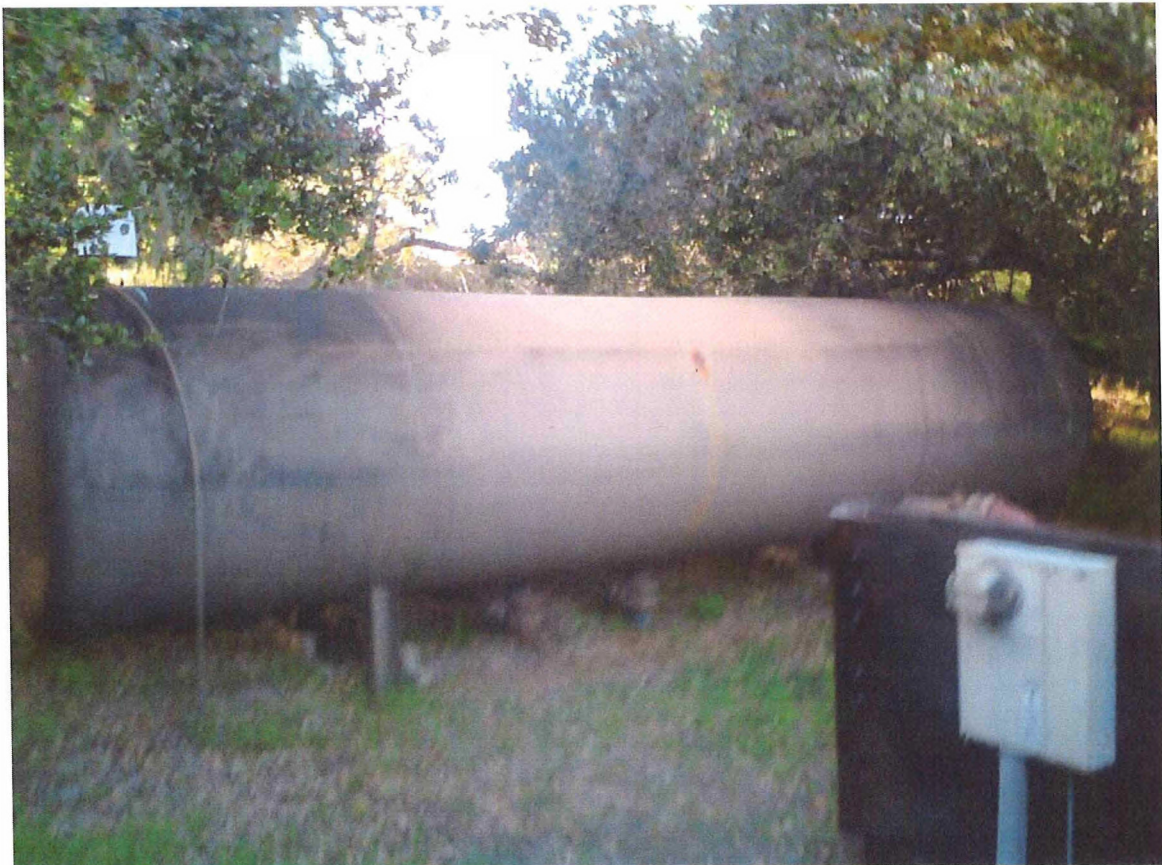
Photo 14 Upper Markham Pneumatic Tank showing signs of corrosion and leakage
