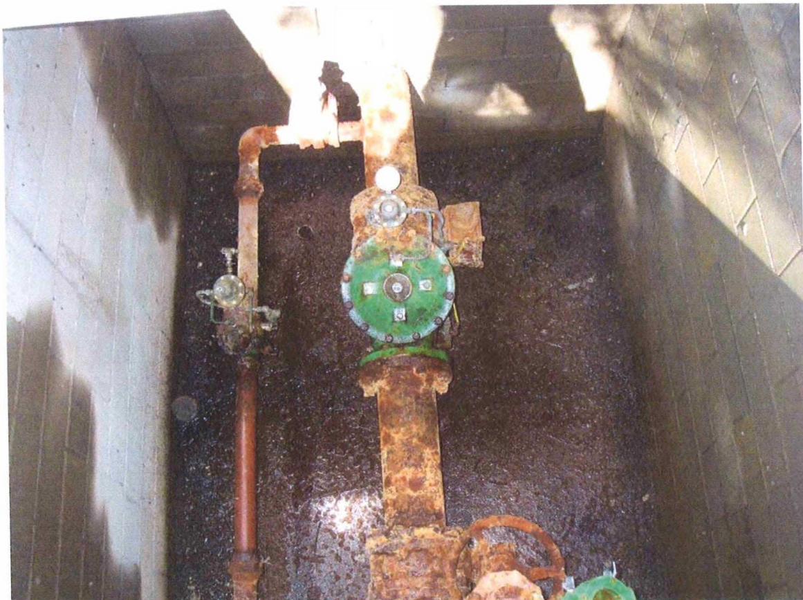
Photo 22: Toro regulating station showing substantial corrosion and leakage
