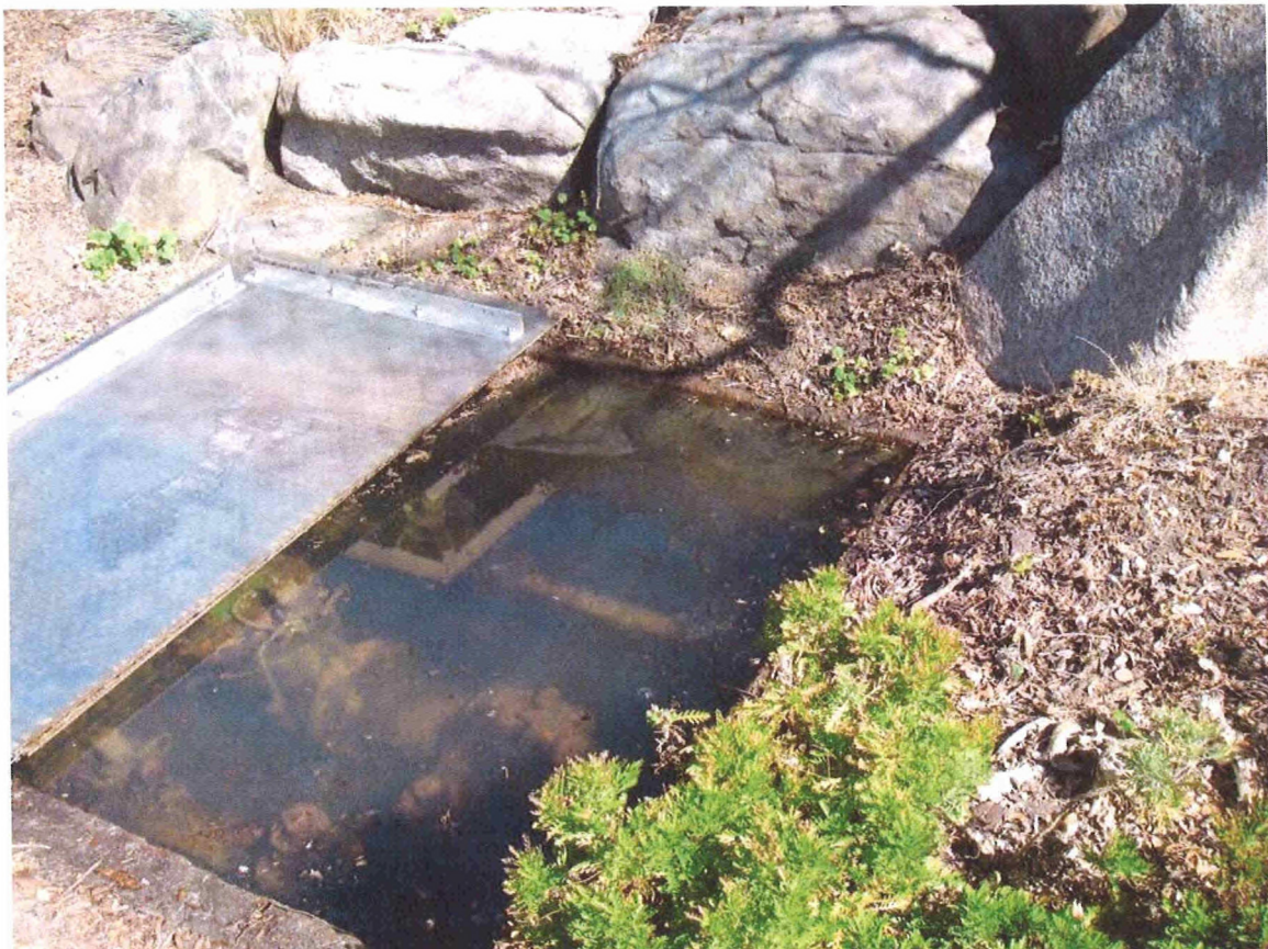
Photo 23: Toro regulating station (inundated/drowning hazard)
