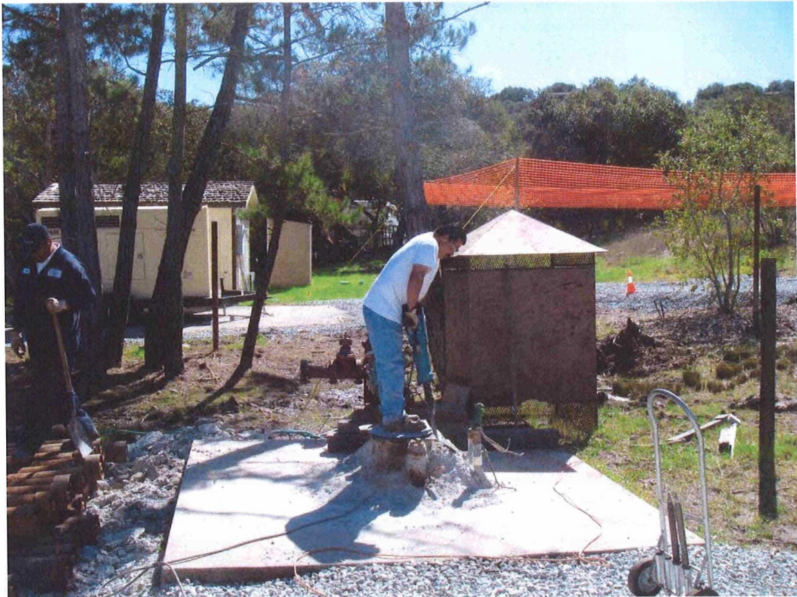
Photo 24 Well No. 1 during foundation rehab
