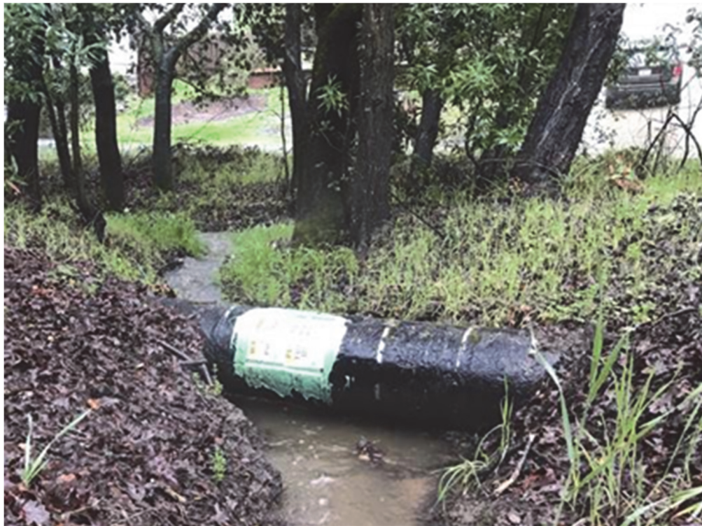
Figure 1: Lafayette Exposed Pipeline Segment 1 10
