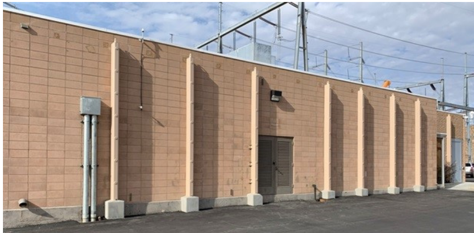
Figure III-6 Completed Seismic Retrofit of a Reinforced Masonry Wall at an SCE AA Substation; Vertical Pipes Added and Ties from Walls to Roof Added
