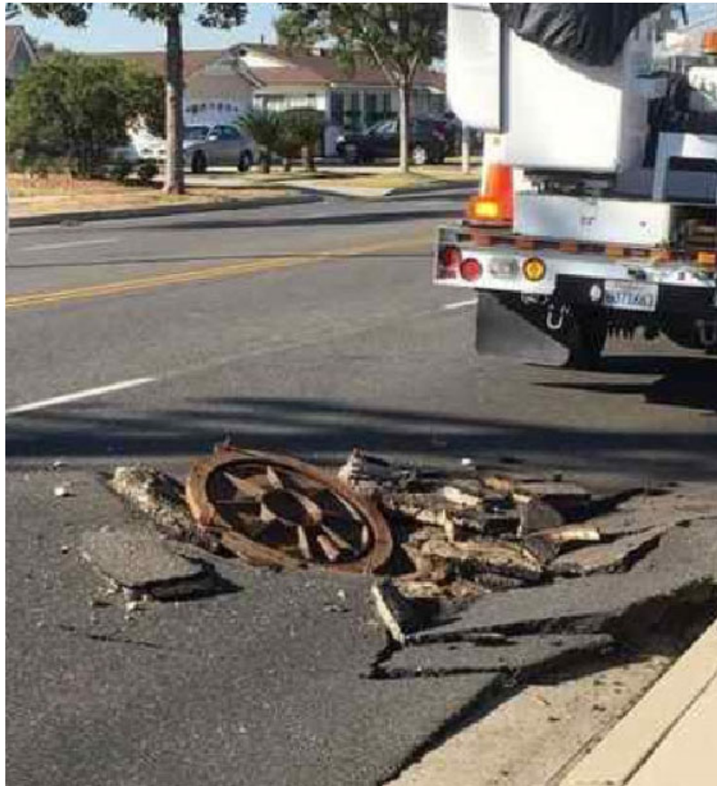
Figure II-8 Illustration of Explosion Outcome (O1) due to Cable Driver (D1)
