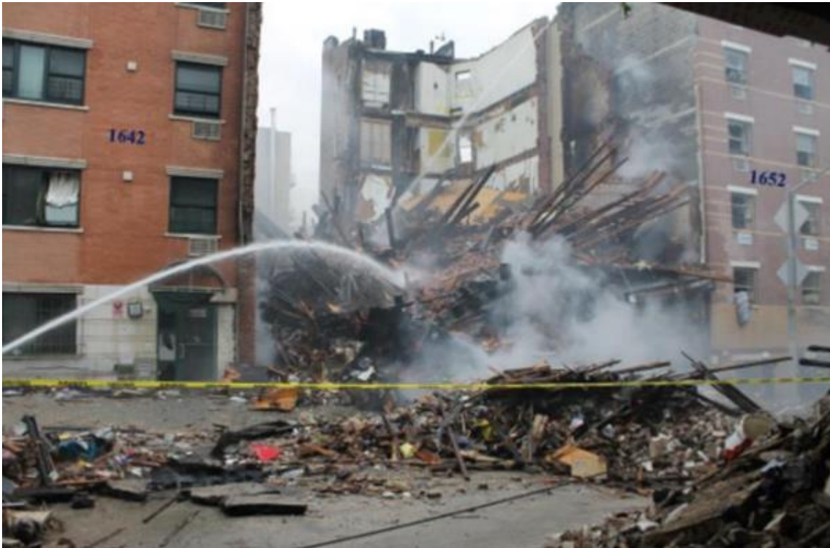
FIGURE 2-3 2014 EXPLOSION IN NEW YORK
