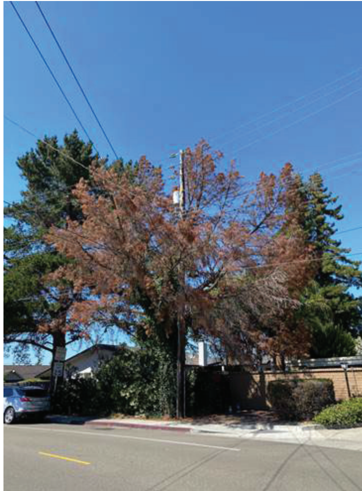
Figure 13: Safety issue submitted through PG&E Report It: A dead tree with branches within four feet of the conductor
