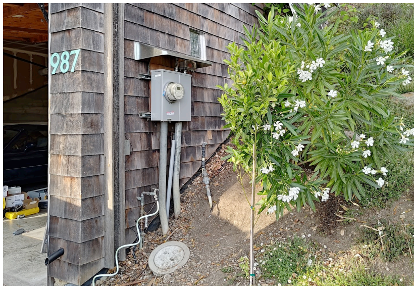
New panel as installed.
