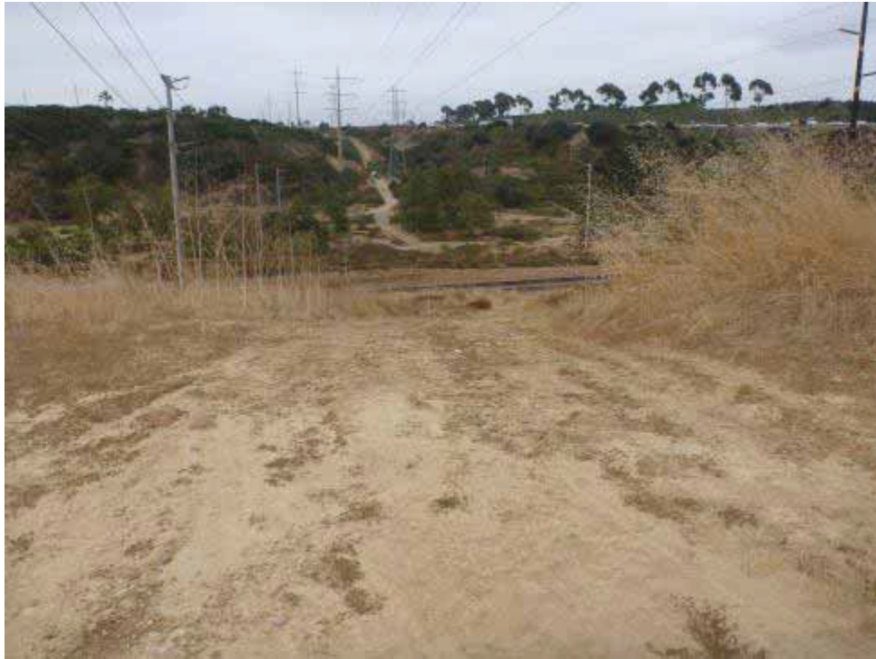
Photo 13. South-facing view of spur road to Z479045 off dirt access road off of Nobel Drive.
