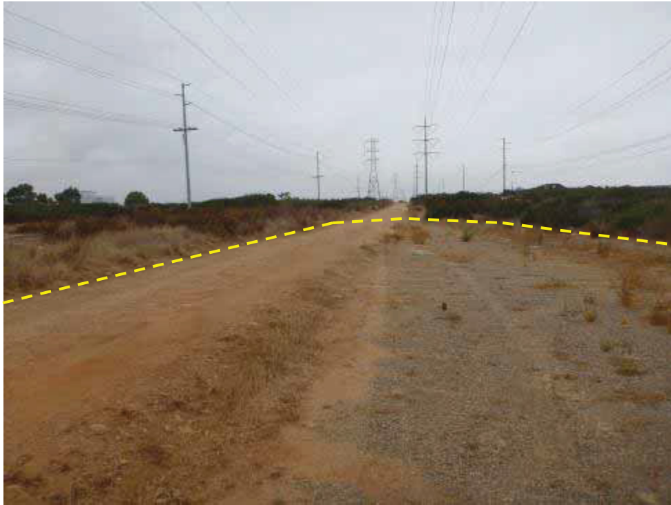
Photo 15. North-facing view of dirt access road off Nobel Drive to Z479046 and portion of work area.
