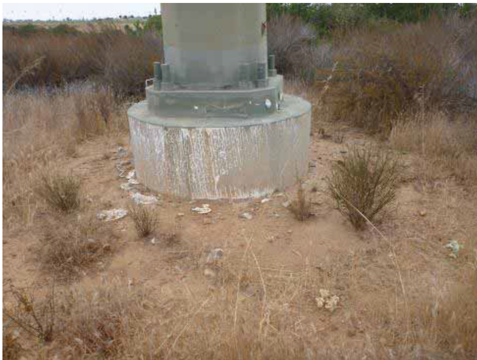
Photo 14. East-facing view of Z479046.
