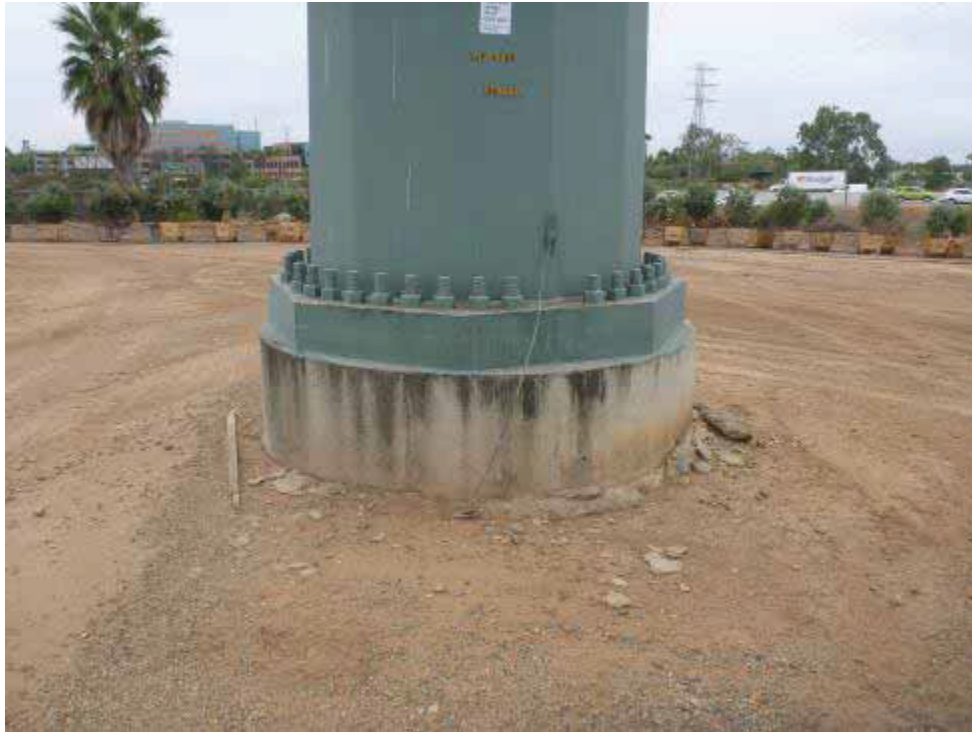
Photo 1. North-facing view of Z479040.
