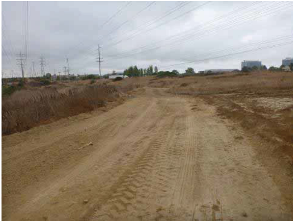
Photo 32. South-facing view of dirt access road off of Eastgate Mall Road leading to Z479053.
