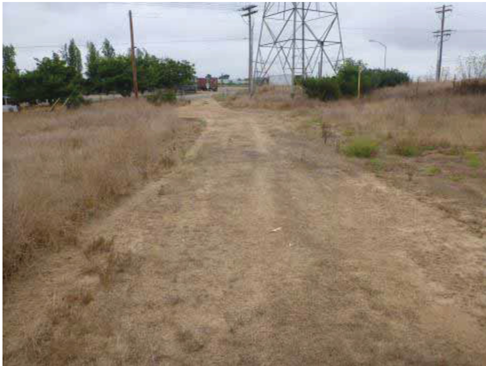
Photo 30. North-facing view of dirt access road off of Eastgate Mall Road leading to Z479052.
