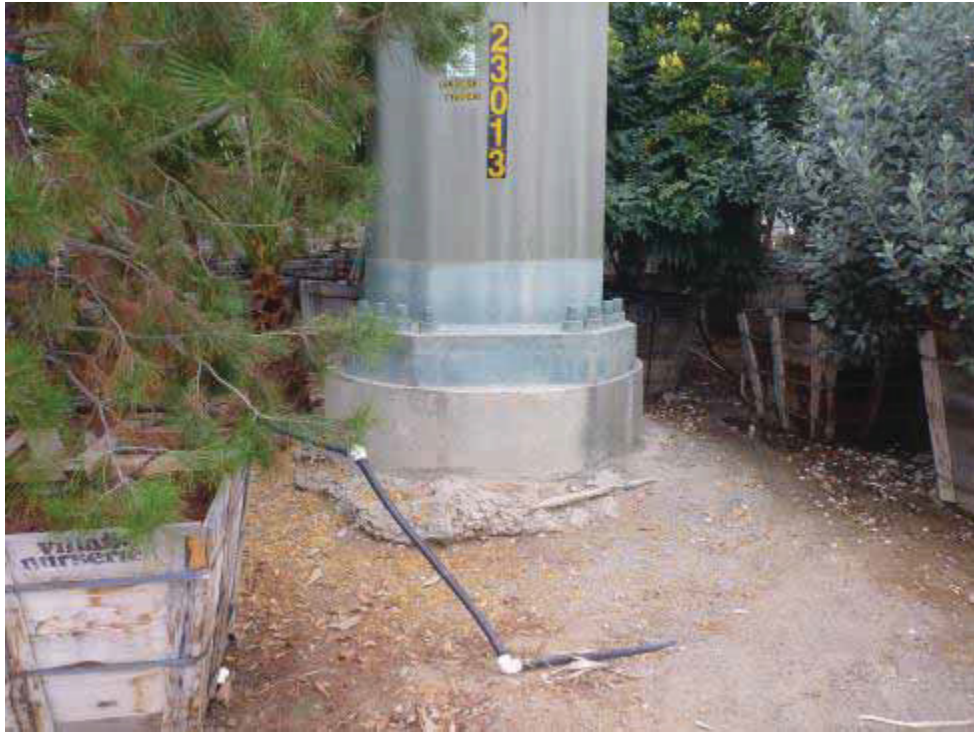
Photo 3. North-facing view of Z479041.
