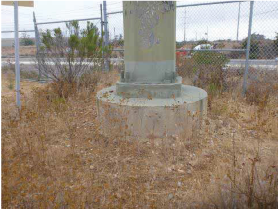
Photo 21. North-facing view of Z479049.
