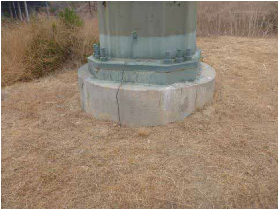
Photo 9. North-facing view of Z479044.
