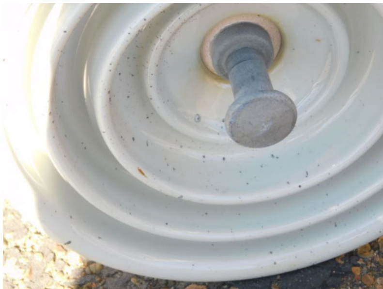
Figure 18: Insulator string that was attached to incident Jumper Cable. The grey spots on the ceramic “skirt” are the arcing residue.
