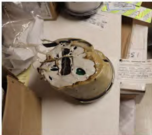
Figure 24: Melted SmartMeter from the Dixie Fire
