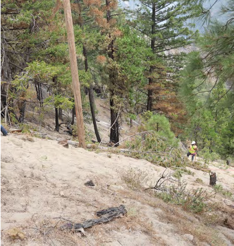
Figure 11: Base of Pole 100403909 showing fallen Subject Tree
