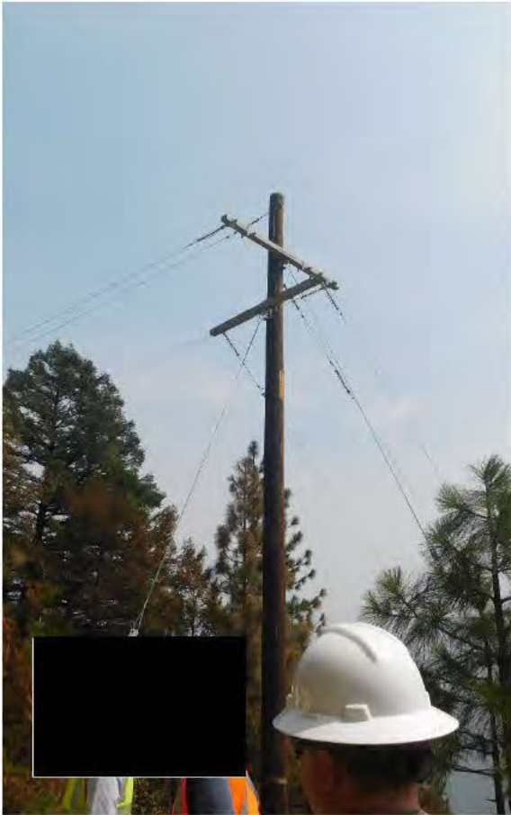
Figure 7: Pole 100403908. The fuse cutout and jumpers connecting the spans were removed by CAL FIRE.
