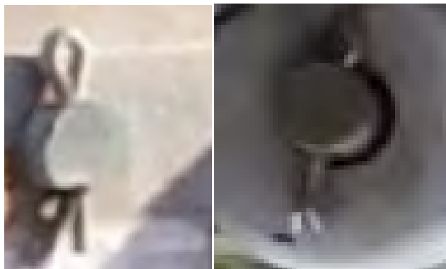
Figure 41: Examples of PG&E fully inserted cotter keys 186
