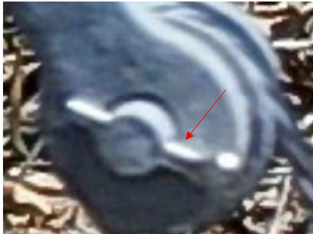
Figure 42: Partially seated cotter key at Pole 009/131 on May 26, 2022 187 (red arrow shows unseated section)
