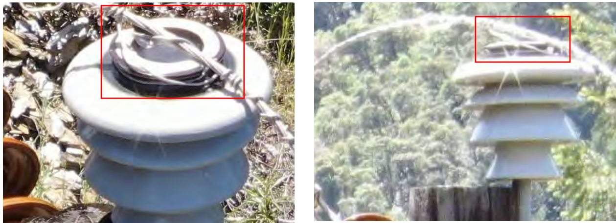
Figure 35: PG&E photos of loose tie wire, Pole 014/186(A), May 26, 2022 130 (SED outlined in red the loose tie wires)
