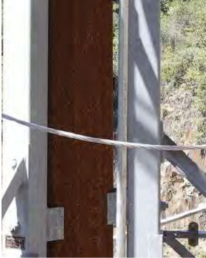
Figure 27: Switch 47 upper control rod and lower jumper on May 16, 2022, showing no visible damage. 97
