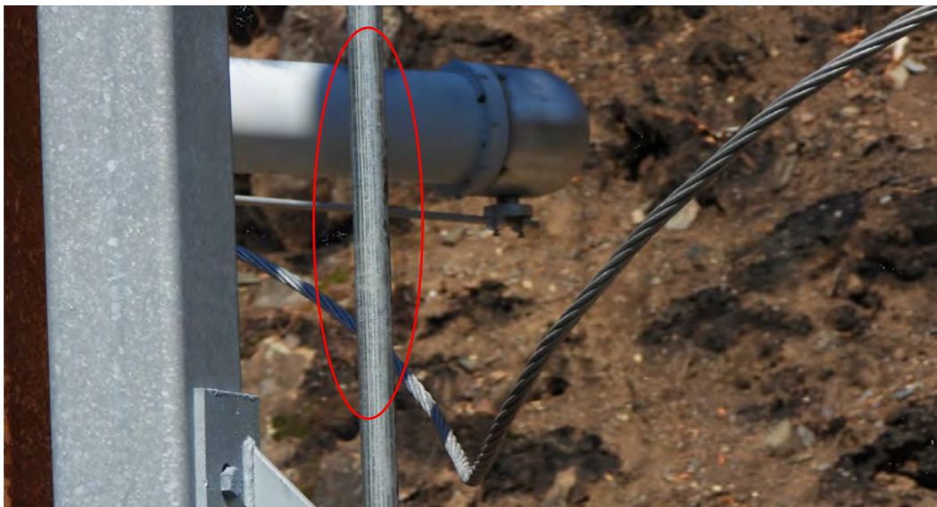
Figure 10: Jumper wire kinked on lowest phase of Switch 47. Red circle indicates damaged section of control rod. 40
