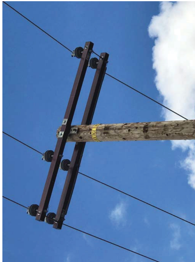
Covered Conductor on Tangent Pole
