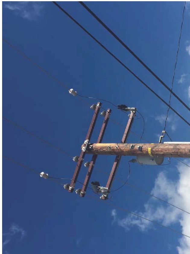
Covered Conductor with Transformer
