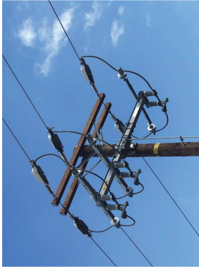
Covered Conductor with Pole Switch
