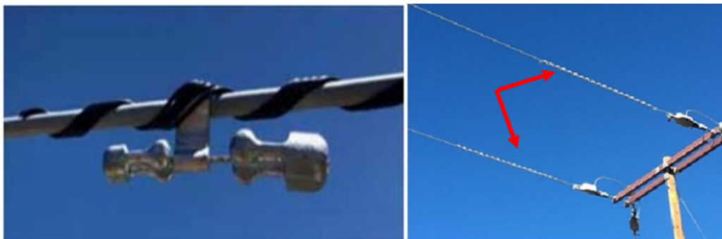
Figure V-16 Types of Vibration Dampers: Stockbridge Damper (left) and Spiral Damper (right)
