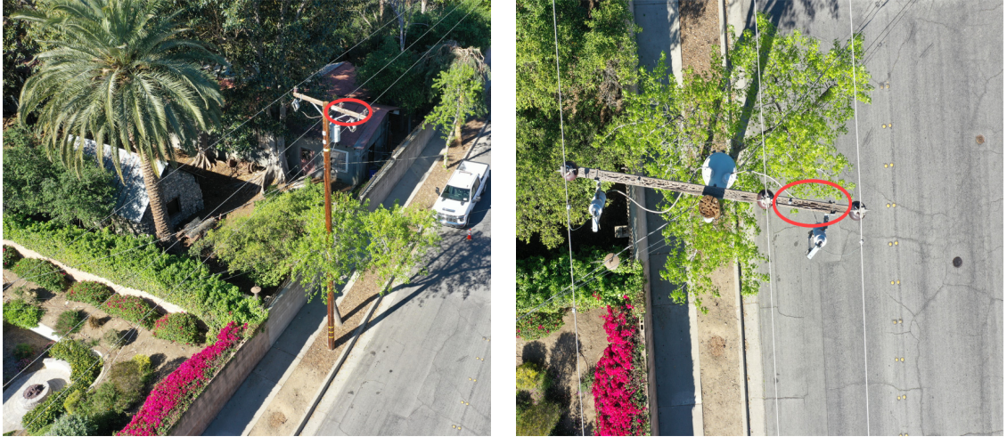
Figure VII-29 Distribution Deteriorated Crossarm Distant (left) and At Close Range (right)
