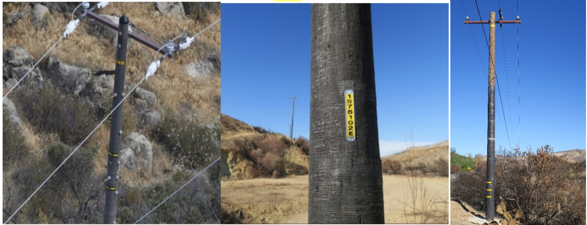
Figure V-13 Composite Pole (left), FRP Close-up (center), and FRP Full Length (right)
