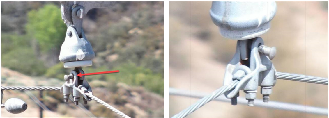
Figure VII-30 Transmission Missing Cotter Key Distant (left) and At Close Range (right)
