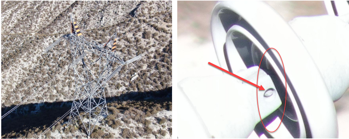
Figure VII-31 Transmission Missing Cotter Key Distant (left) and At Close Range (right)
