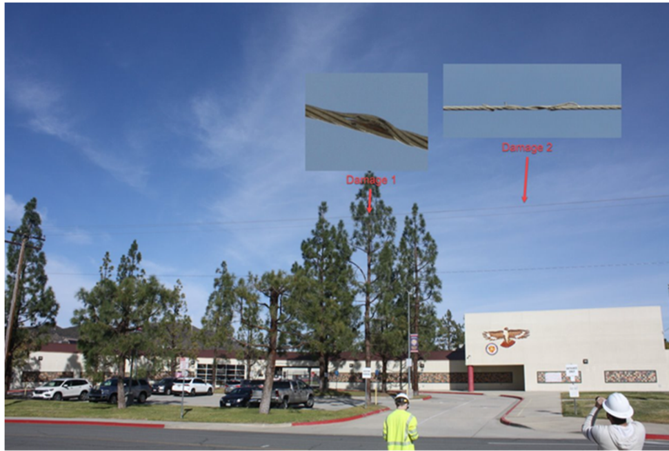
Figure V-23 An Example Where EFD Detected Conductor Damage Due to Gun Shot(s)
