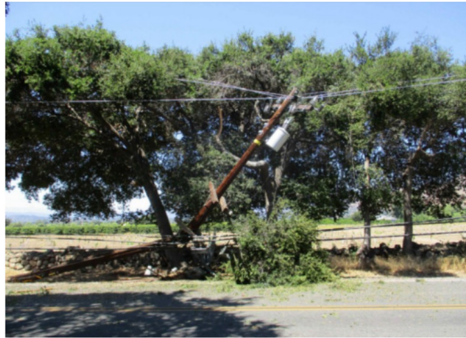
Figure V-12 Car-hit-pole with Covered Conductor – No Fault Occurred Ojai, California – July 24, 2020
