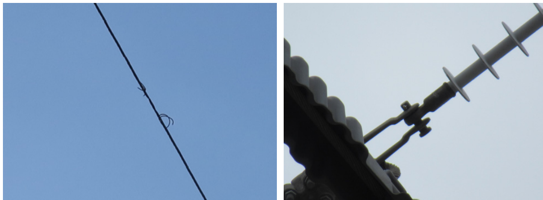
Figure VII-28 Damaged Primary Conductor (left) and Missing Cotter Key (right) on 12kV Circuits
