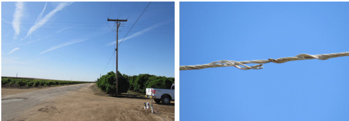
Figure VII-27 Damaged Primary Conductor on a 12kV Circuit Distant (left) and At Close Range (right)
