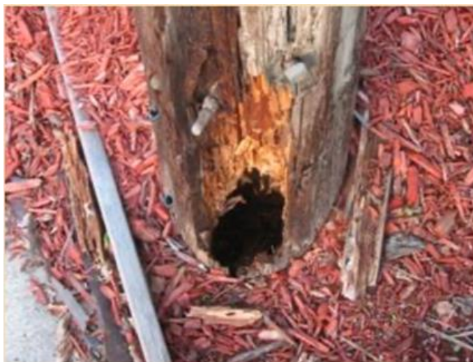
FIGURE 2-7 DETERIORATED POLE
