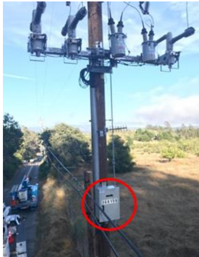
FIGURE 2-11 SCADA RECLOSER INSTALLED ON POLE
