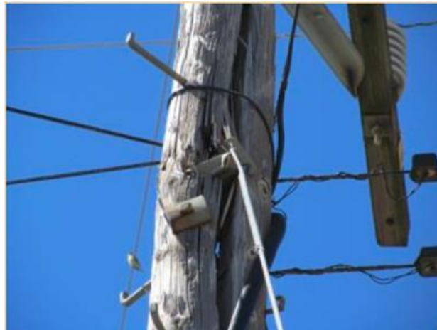
FIGURE 2-8 POLE SPLIT AT COMMUNICATION LEVEL
