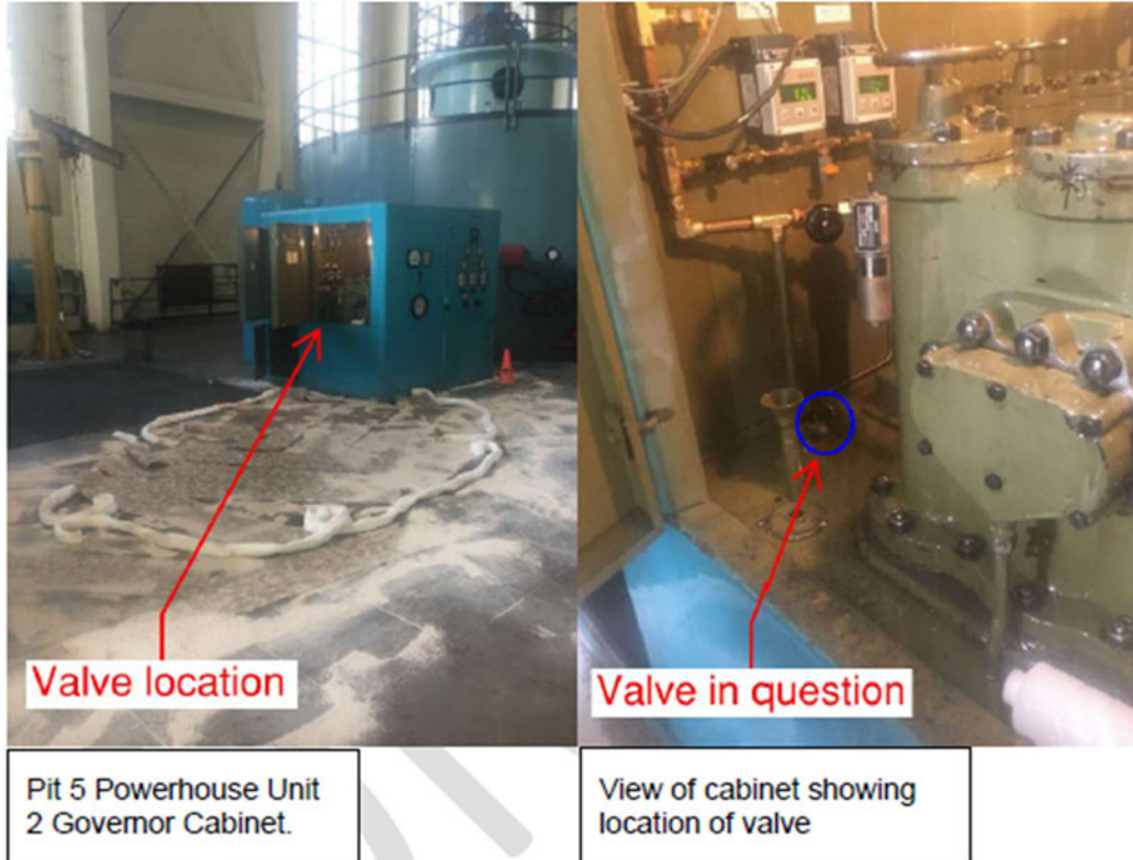
Figure 3-4 Pit 5, Unit 2 – Min-Ball Valve Location 198
