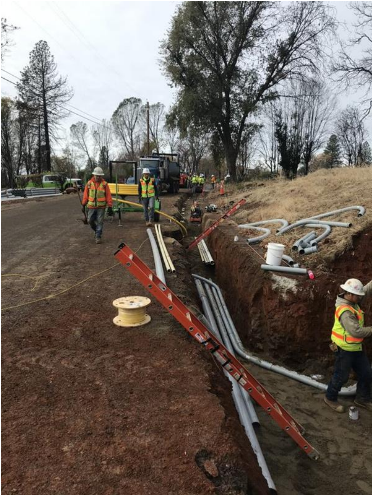
FIGURE 4.3-4 UNDERGROUNDING CONSTRUCTION IN PROGRESS
