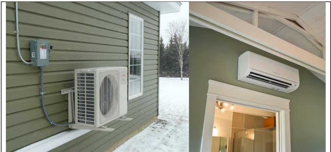
Figure 47: An example of a ductless mini-split heat pump outdoor compressor 100 mounted to stay above the snow and a wall-mounted indoor fan coil 101 .
