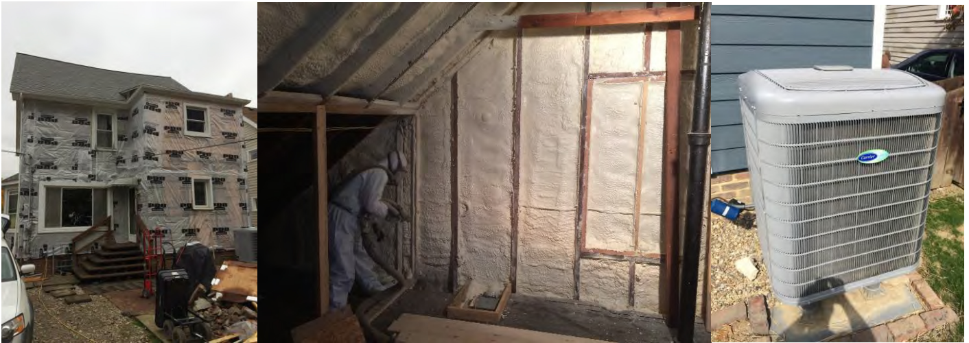
Figure 32: Jon and Kelly's retrofit snap shots, new siding (left), adding insulation, and their Carrier Greenspeed heat pump. 79
