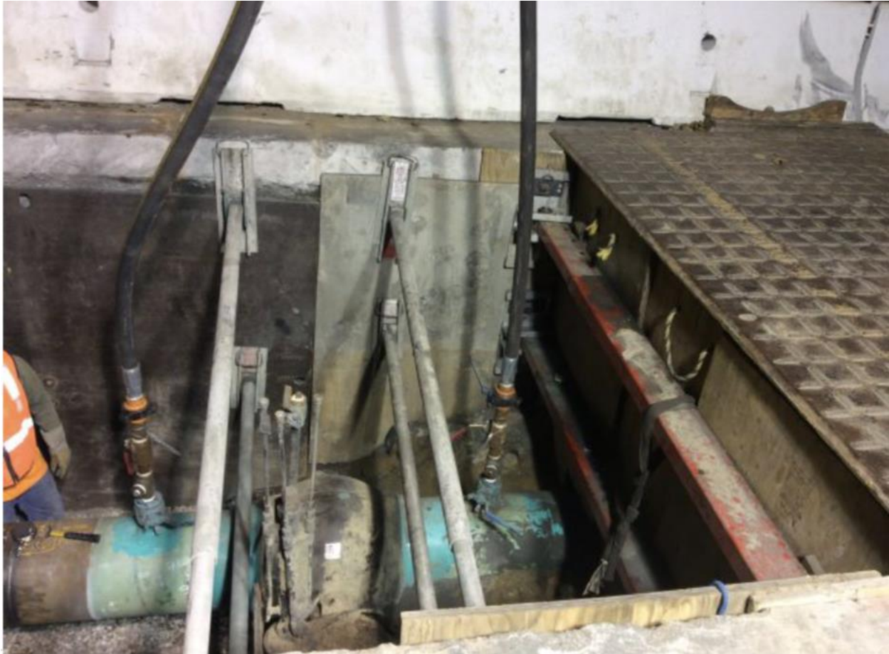
Figure 8: Hoses and Connections for Seasoning of New Pipeline
