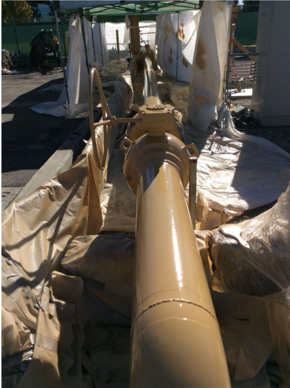
Figure 3: Newly Coated Pipeline
