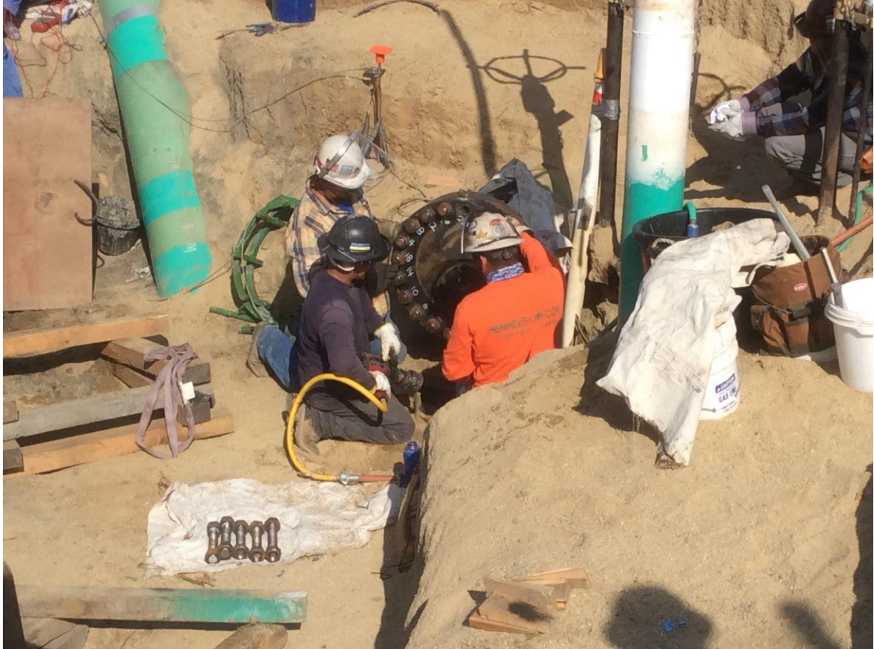
Figure 3: Bolting up Blind Flange
