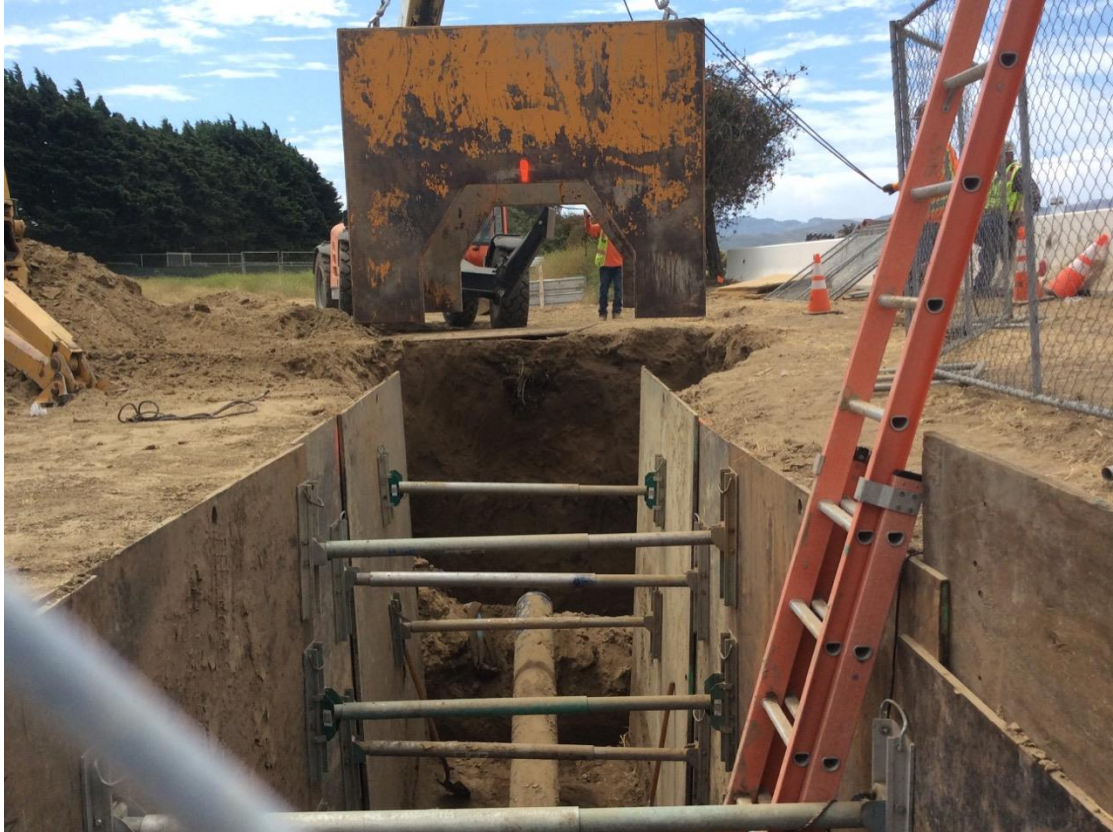
Figure 3: Setting Shoring Box
