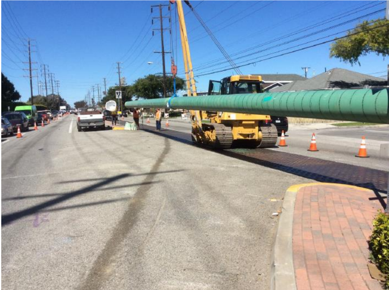
Figure 3: Positioning New Pipe Along 190 th Street
