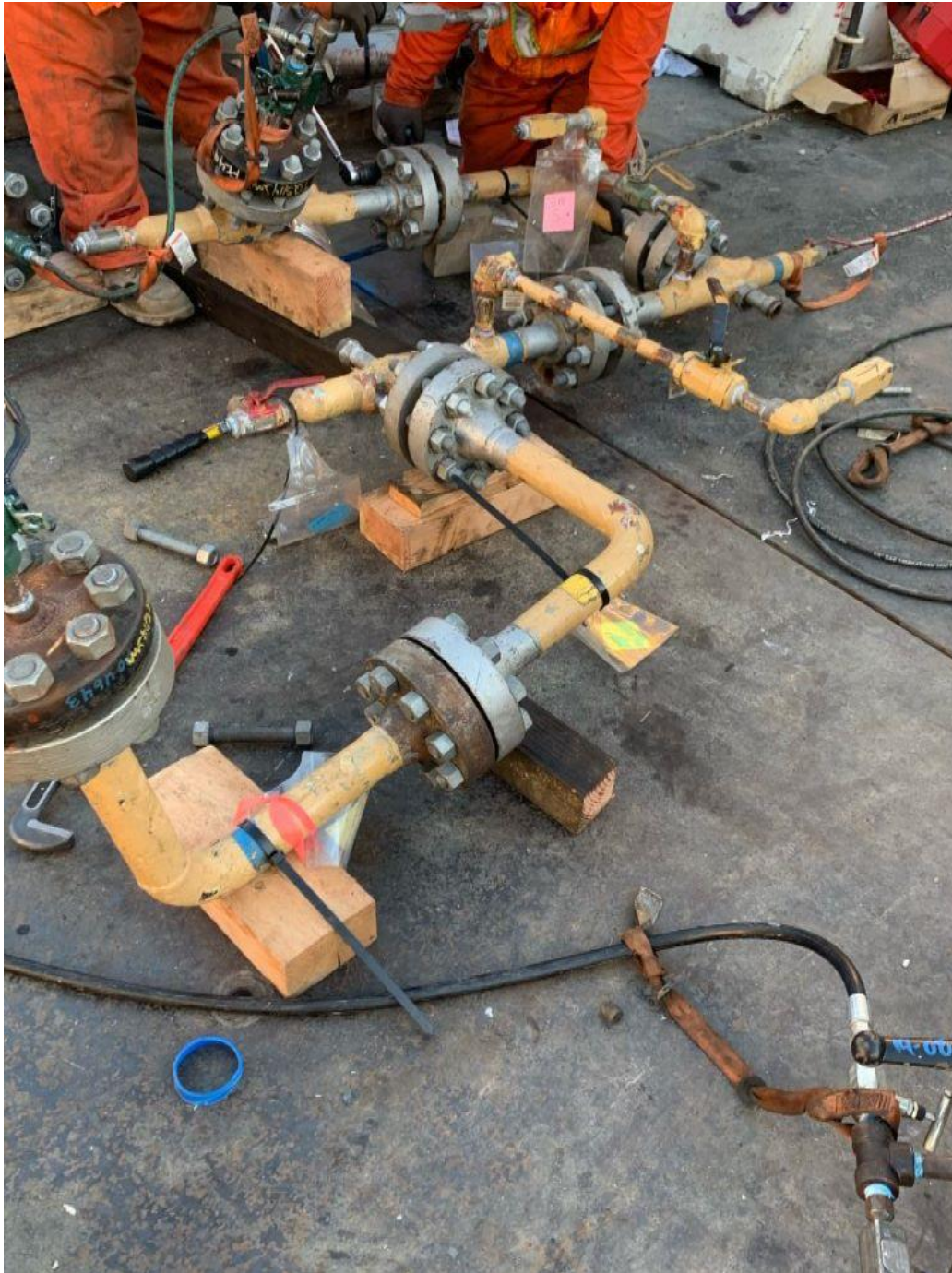
Figure 3: Flanges Being Prepared Prior to Hydrotest
