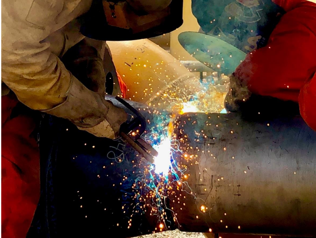
Figure 1: Welding of Pipe and Reducer Flange
