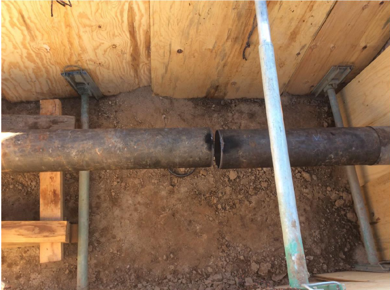
Figure 4: Cut of Existing Pipeline for Replacement
