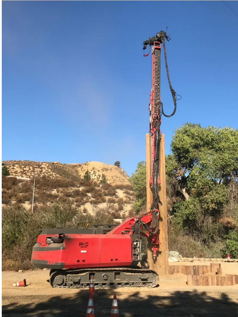
Figure 4: Driving Sheet Piling
