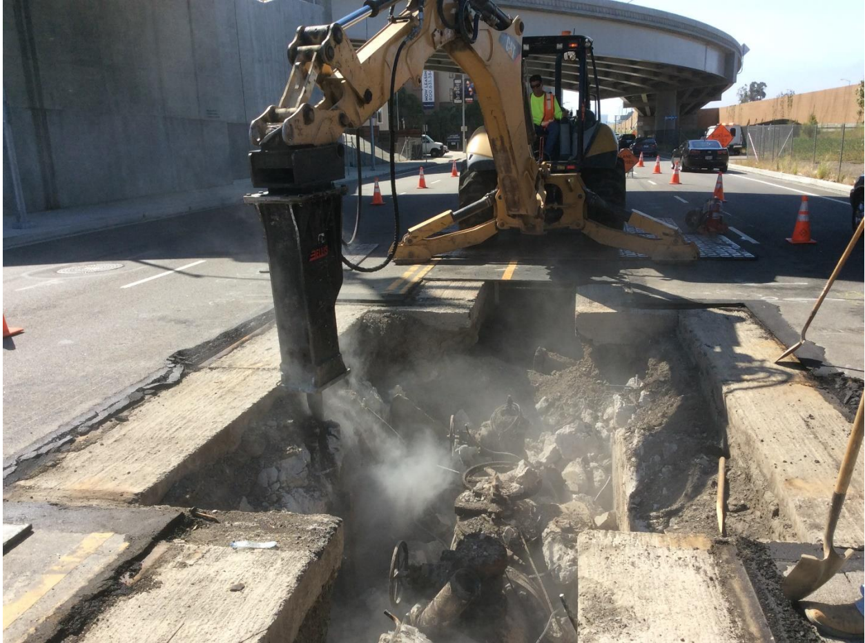
Figure 9: Demolition of a Concrete Vault
