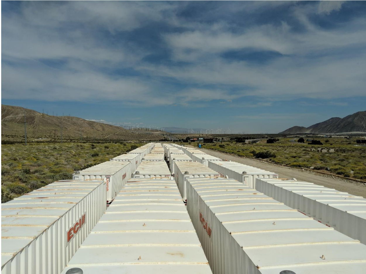
Figure 6: Water Storage Tanks at Test Break
