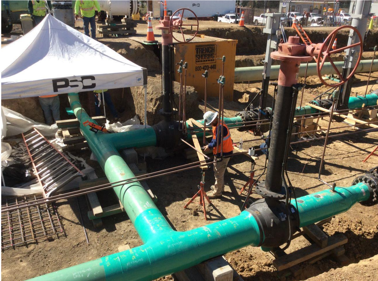
Figure 2: Applying Cathodic Protection Wrap
