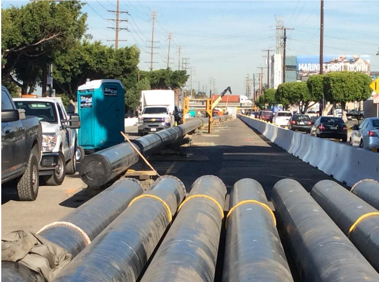
Figure 5: Preparing for Horizontal Directional Drill Pullback
