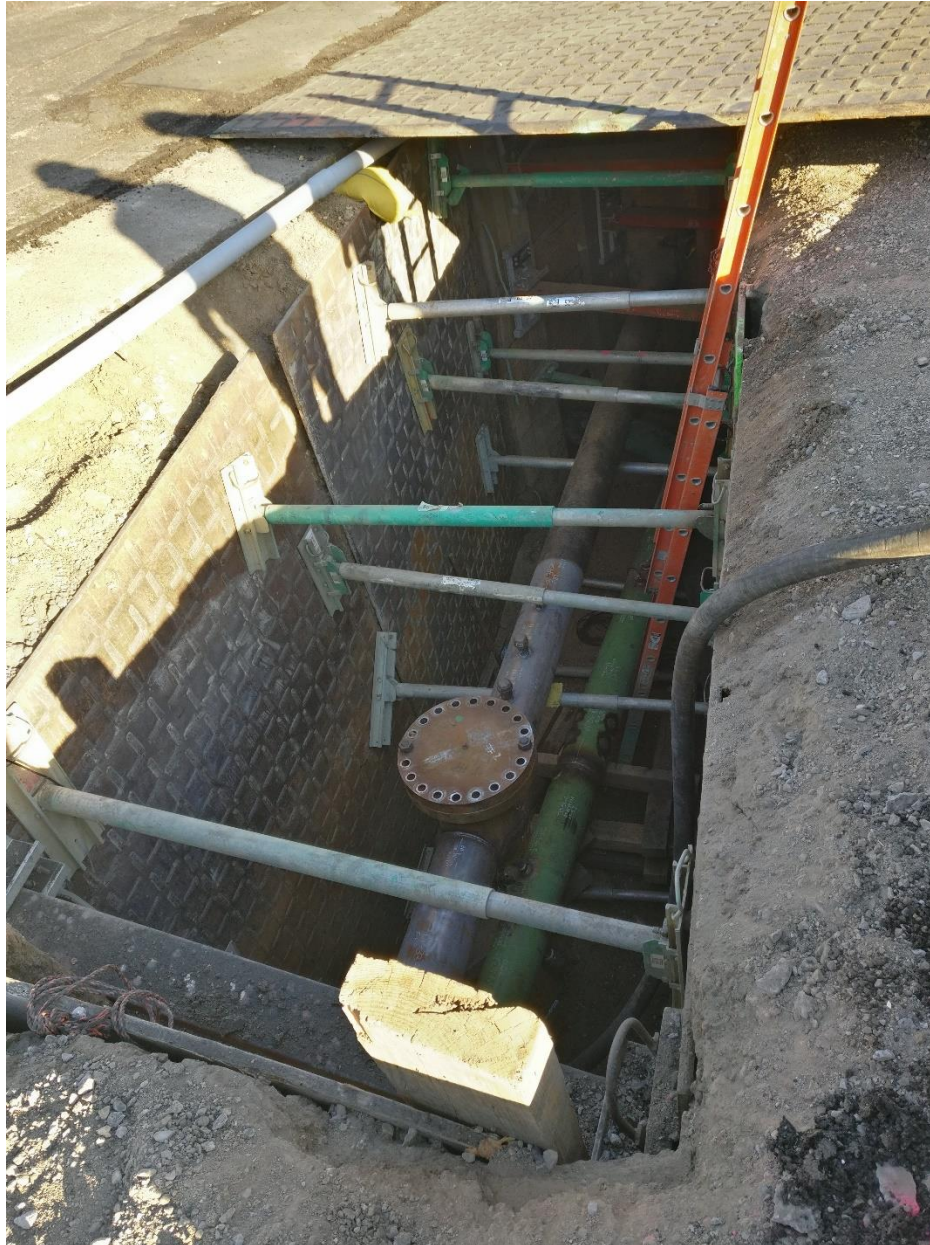
Figure 4: PCF Connecting the Old and New Pipeline
