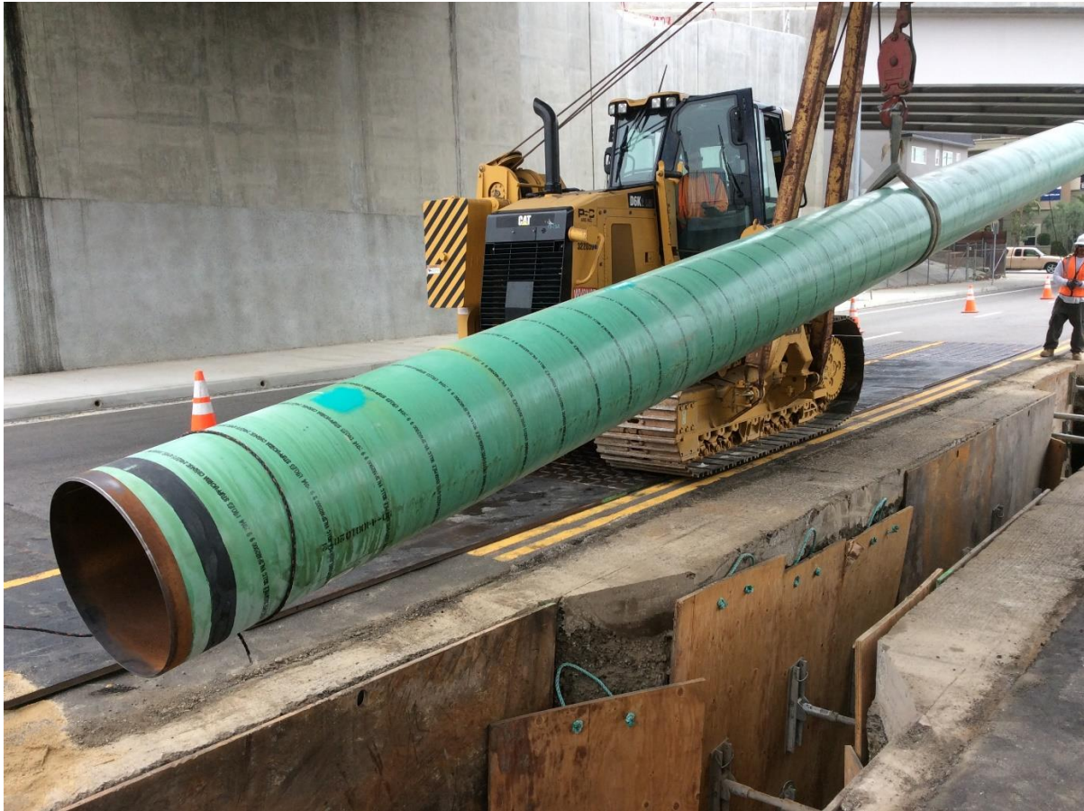
Figure 10: Lowering in of New Pipe
