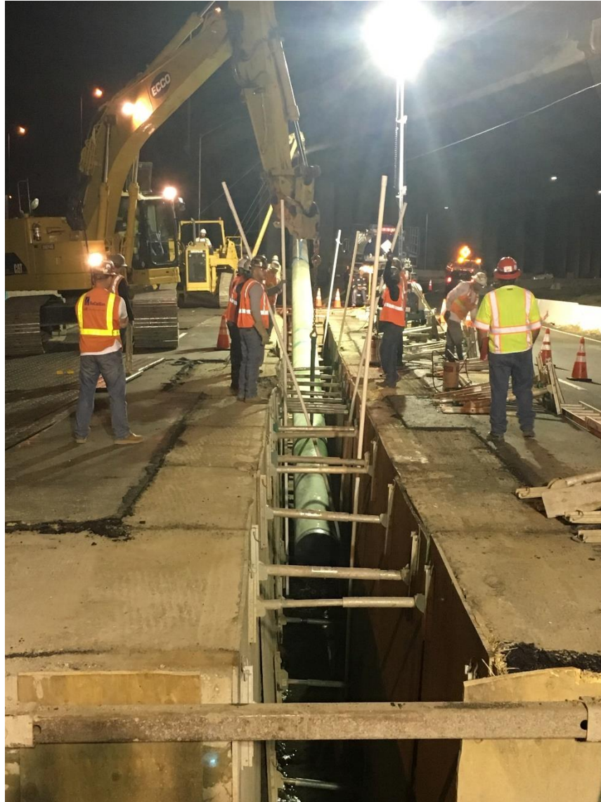
Figure 12: Lowering in New Pipe
