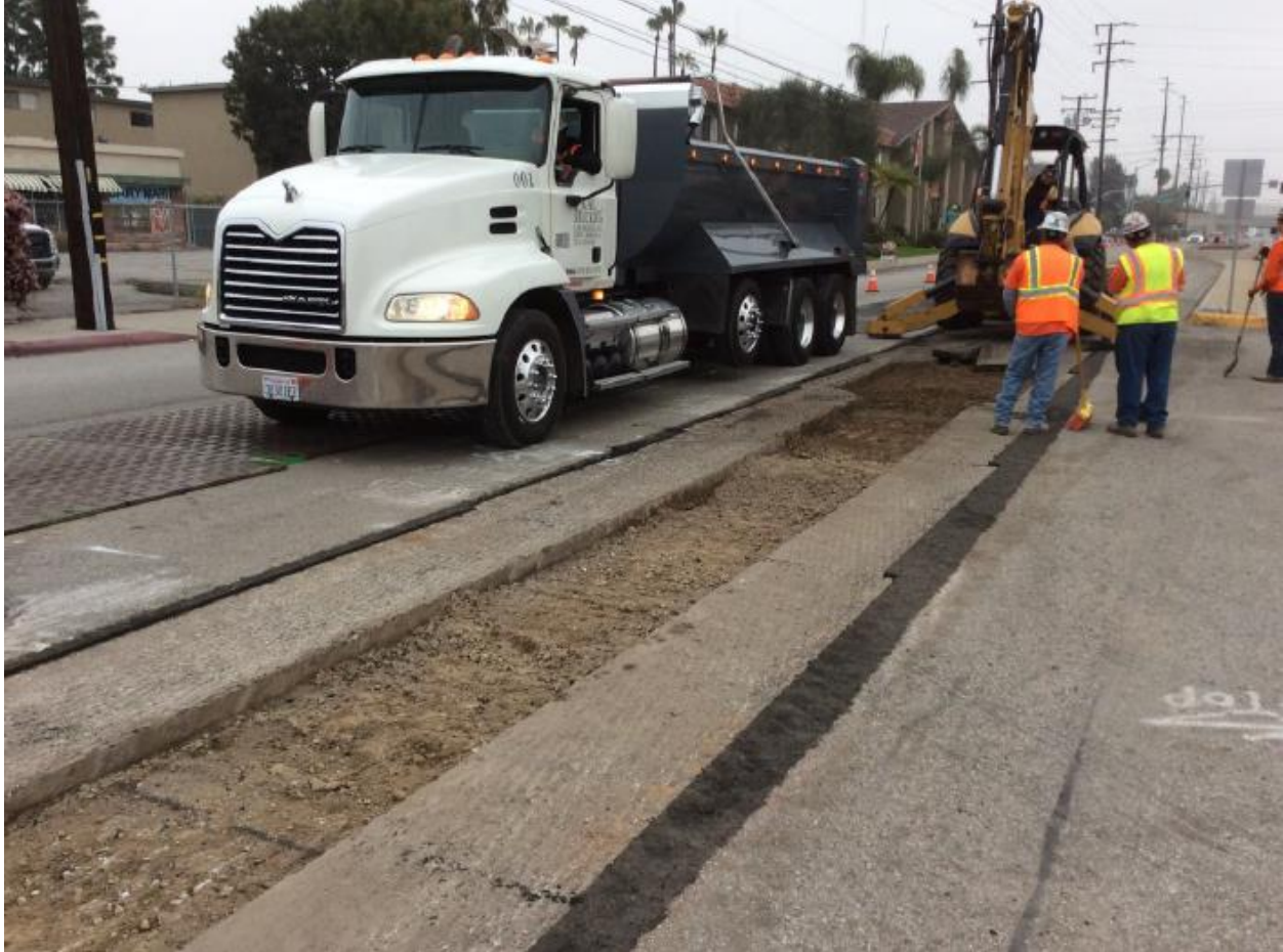
Figure 5: Trenching Along 190 th Street Near Hawthorne Boulevard
