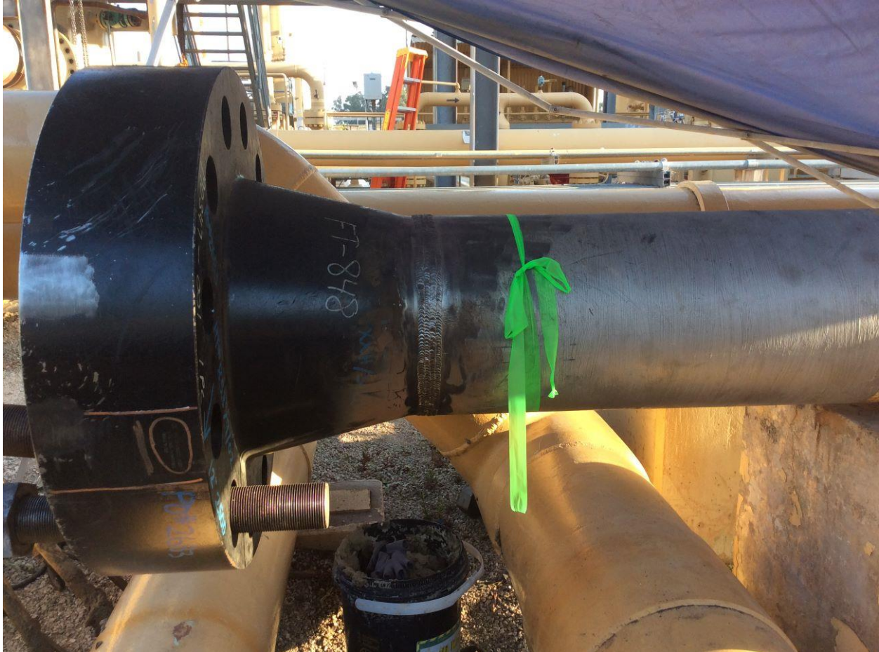
Figure 2: Completed Weld of Pipe and Reducer Flange
