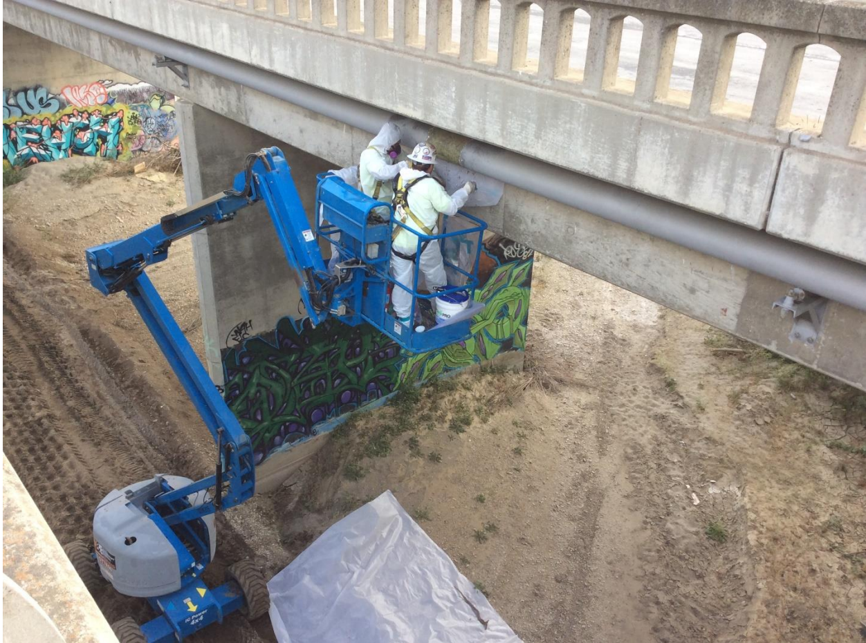
Figure 5: Abatement for Pipe Removal of Santa Ynez River Bridge.
