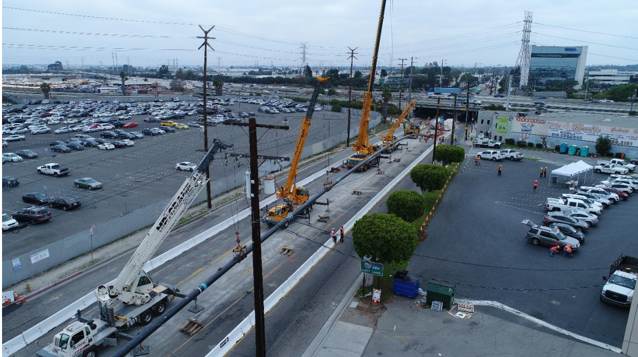
Figure 4: Cranes Positioning Pipe for Horizontal Directional Drill Pullback
