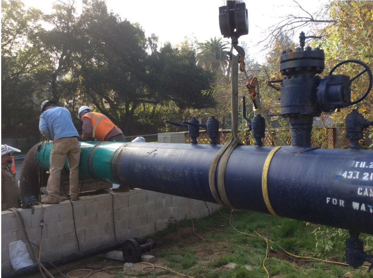
Figure 3: Installing Test Head
