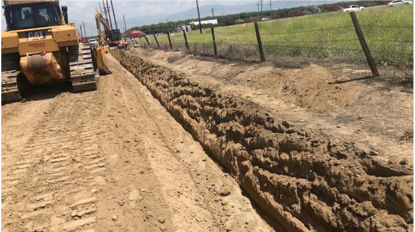
Figure 4: Excavation for Section 2 Reroute
