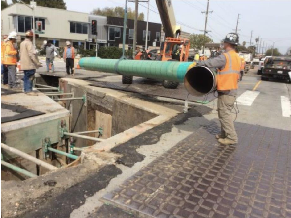
Figure 6: Installing Offset at the Intersection of Figueroa Street and Victoria Street
