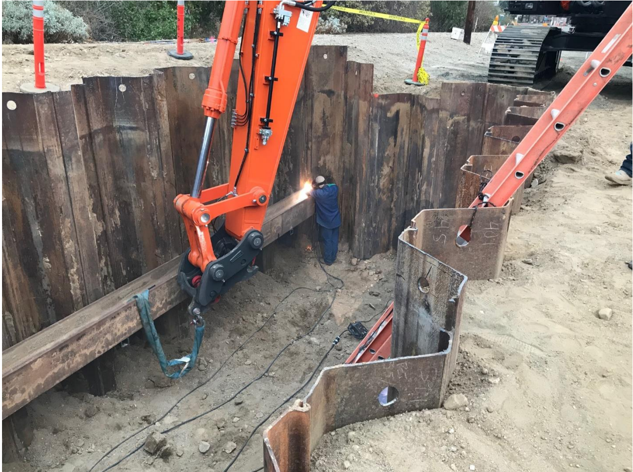
Figure 5: Welding Support Beams for Entry Bore Pit
