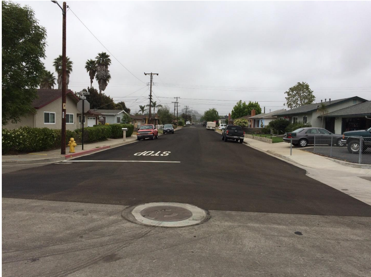
Figure 6: Site Restoration / Repaved Street
