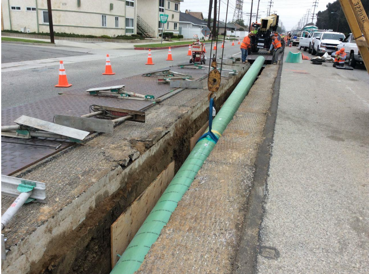
Figure 4: Installing Pipe Along 190 th Street
