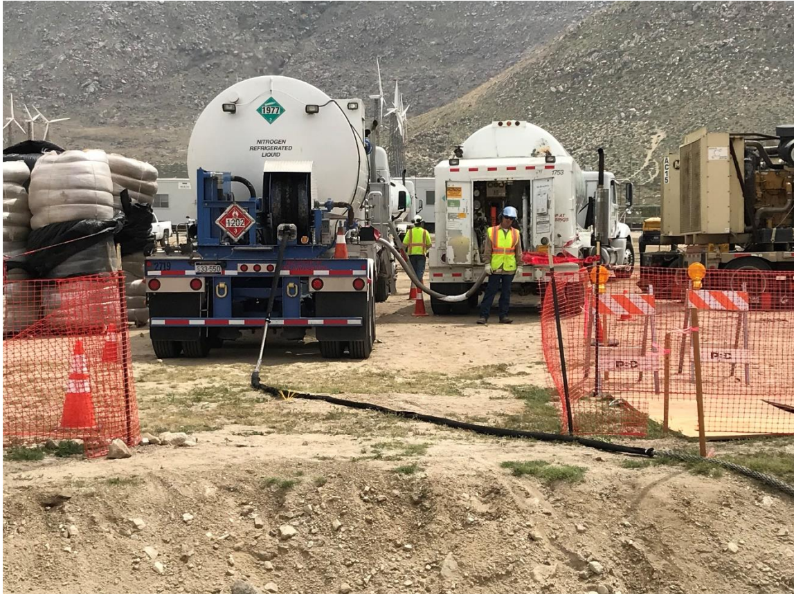
Figure 4: Liquid Nitrogen Truck and Equipment Used For Leak Detection
