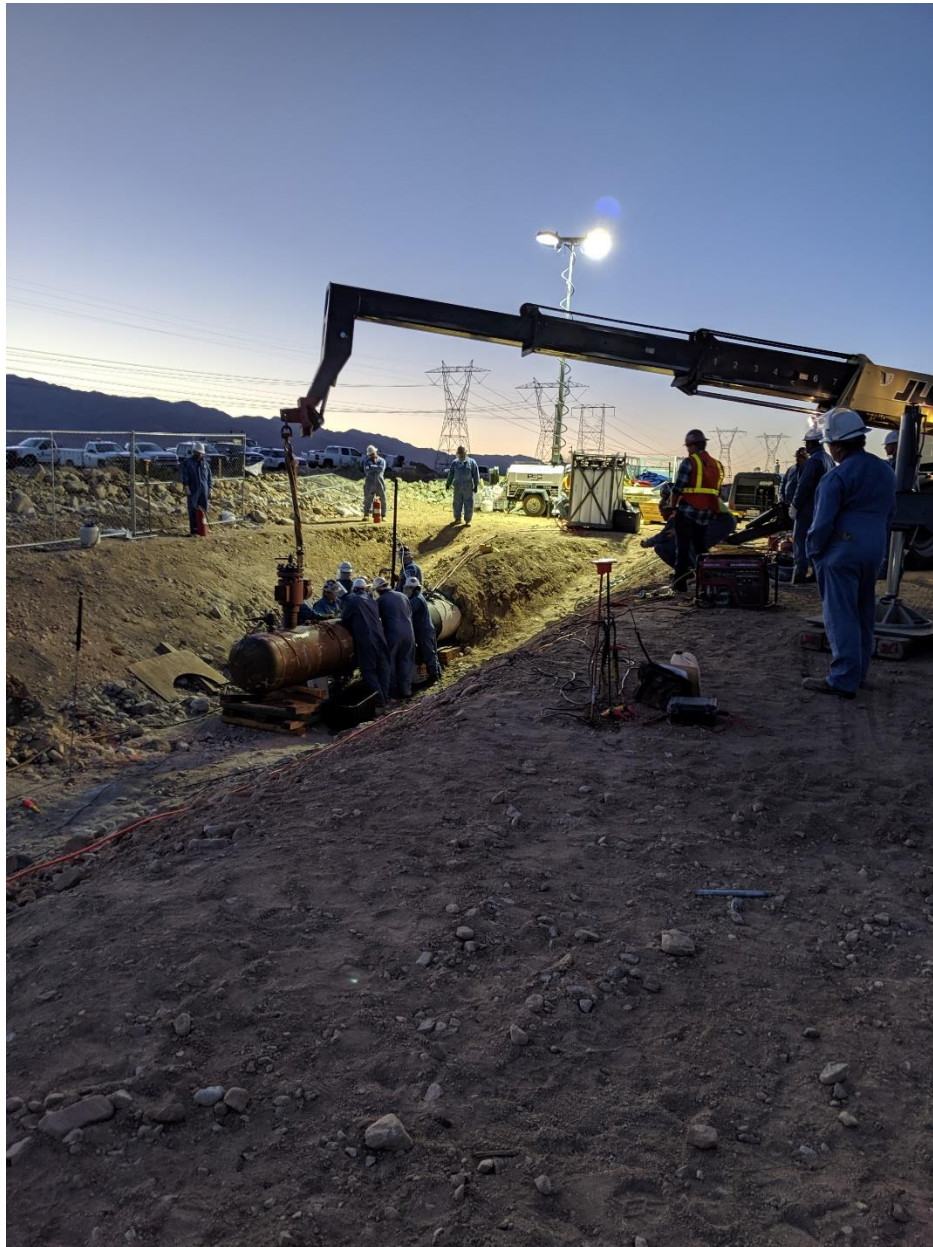
Figure 5: Pre Tie-In Activities
