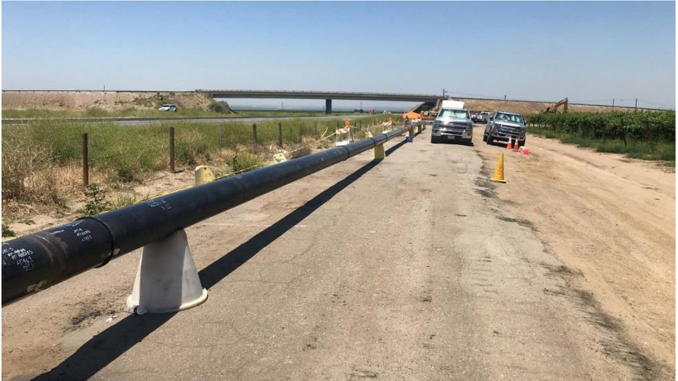
Figure 5: Pipe Prepared for HDD under Sabodan Street
