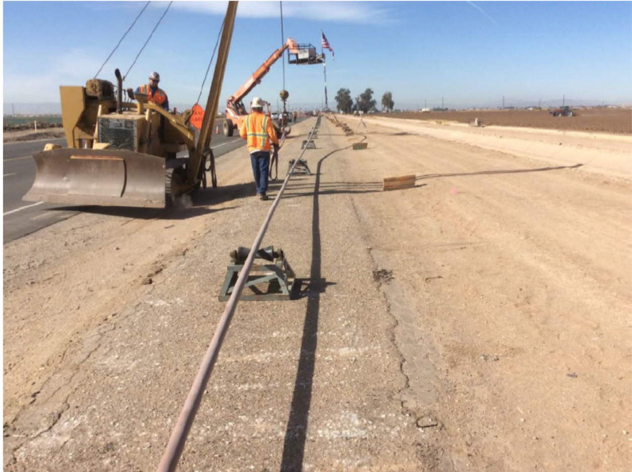
Figure 9: Stringing of New [REDACTED] Pipe for Bore Along Aten Road
