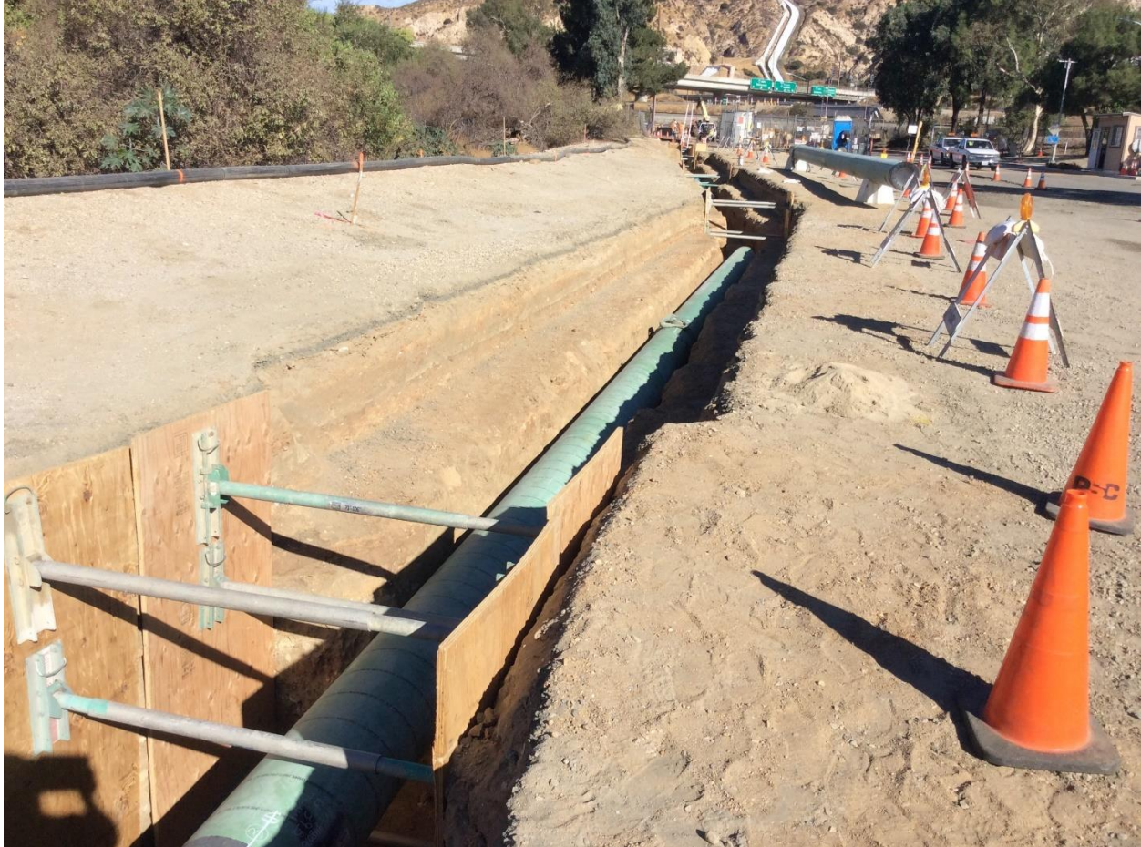
Figure 6: New Pipe Lowered into Trench
