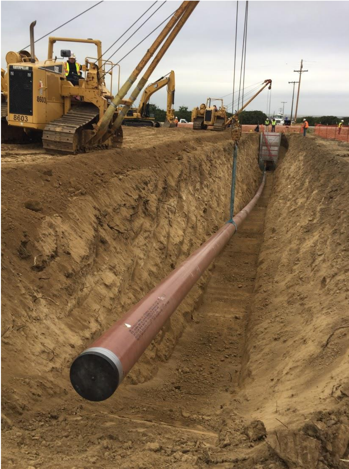
Figure 3: Lowering in Pipe at the Wheeler Ridge Access Road Crossing
