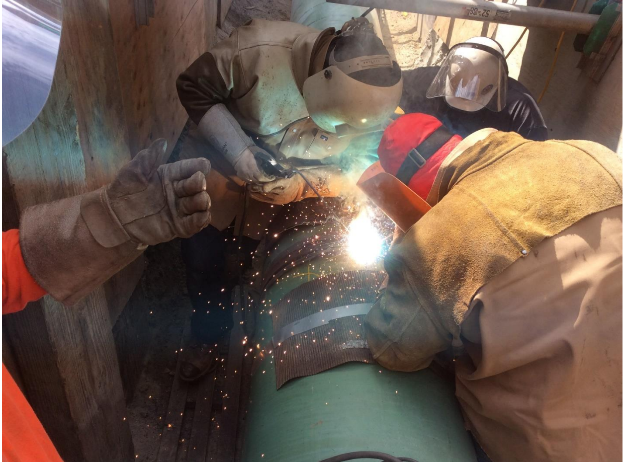
Figure 12: Construction Crew Welding
