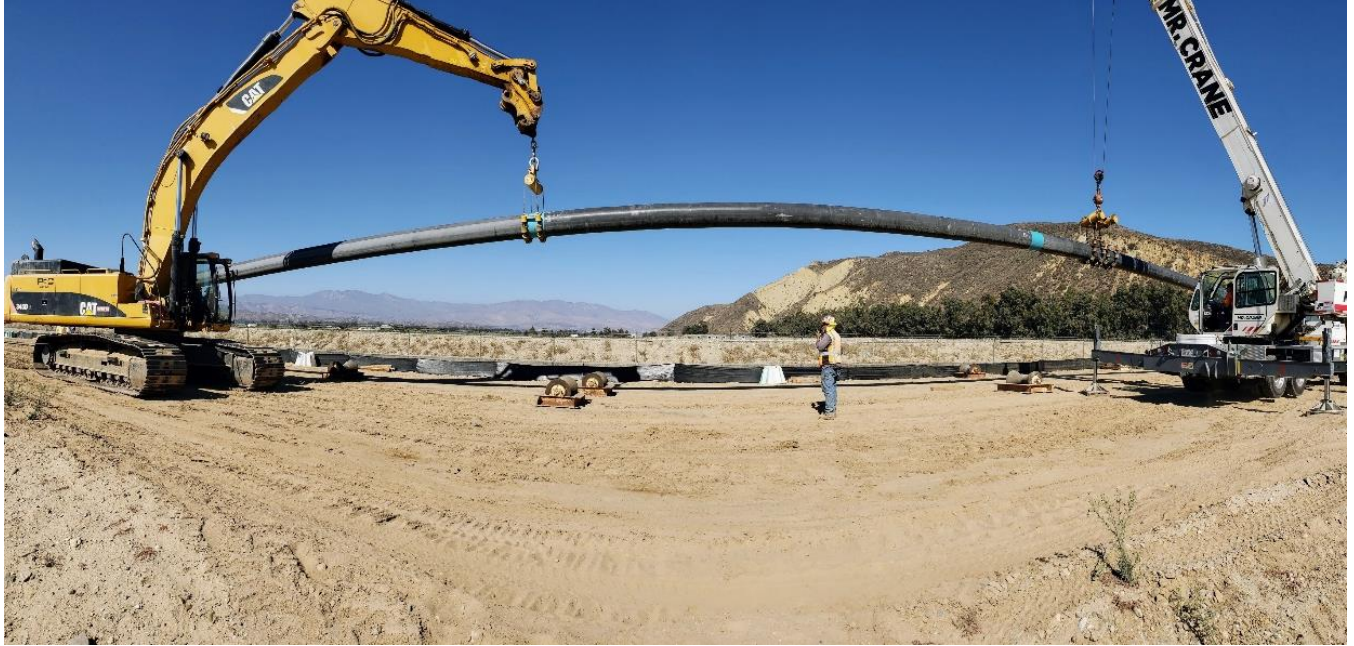
Figure 5: Horizontal Directional Drill Pullback
