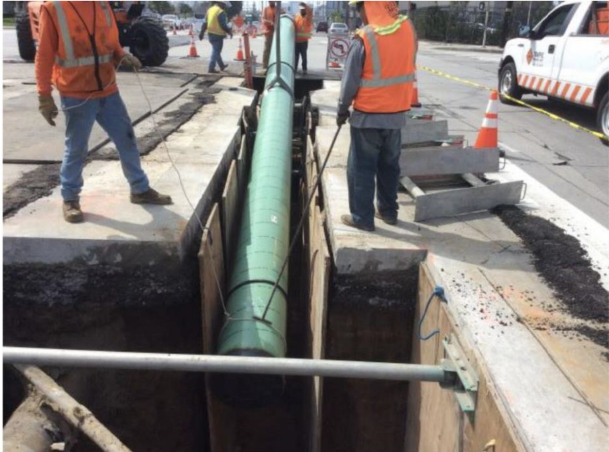
Figure 7: Lowering New [REDACTED] Pipe into Trench
