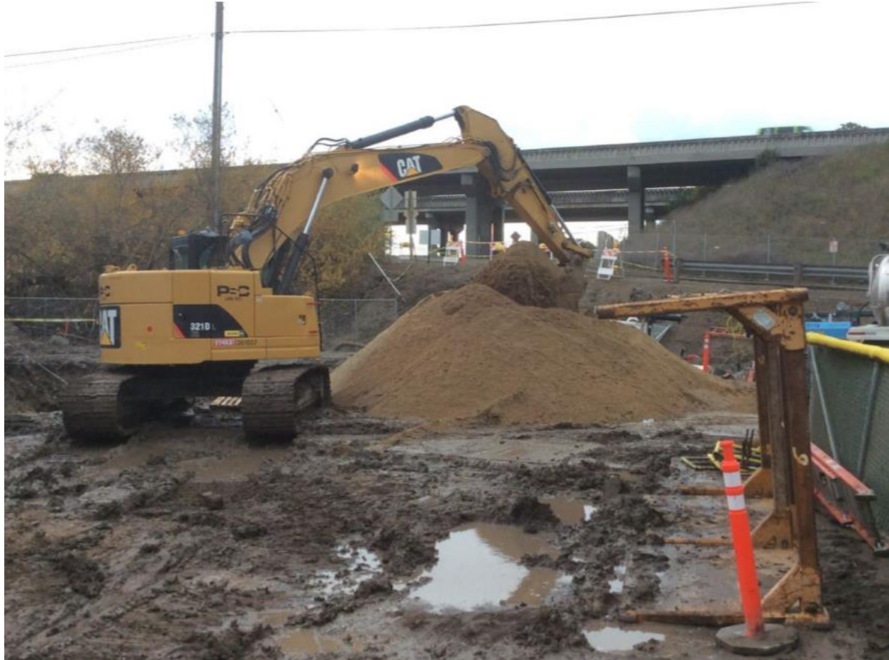
Figure 8: Excavation in Progress for James Way Horizontal Directional Drill Exit Pit
