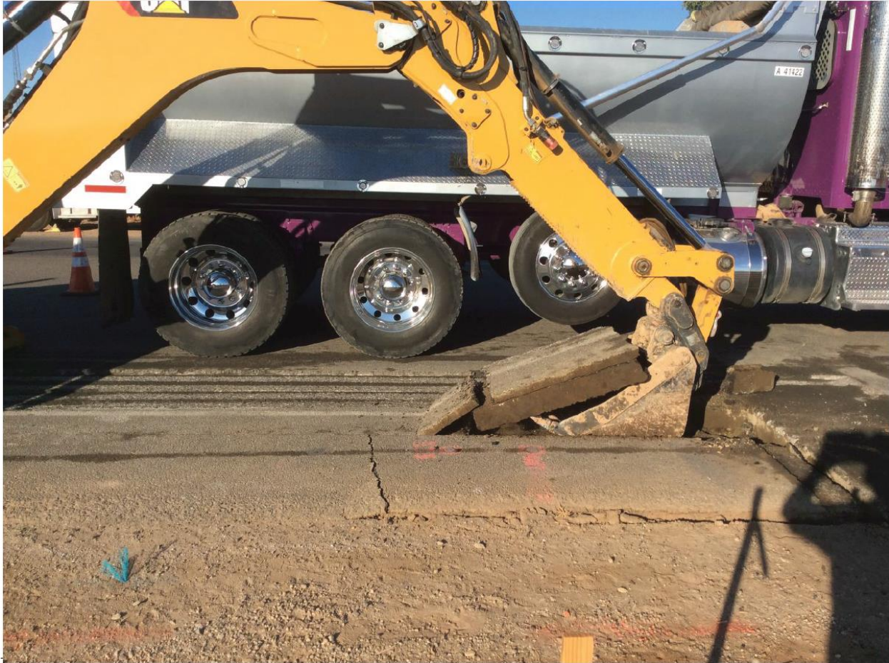
Figure 3: Excavation and Removal of Asphalt
