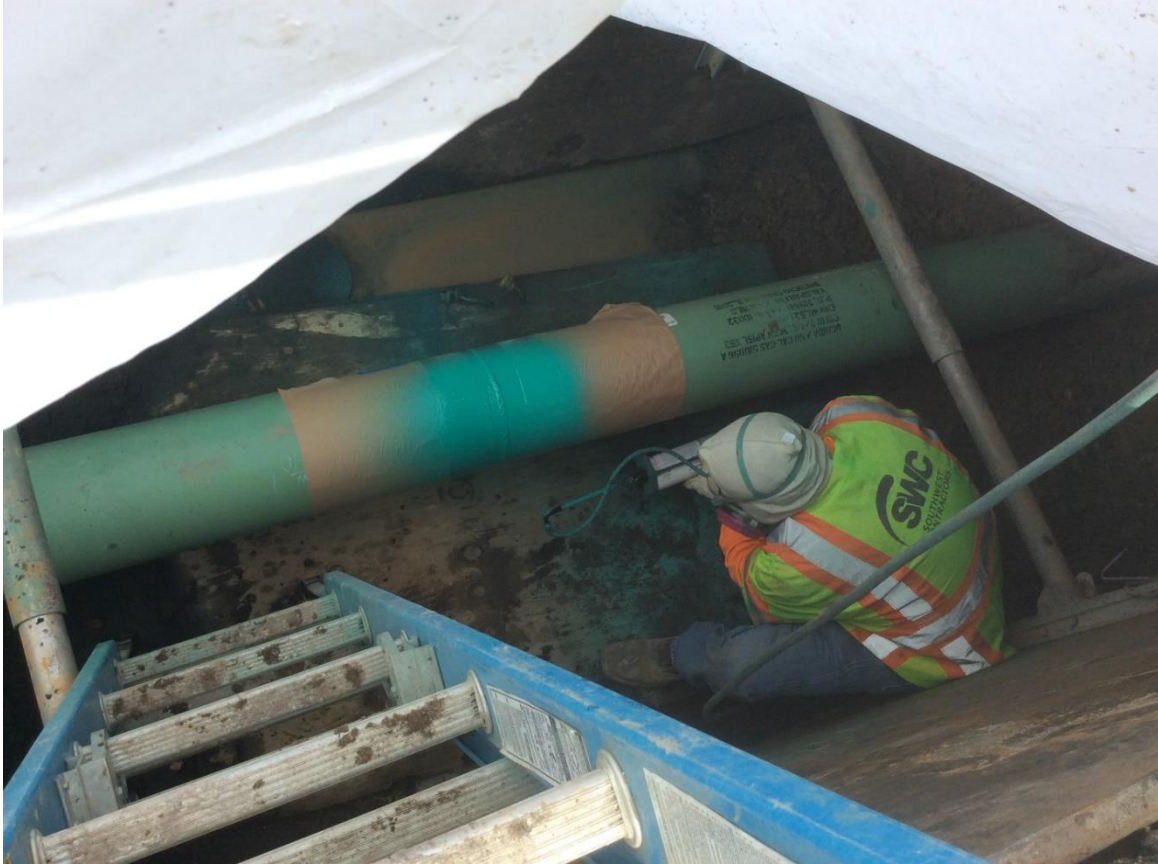
Figure 9: Applying Epoxy Coating to New Pipeline
