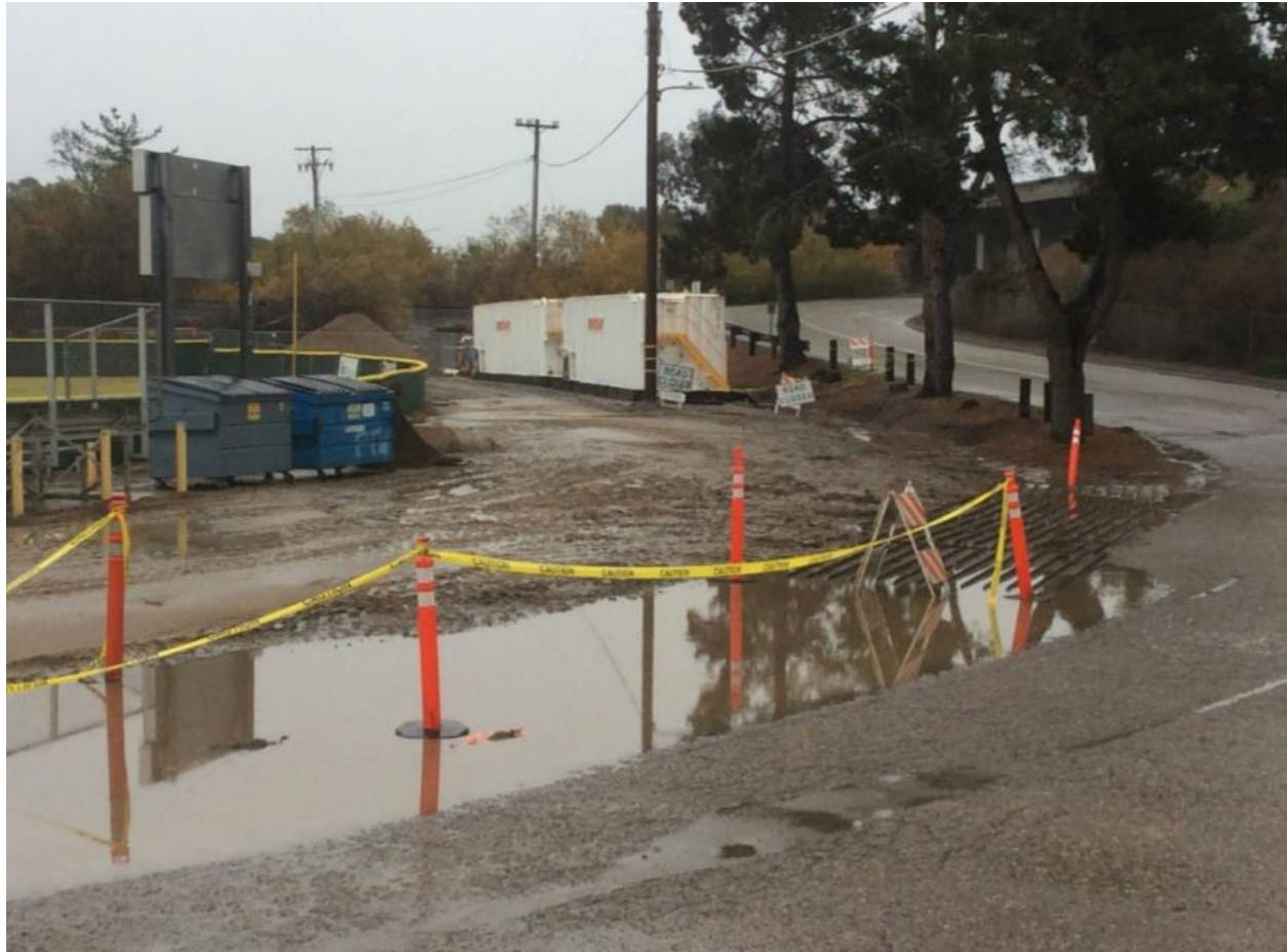
Figure 7: Access Road Leading to James Way Horizontal Directional Drill Exit Pit
