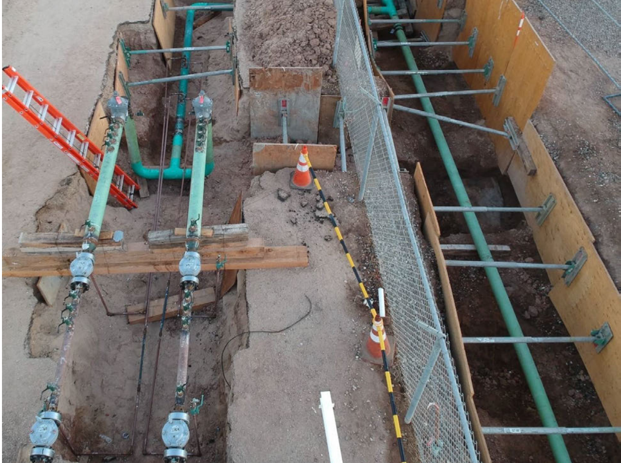
Figure 7: Aerial View of New Regulator Station
