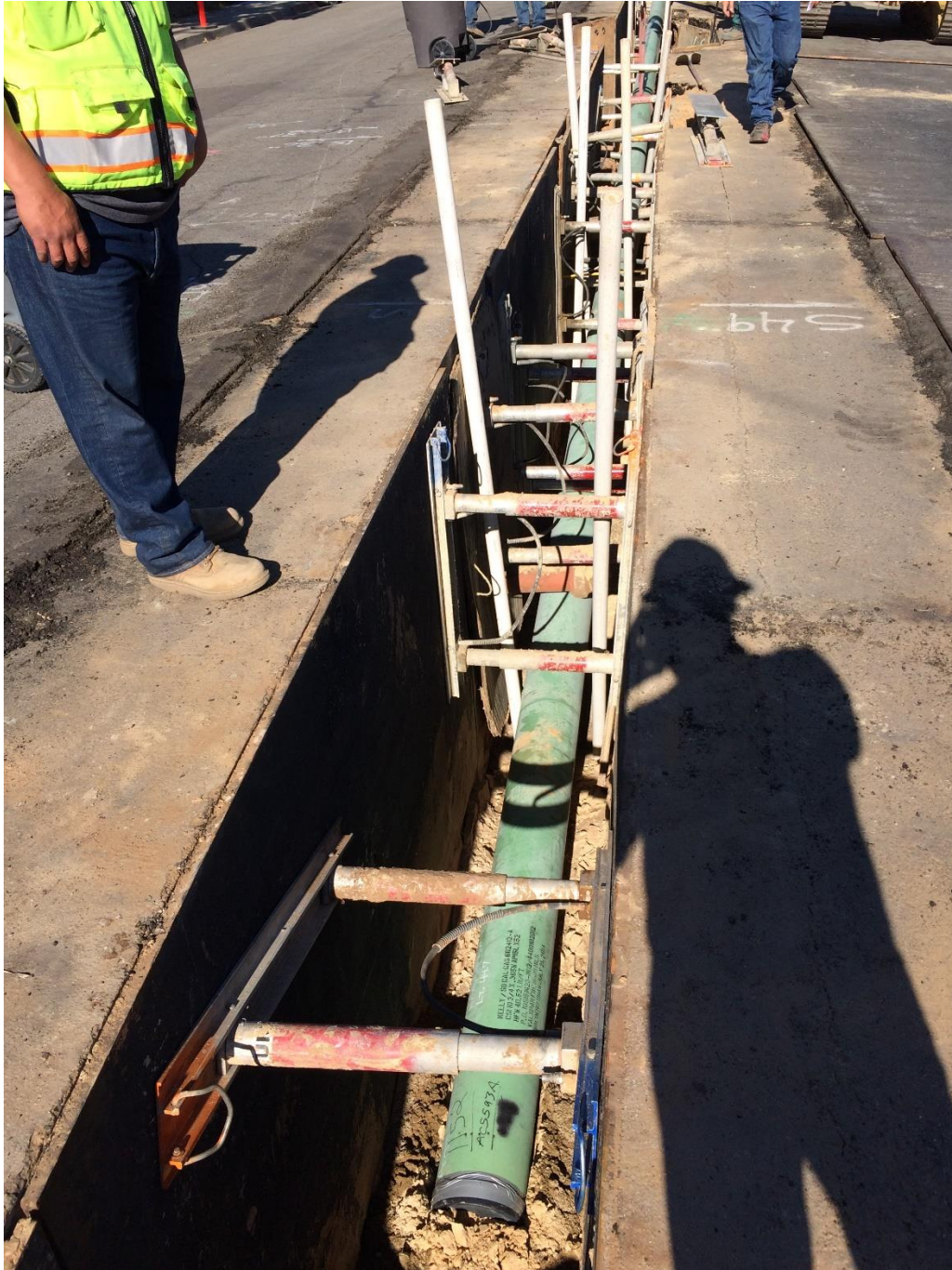
Figure 5: Pipe Being Lowered into Trench
