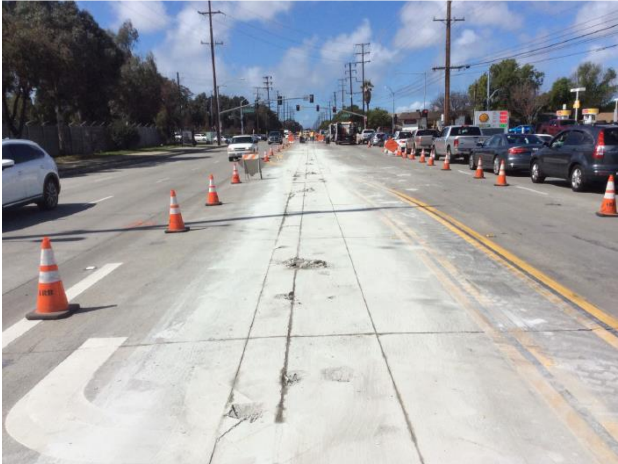
Figure 6: Traffic Control Along 190 th Street Near Crenshaw Boulevard
