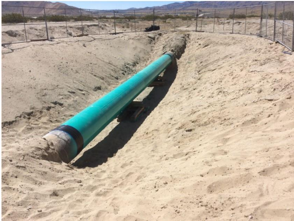
Figure 7: Feature Repair and Recoating
