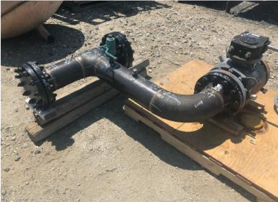
Figure 4: Prefabricated Assembly for Regulator Station
