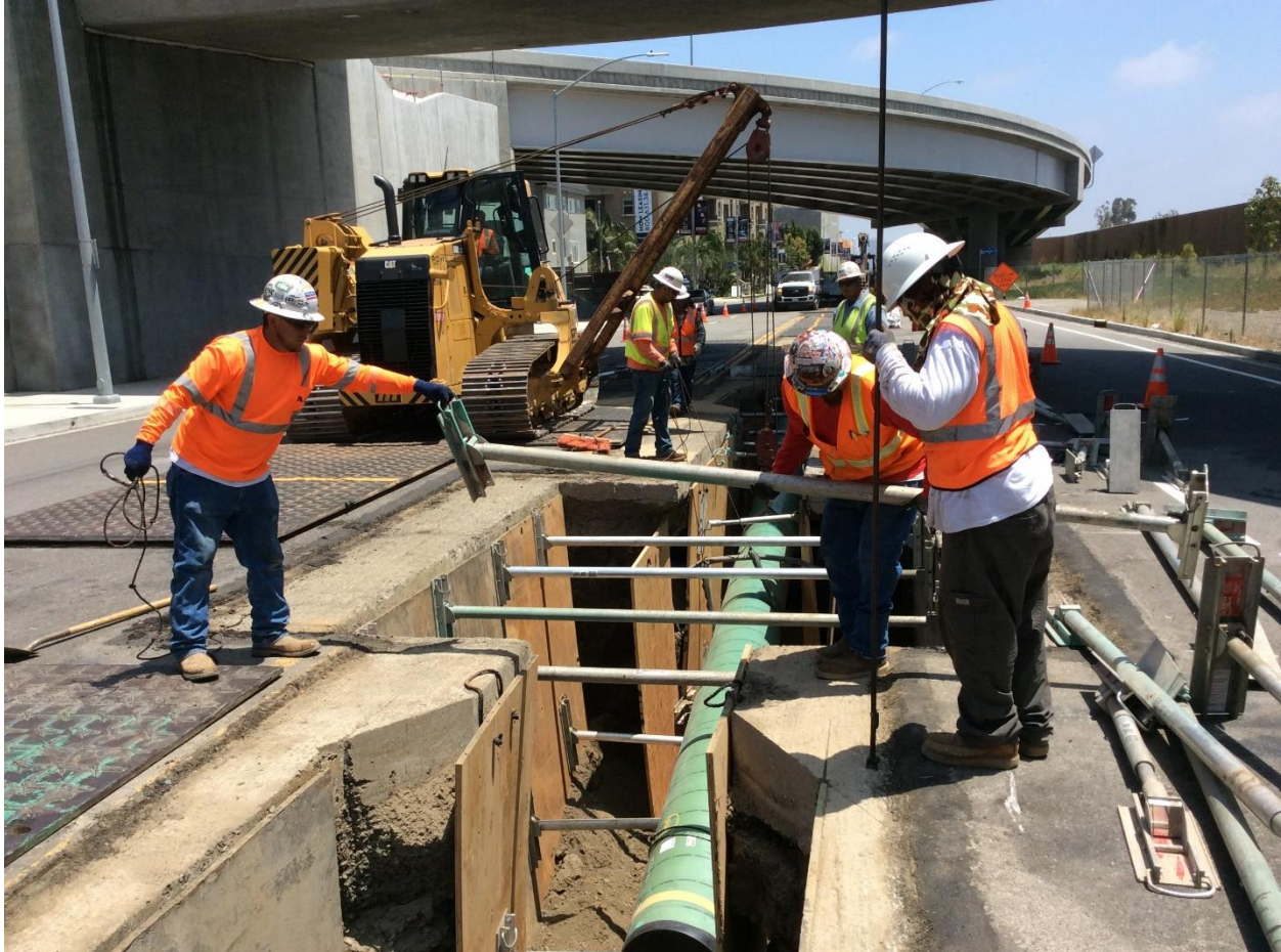
Figure 11: Removal of Hydraulic Shoring and Road Plates
