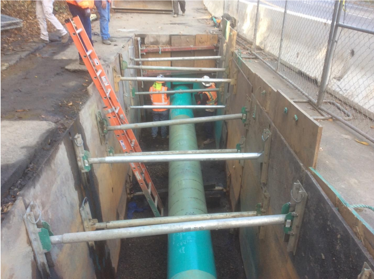
Figure 4: Prepping for Slurry and Backfill
