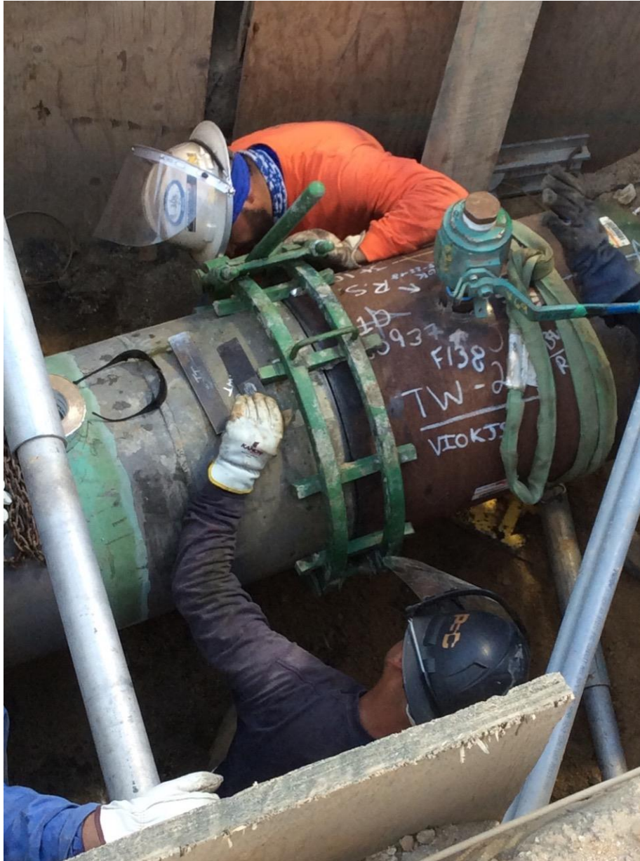
Figure 4: Installation of Isolation Cap
