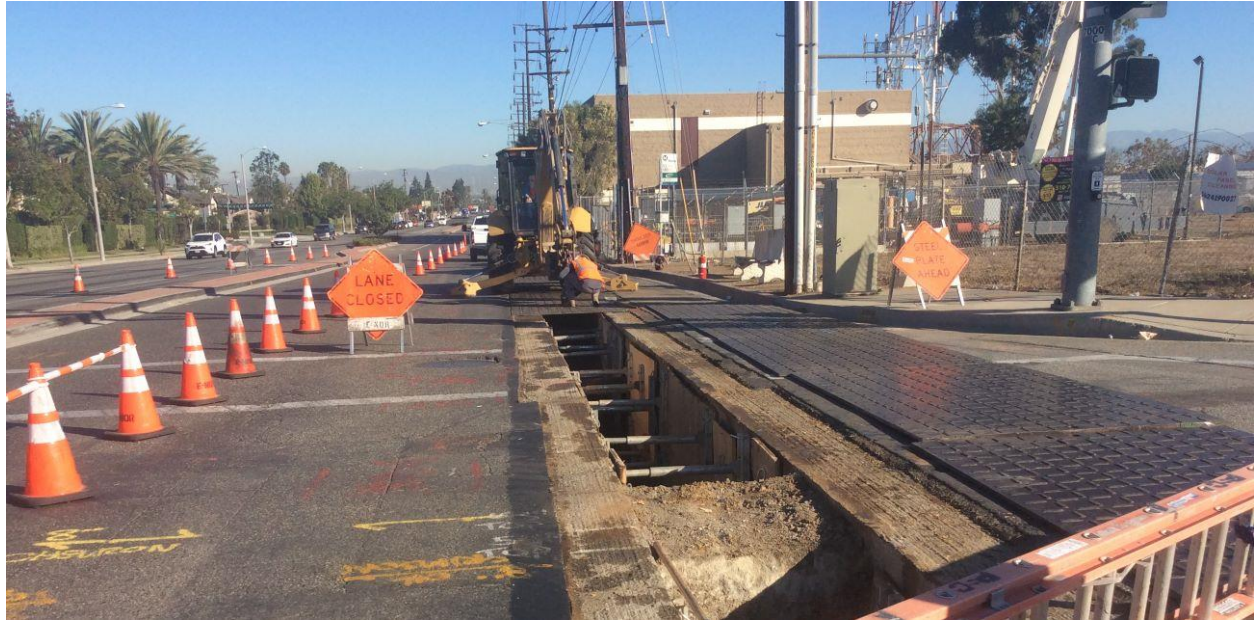
Figure 4: Workspace Along South Central Avenue
