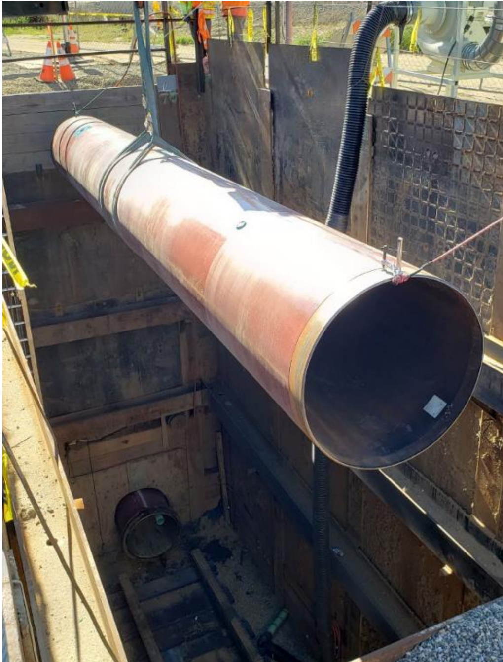
Figure 6: Lowering of Casing Pipe into Bore Pit
