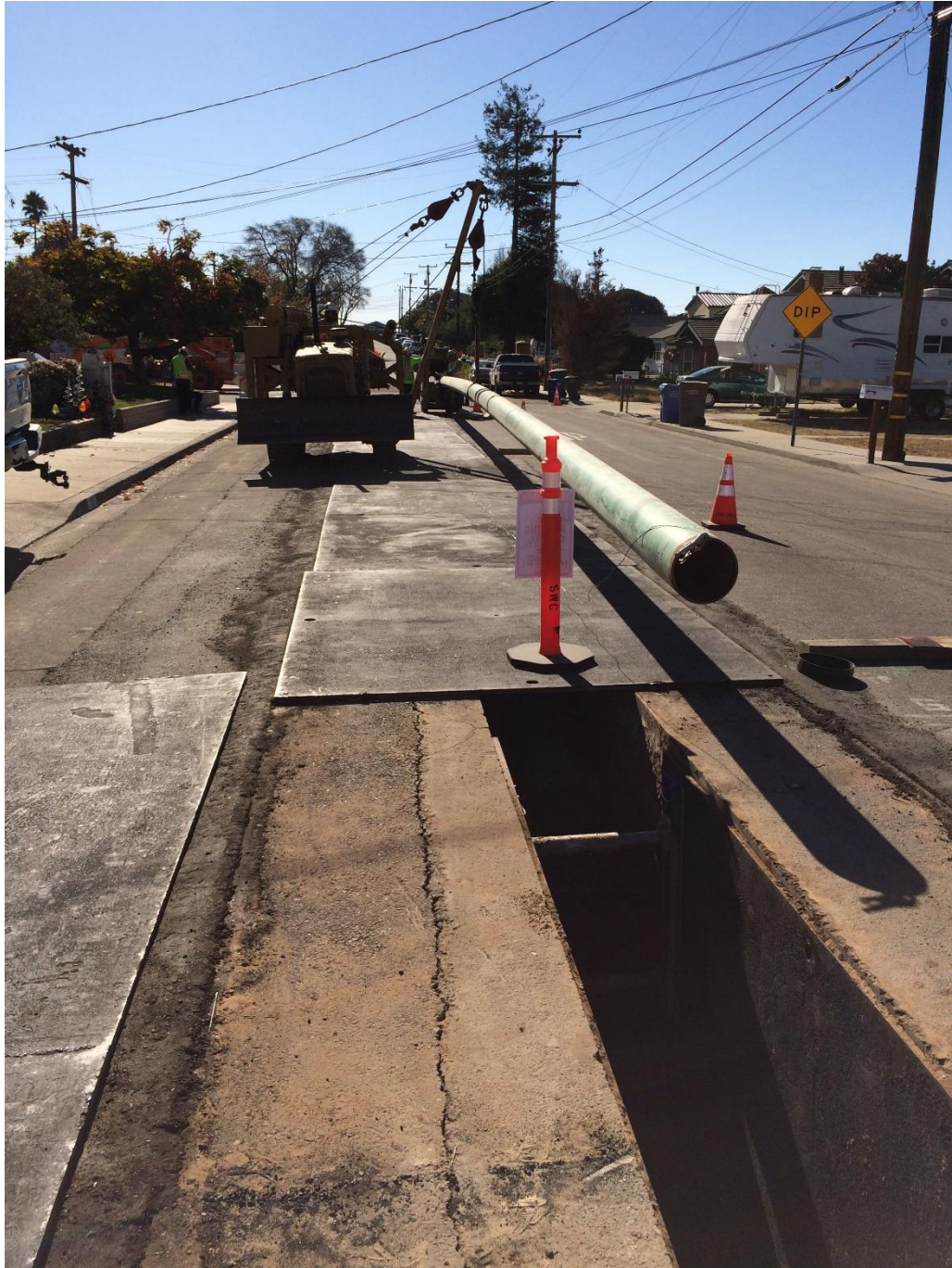
Figure 4: Pipe Strung Out Along Alpine Street
