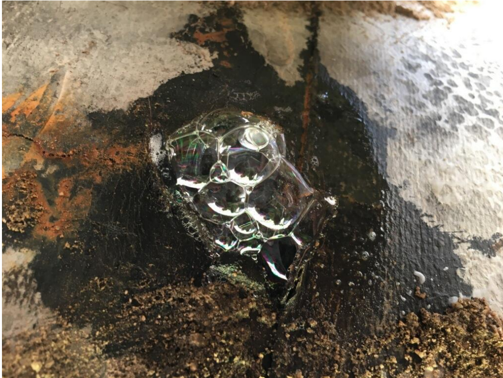
Figure 7: Leak Detection Bubbles Used to Locate Leak
