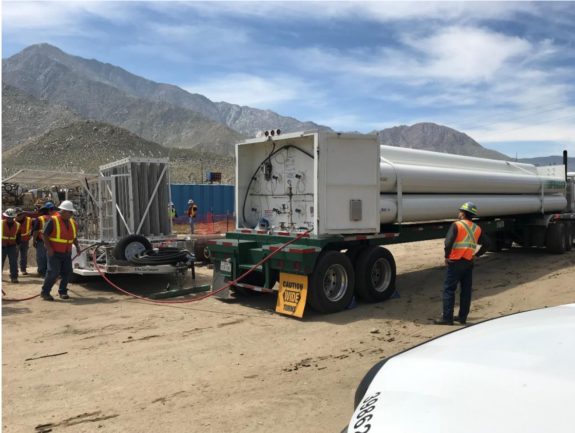
Figure 5: Helium Truck Used For Leak Detection
