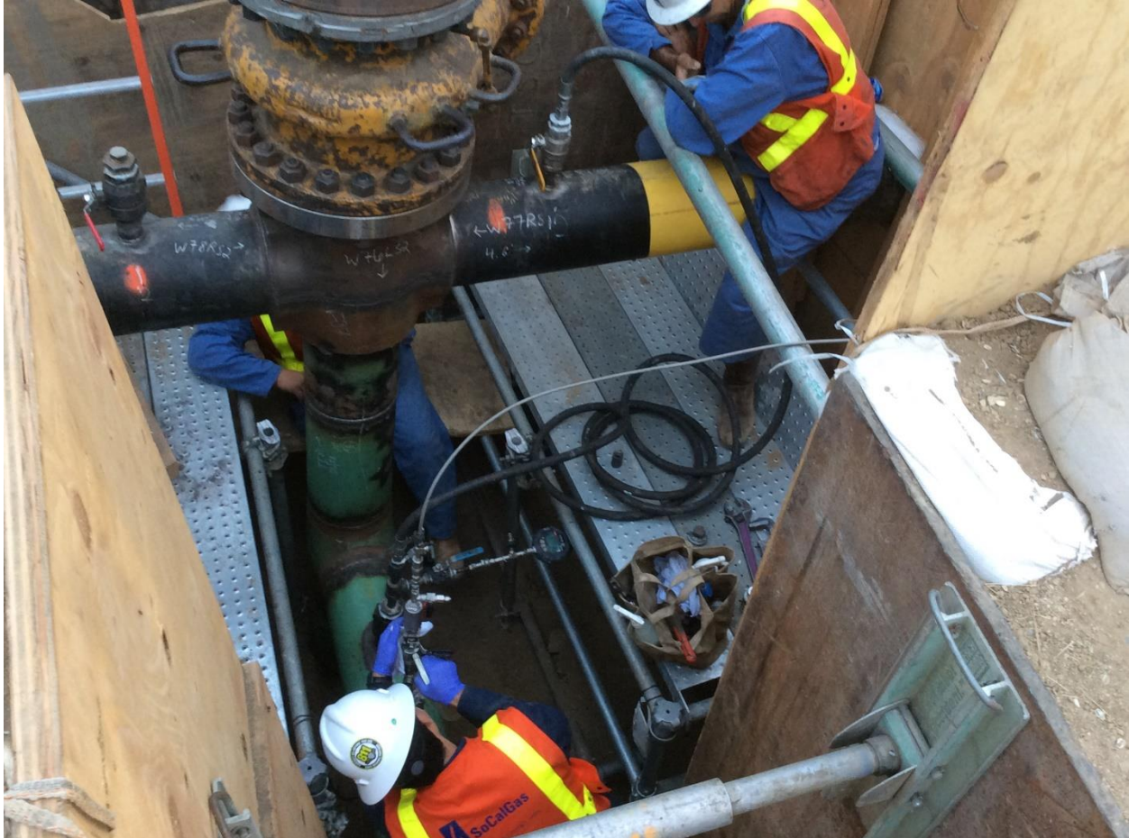
Figure 4: Checking for Leaks Before Start of Line Odorizing.
