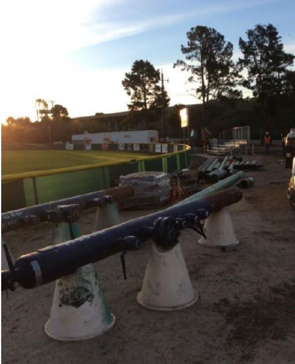
Figure 6: Test Head and Material Staging at Sports Complex
