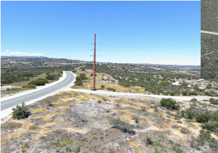
Fuels Reduction in an area along an SDG&E corridor in Tier 3 of the HFTD
