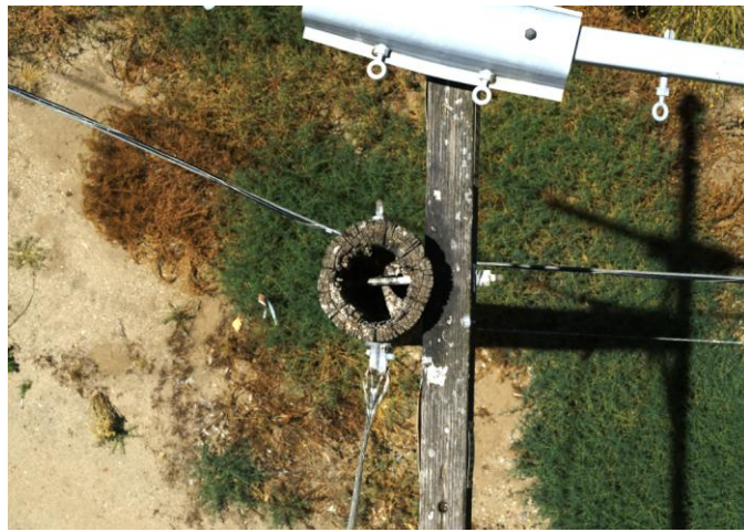
8 9 Figure JK- 1: P110290, 6/25/2020, Hollow Pole Top and view from below with no visible 10 damage.
