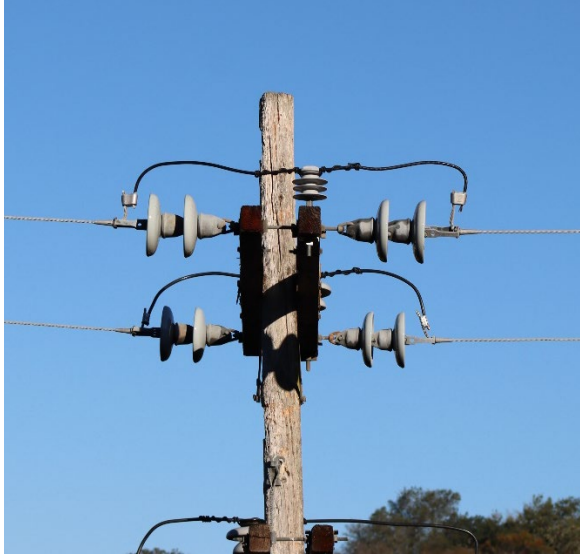
Figure 17: Top of the Incident Pole showing new, insulated jumper lines.
