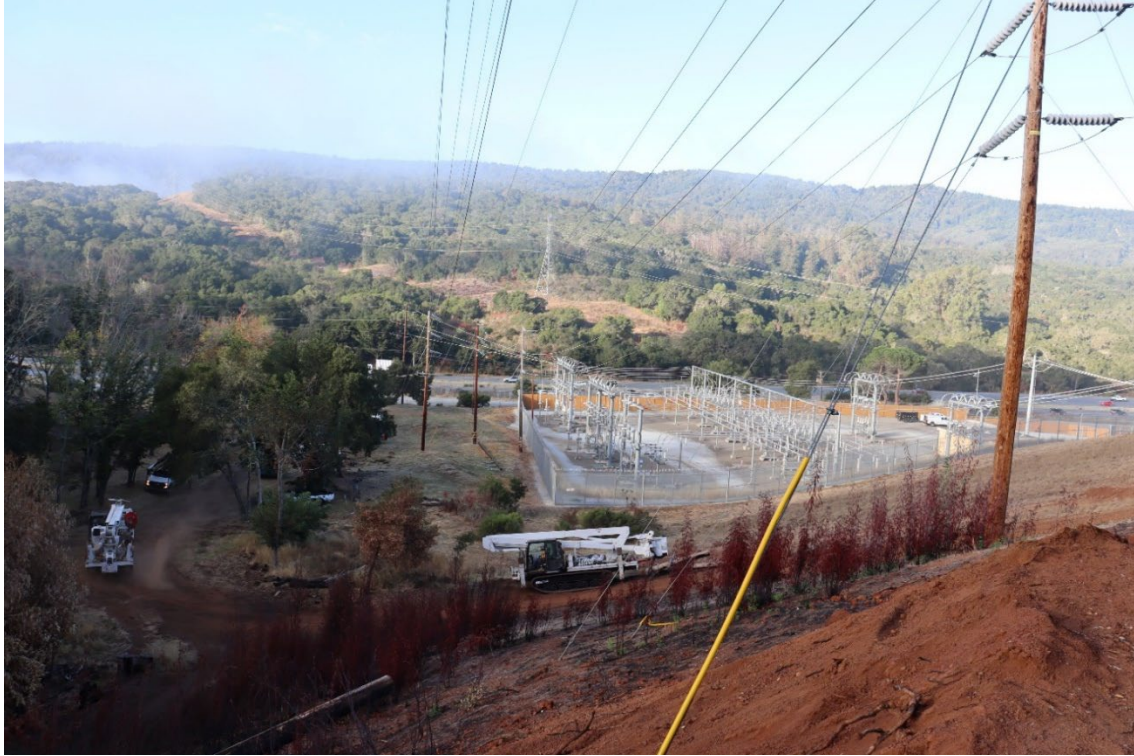
Figure 13: Staging Area for Repair Work (looking down at Jefferson Substation).
