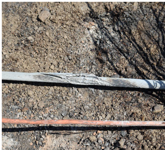
Figure 6: Damaged transmission conductor collected by CAL FIRE.
