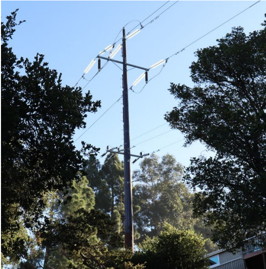
Figure 20: Pole 000/005 viewed from down the hill looking north-east.
