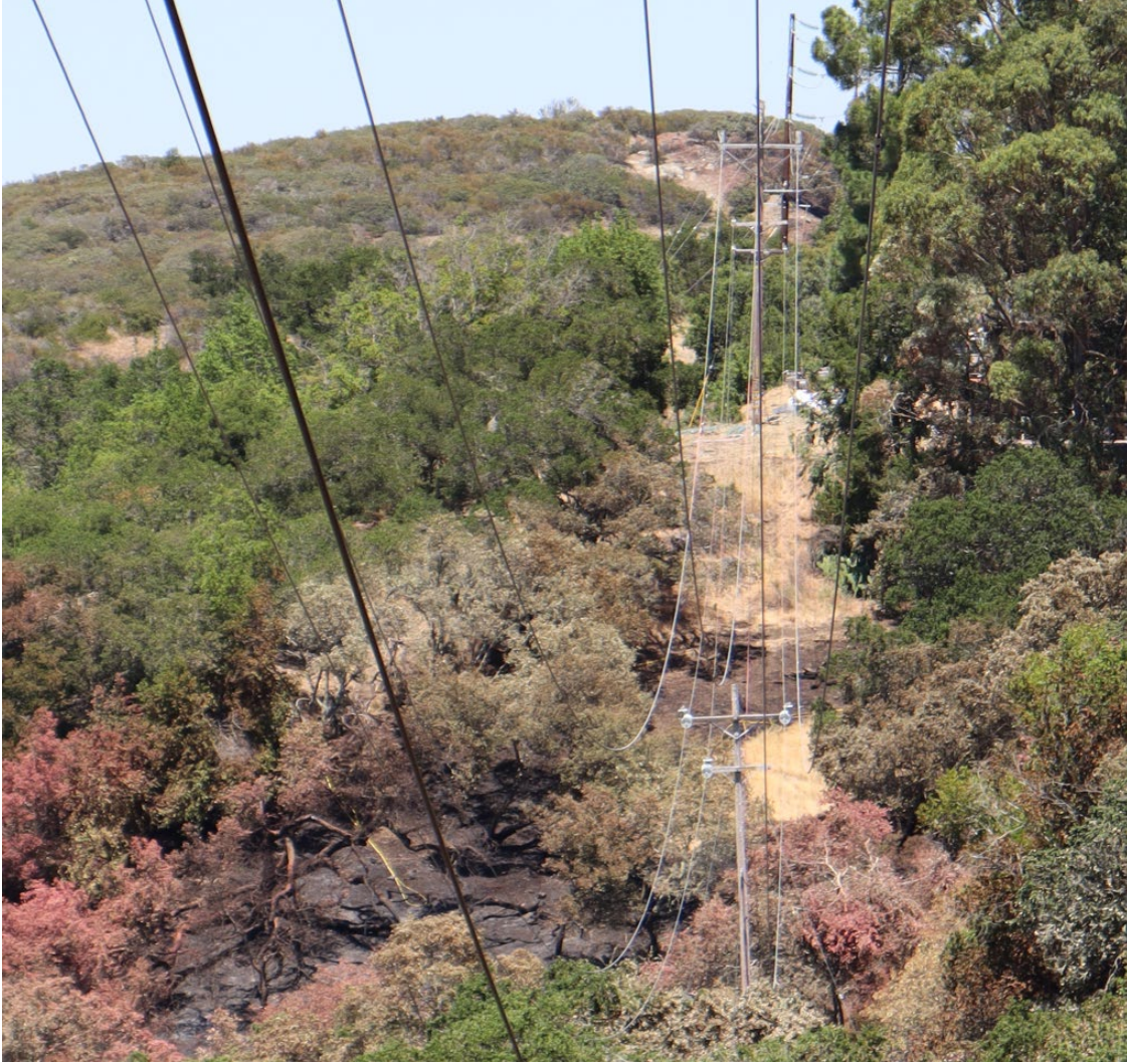
Figure 11: View from Pole 000/004 looking towards the Incident Pole and Pole 000/005.
