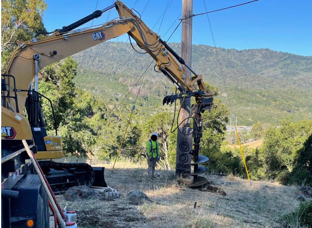
Figure 24: Excavation at Pole 000/005 the morning of June 21, 2022. 76
