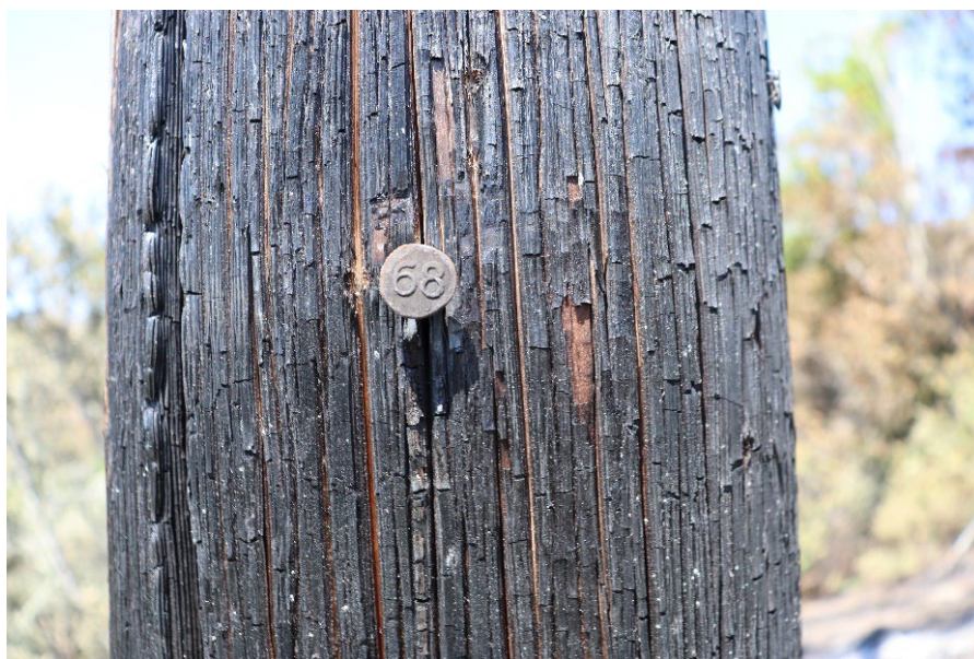
Figure 7: Tag indicating the Incident Pole was installed in 1968.
