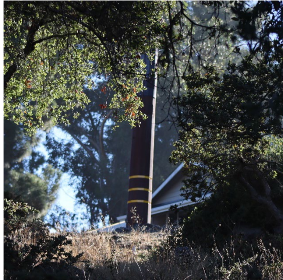
Figure 21: Bottom of Pole 000/005 viewed from down the hill looking north-east.
