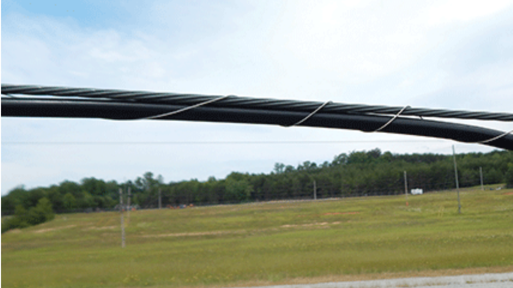
Figure 4: A messenger wire supporting a communications conductor and wrapped with lashing wire. Note that this is a stock image and that this particular communications conductor was not involved in the Woolsey Fire in any way. However, the communications infrastructure involved in the Woolsey Fire was very similar to that depicted in the image.
