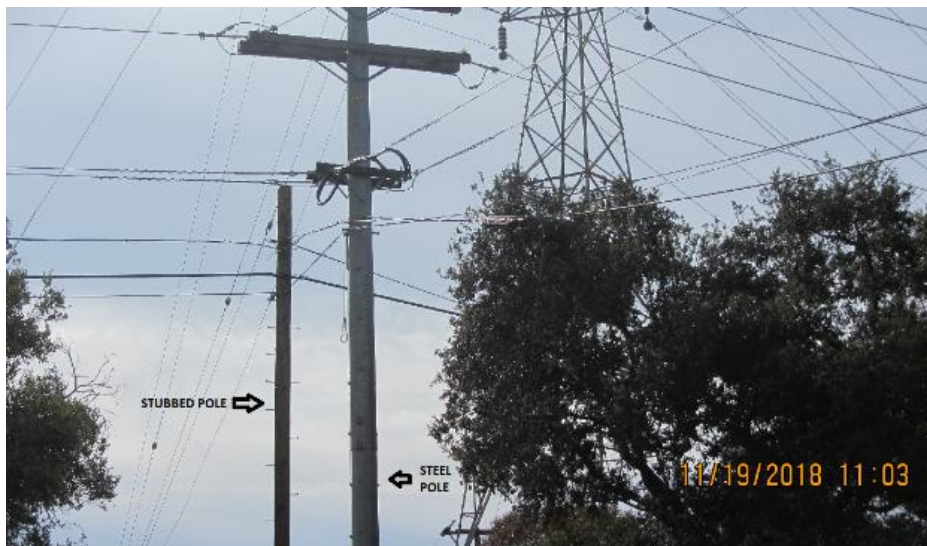
Figure 15: The Steel Pole and Stubbed Pole as viewed from the northeast.
