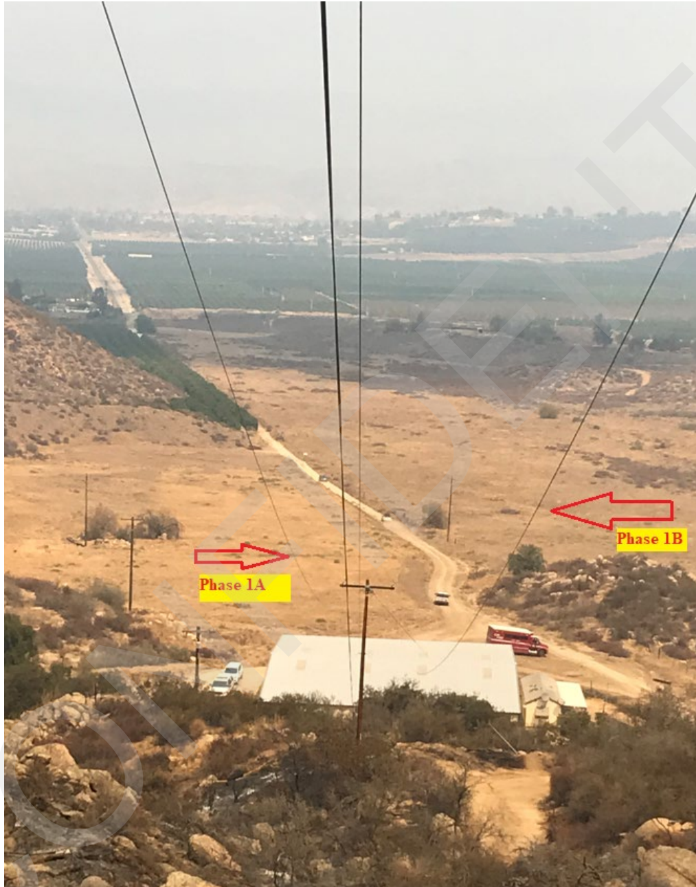
Figure 27: View of the Incident Span from the top of the hill taken by SCE on September 7, 2022.
