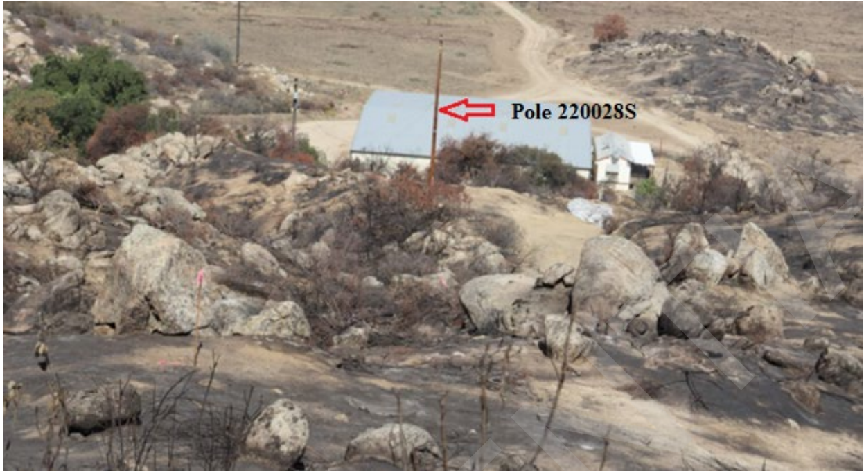
Figure 7: View of Incident Span between Incident Pole 220029S at the top of hill (behind the camera) and Pole 220028S (brown pole in front of barn).
