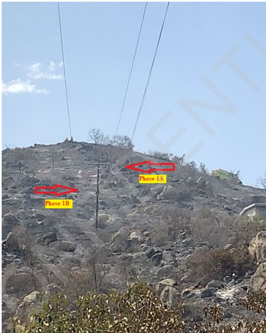
Figure 28: Southern view of the Incident Span taken by SCE on September 7, 2022. 52
