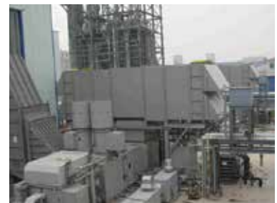
FIGURE 13: A: Frame 9E.03 operating on steel mill gases at a plant in China; B: LM2500+ operating on high H 2 coke oven gas
