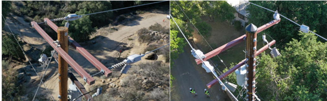
Figure I-24 Dead-end Structure (left) and Tangent Structure (right)
