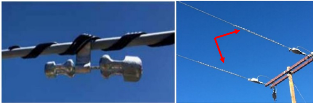
Figure I-23 Types of Vibration Dampers: Stockbridge Damper (left) and Spiral Damper (right)
