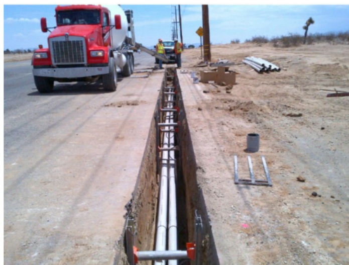
Figure I-3 Open Trenching Housing a Conduit Bank
