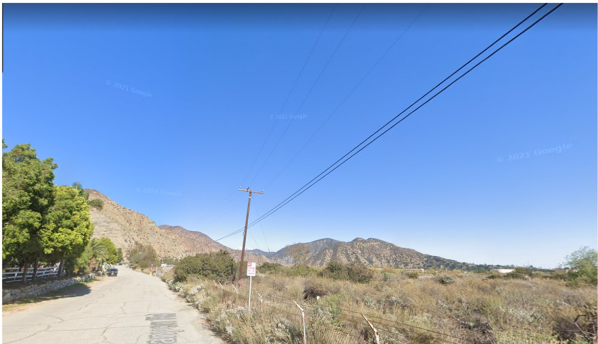
Figure I-16 Photo of Location Confirms Covered Conductor as Appropriate Mitigation
