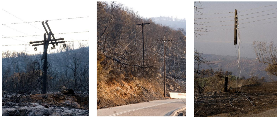
Figure 5: Damaged lines and poles from the 2007 forest fires in Greece (Courtesy: Public Power Corporation, Greece).
