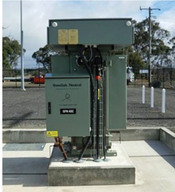
FIGURE PG&E-7.3.3-5: ARC SUPPRESSION COIL / GFN
