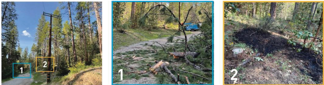
FIGURE PG&E-22-11-2: COVERED CONDUCTOR EFFECTIVENESS – EXAMPLE 2
