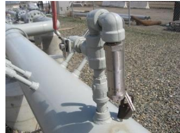
1 Thermal Relief Typical Installation
