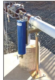
Typical above-ground filter installation
