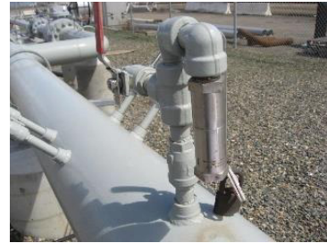
1 Thermal Relief Typical Installation
