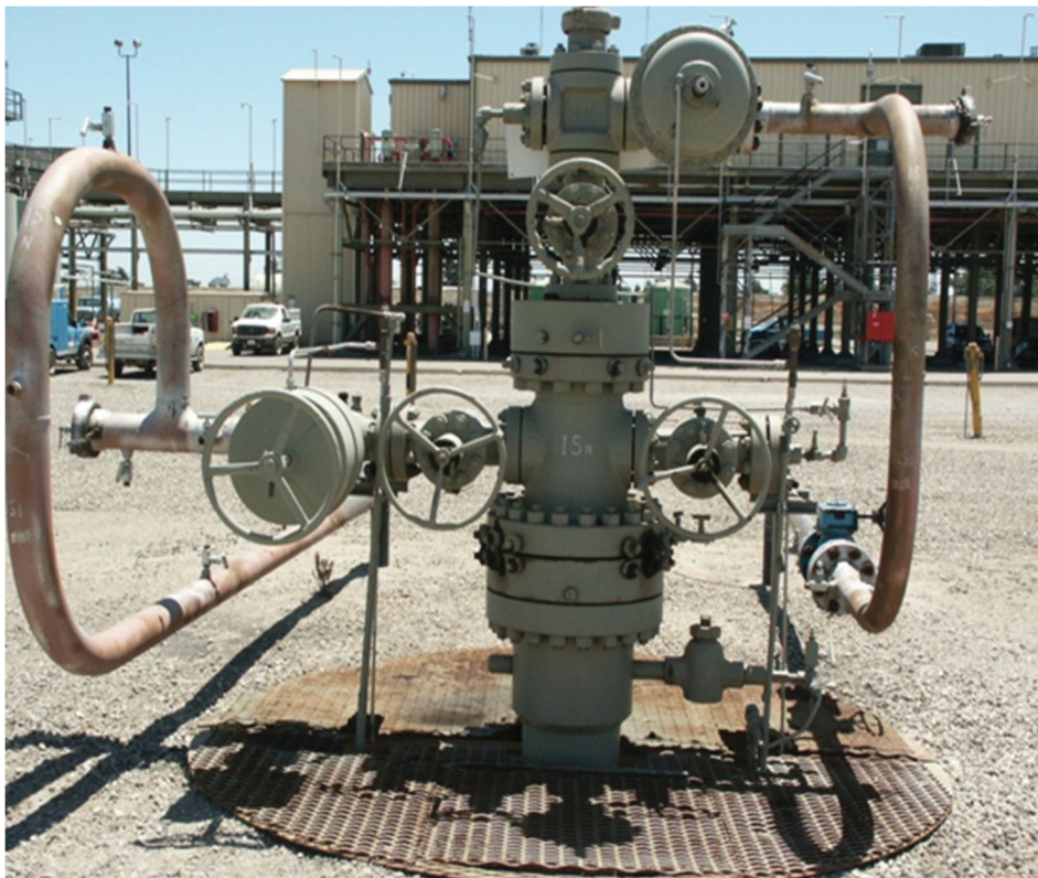
Figure J-1. A Typical PG&E Christmas Tree.
