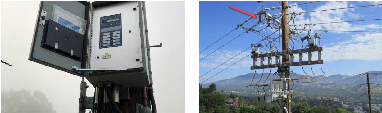
Figure SCE 8-15 - A Remote Control Box (left) and Remote Automatic Recloser (RAR) Switch (right)
