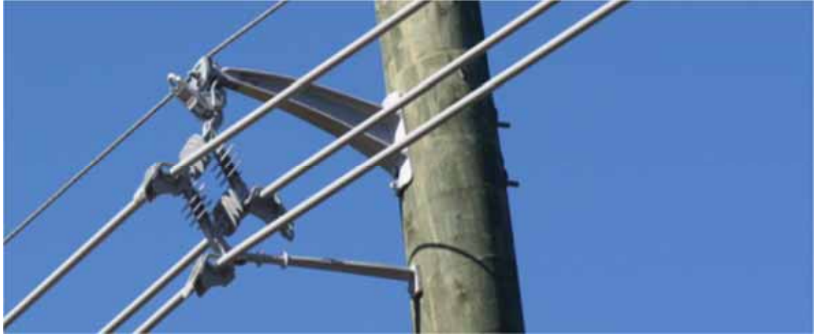
Figure II-2 Spacer Cable System
