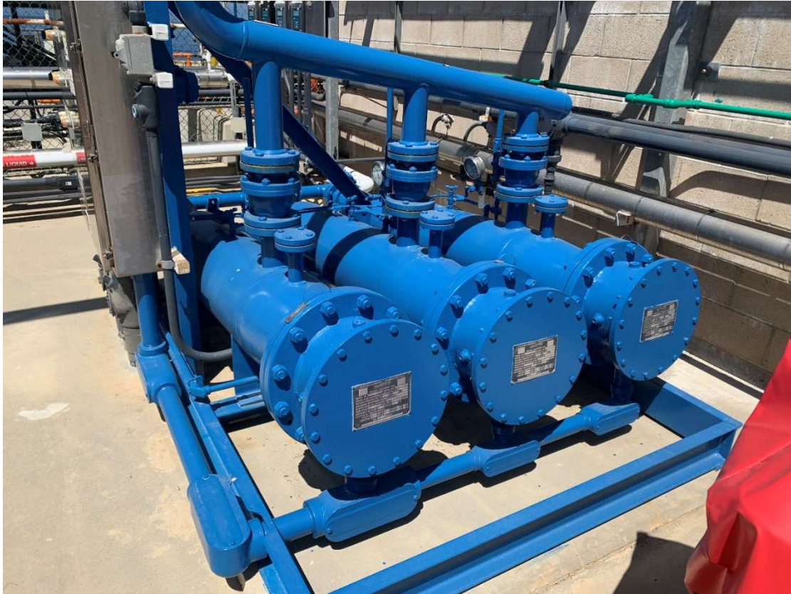
Catalina Gas Vaporizer – 3 independent trains
