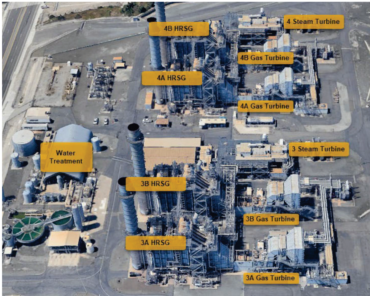
1 Figure 3-1 Mountainview Station – Aerial View of Unit 3 and Unit 4 137, 138
