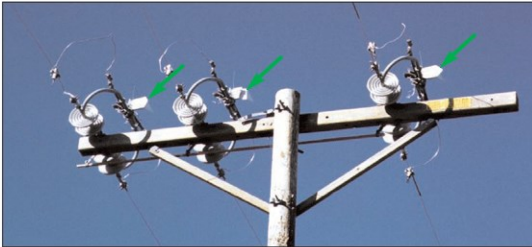
Figure B-24: 600 Amp KPF Air Switch, Crossarm Construction (Closed Position) with Arcing Horns and Snuffers
