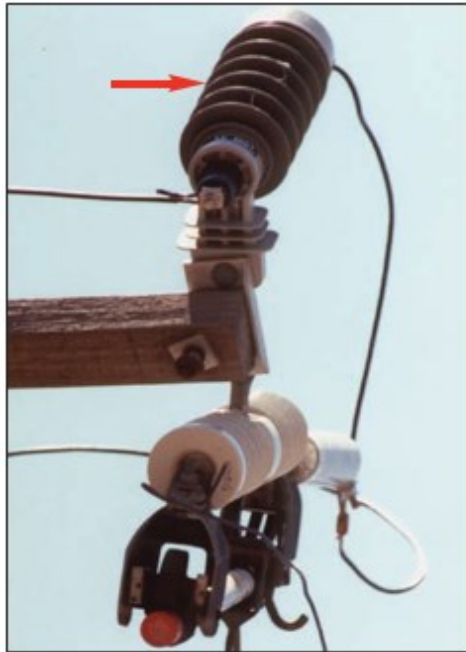
Figure NE-23: Non-Porcelain Lightning Arrester
