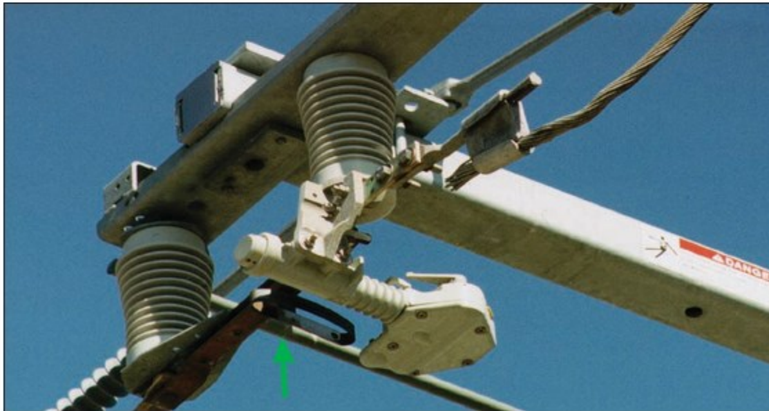
Figure B-31: S&C Omni-Rupter 600 Amp Underarm Side Break Switch (Closed Position)
