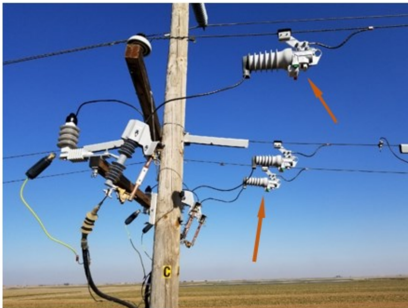
Figure A-4: Conductor Mounted Fusesaver with in-line solid blades
