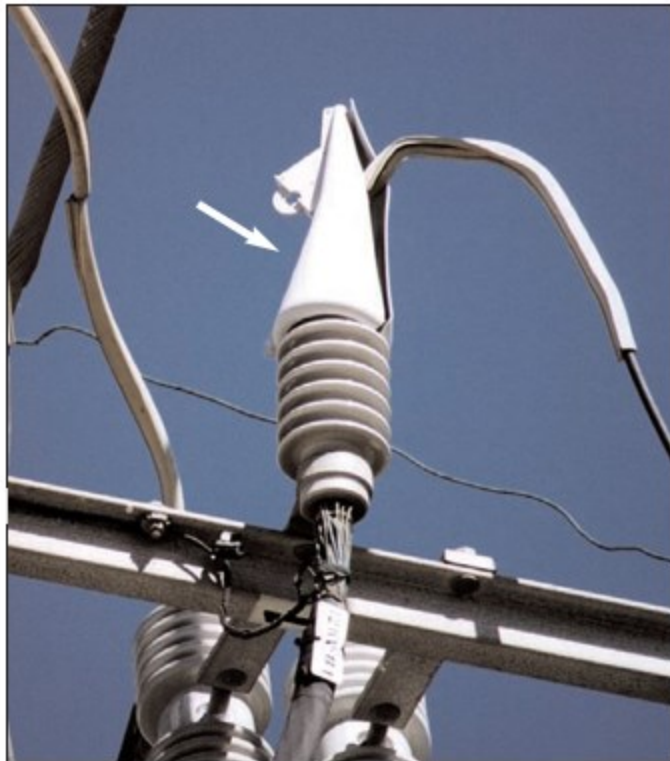
Figure PLC-23: Close up of Squirrel Guard
