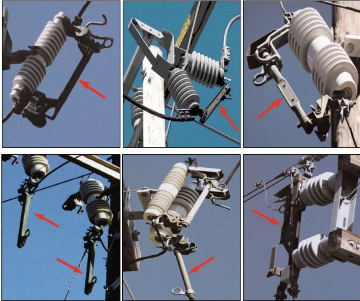
Figure NE-13: Solid Blade Disconnects
