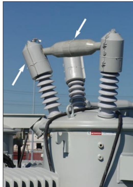
Figure PLC-26: Bushing Covers
