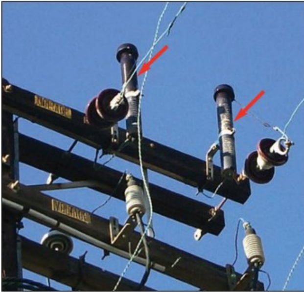
Figure NE-27: Lightning Arrester
