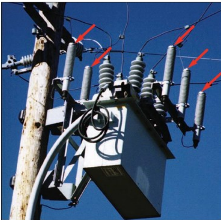
Figure NE-20: Lightning Arrester (with Recloser)
