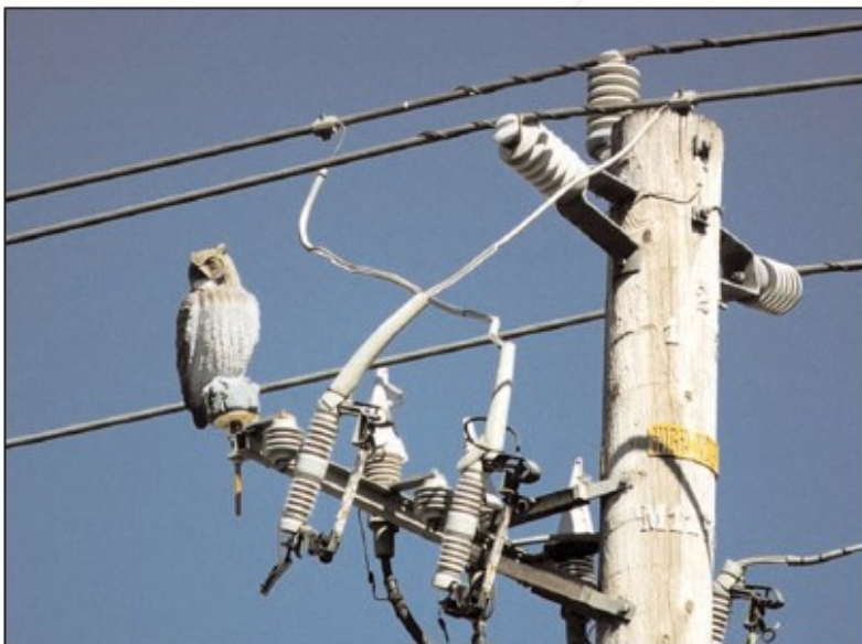
Figure PLC-20: Anti-Perch Owl
