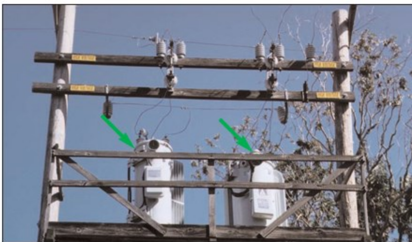
Figure B-49: Voltage Regulator
