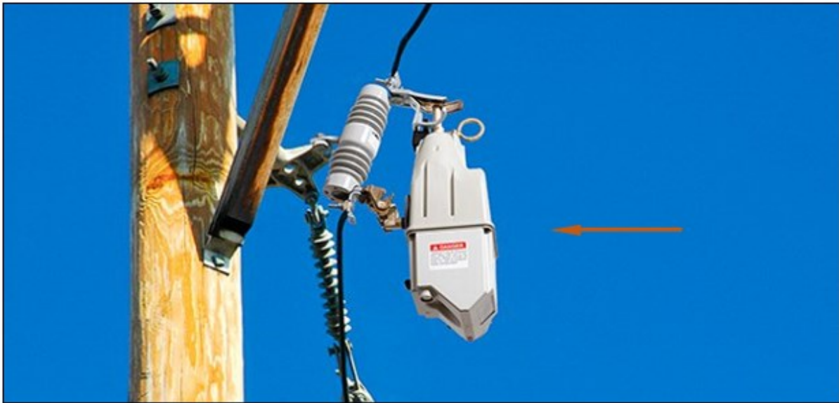
Figure A-6: Trip Saver II Cutout mounted single phase recloser
