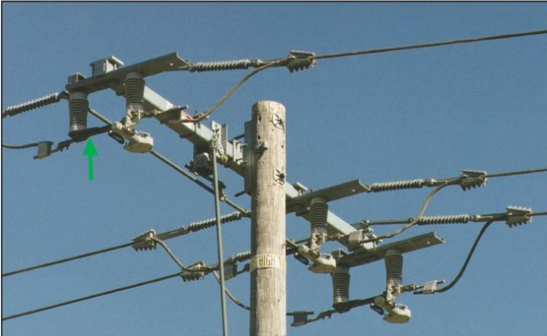
Figure B-30: S&C Omni-Rupter 600 Arm Underarm Side Break Switch (Closed Position)
