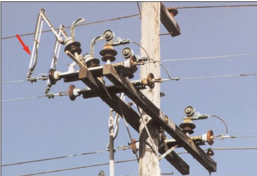
Figure NE-39: Grasshopper Air Switch (open position)
