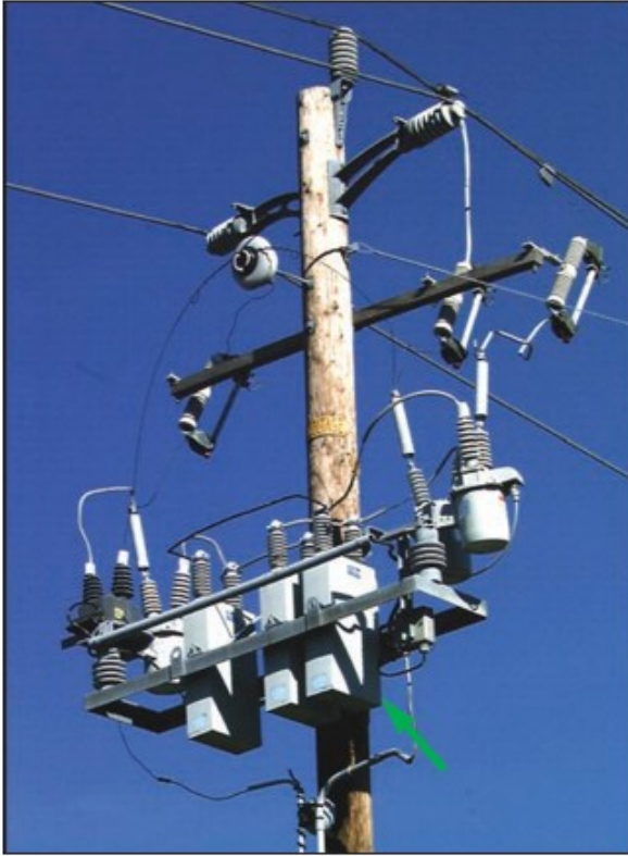
Figure B-50: Capacitor Bank
