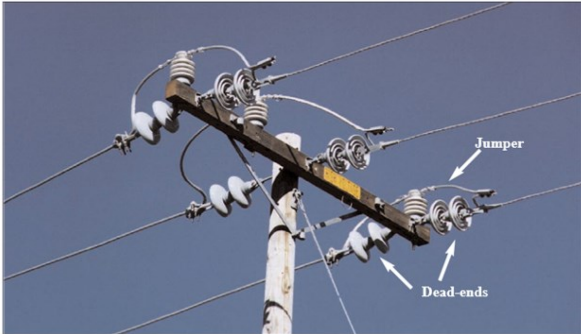
Figure PLC-7: Crossarm Double Dead-end
