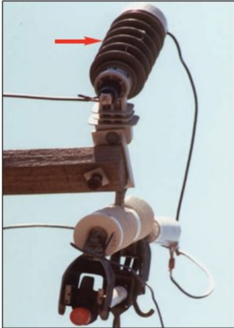
Figure NE-23: Non-Porcelain Lightning Arrester
