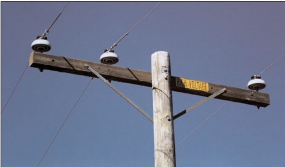
Figure PLC-4: Crossarm (Tangent)
