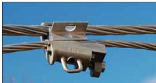
Figure B-71: CPI Wedge Connectors on Line
