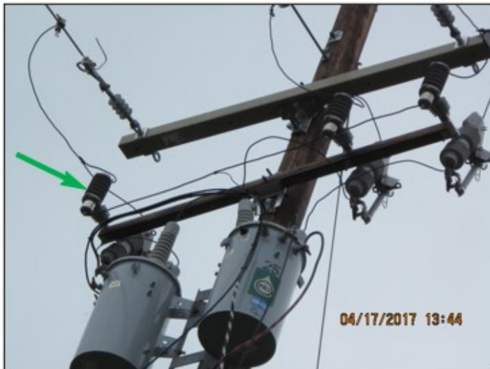
Figure B-87: Siemens Lightning Arrester
