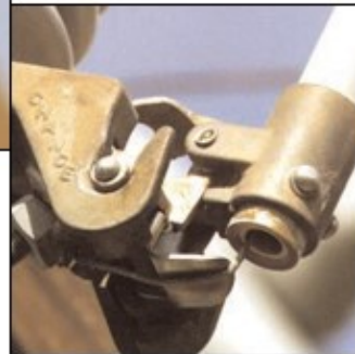
Figure NE-2: Universal Fuse, Fuse Link, and Expulsion End of Fuse
