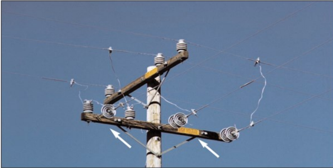
Figure PLC-5: Tangent Crossarm with Dead-end Tap (T-Tap)
