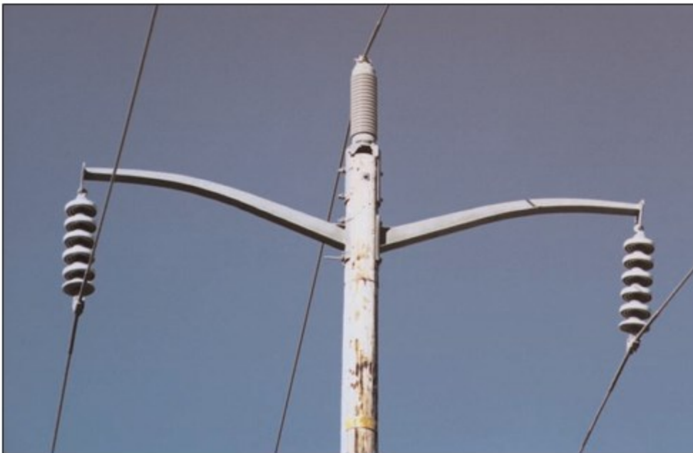
Figure PLC-31: Gull Wing
