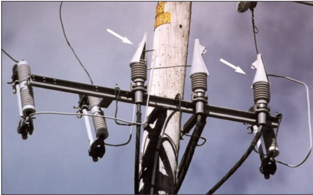
Figure PLC-22: Squirrel Guard
