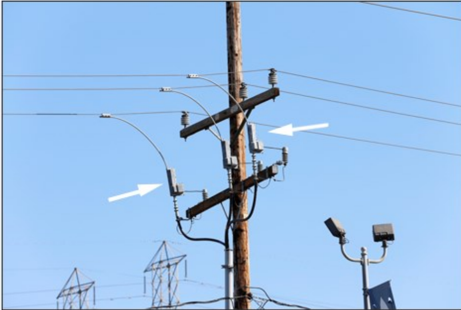
Figure PLC-15: Termination with animal protection cover
