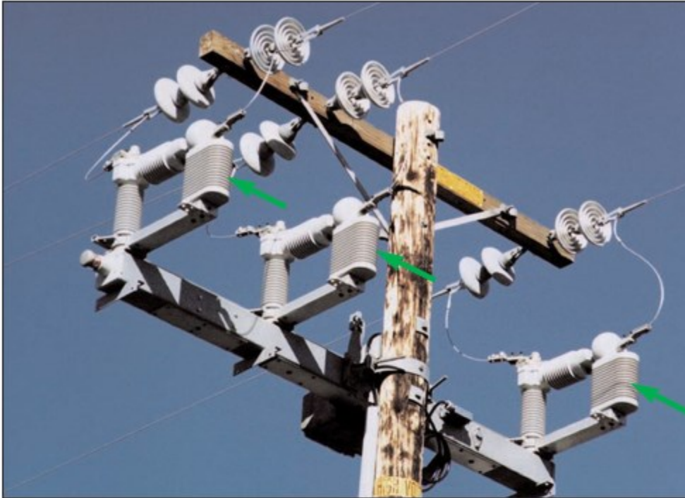
Figure B-37: S&C Scada-Mate Switch
