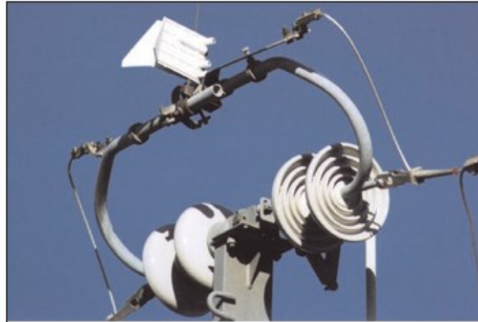
Figure B-22: 600 Amp KPF Air Switch, Triangular Construction (Closed Position)
