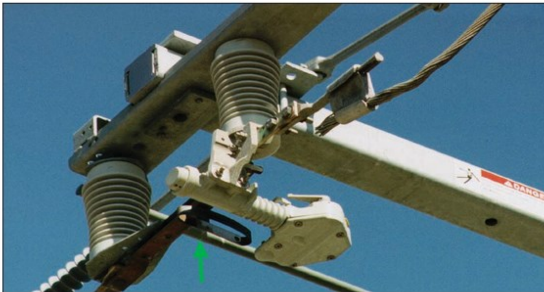
Figure B-31: S&C Omni-Rupter 600 Amp Underarm Side Break Switch (Closed Position)
