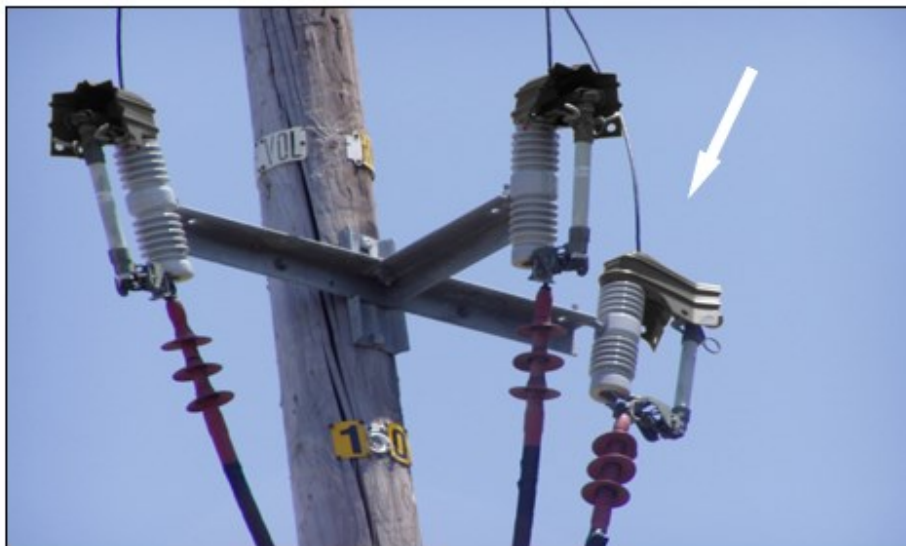
Figure PLC-16: Cut-out animal protection covers
