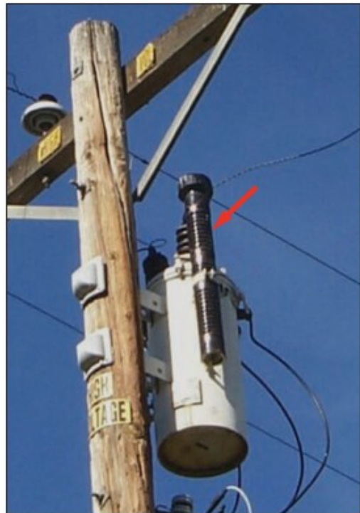
Figure NE-28: Lightning Arrester
