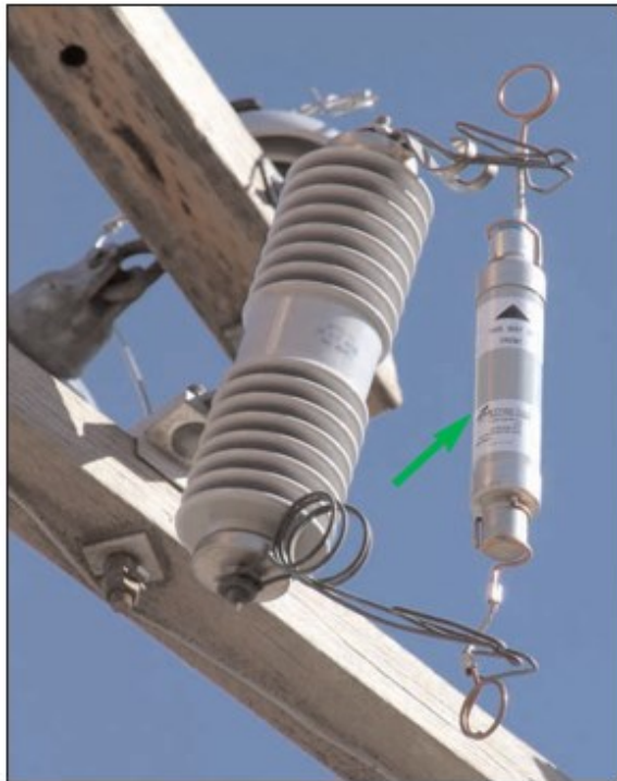
Figure B-12: Also Fits "Open Link" Cutouts
