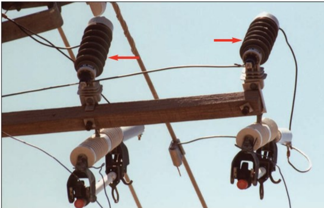
Figure NE-24: Non-Porcelain Lightning Arrester
