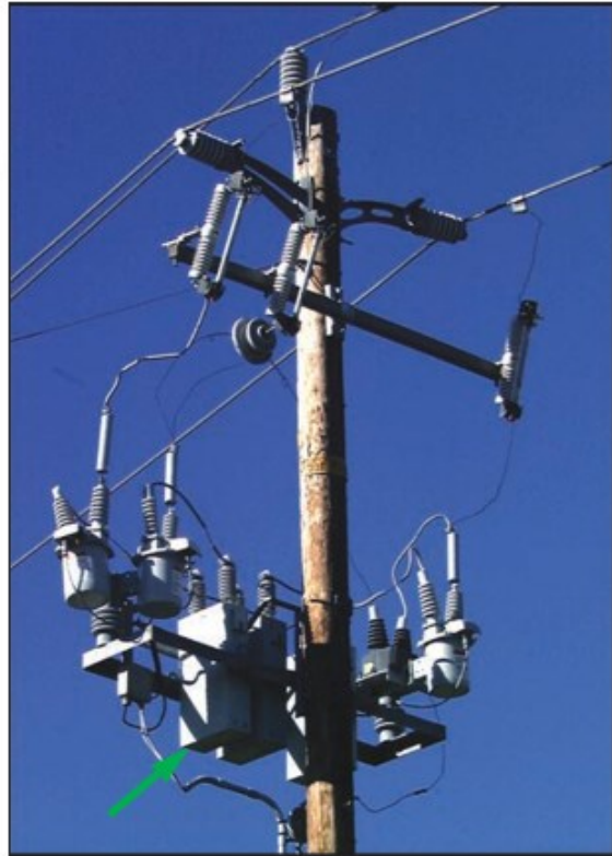
Figure B-51: Capacitor Unit
