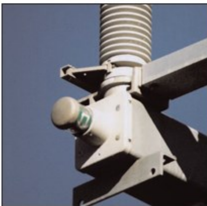
Figure B-38: Open Position Indicator Green Letter "O"
