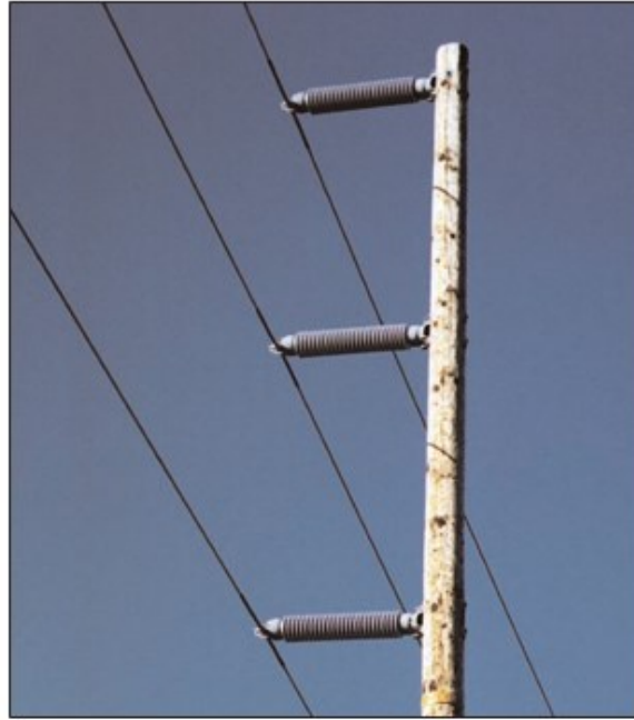
Figure PLC-28: Vertical Post
