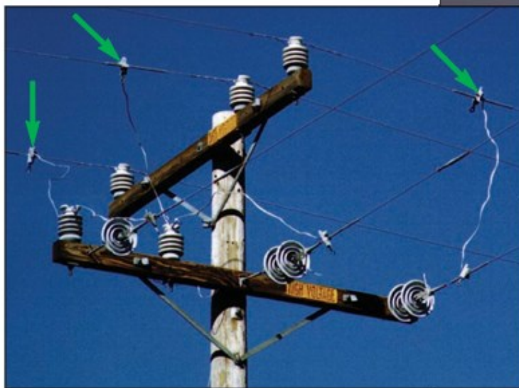
Figure B-60: Hot Tap Clamps on conductor
