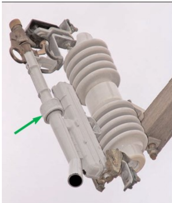
Figure B-20: S&C Fault Tamer Fuse
