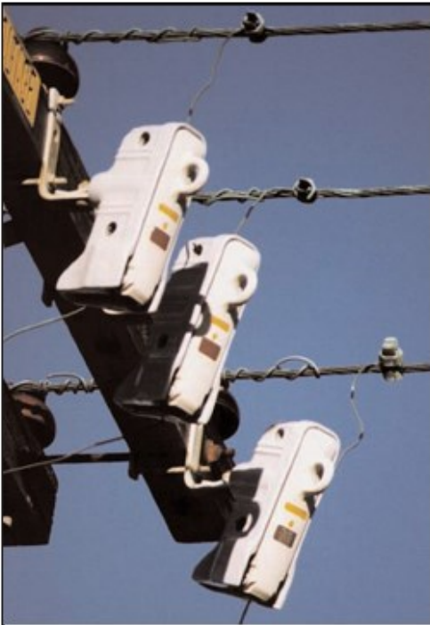
Figure NE-8: Enclosed Cutouts
