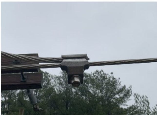
GA9000 Parallel Groove Connector on Conductor
