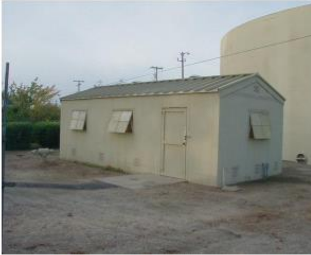
Photo 1. Existing Pump Building
