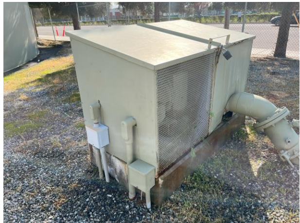
Photo 4. Existing Pump E Shelter
