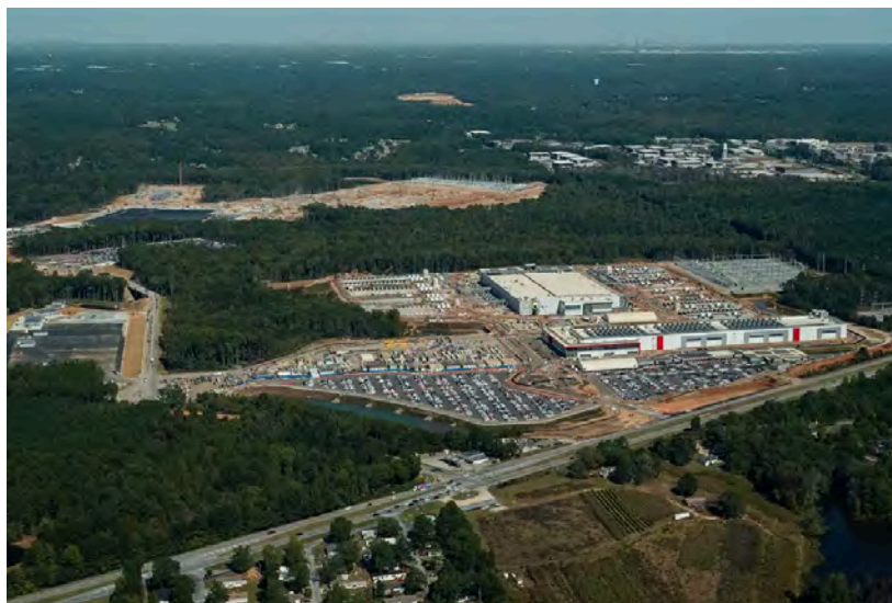
A QTS data center complex under development in Fayetteville, Ga. Elijah Nouvelage/Bloomberg
