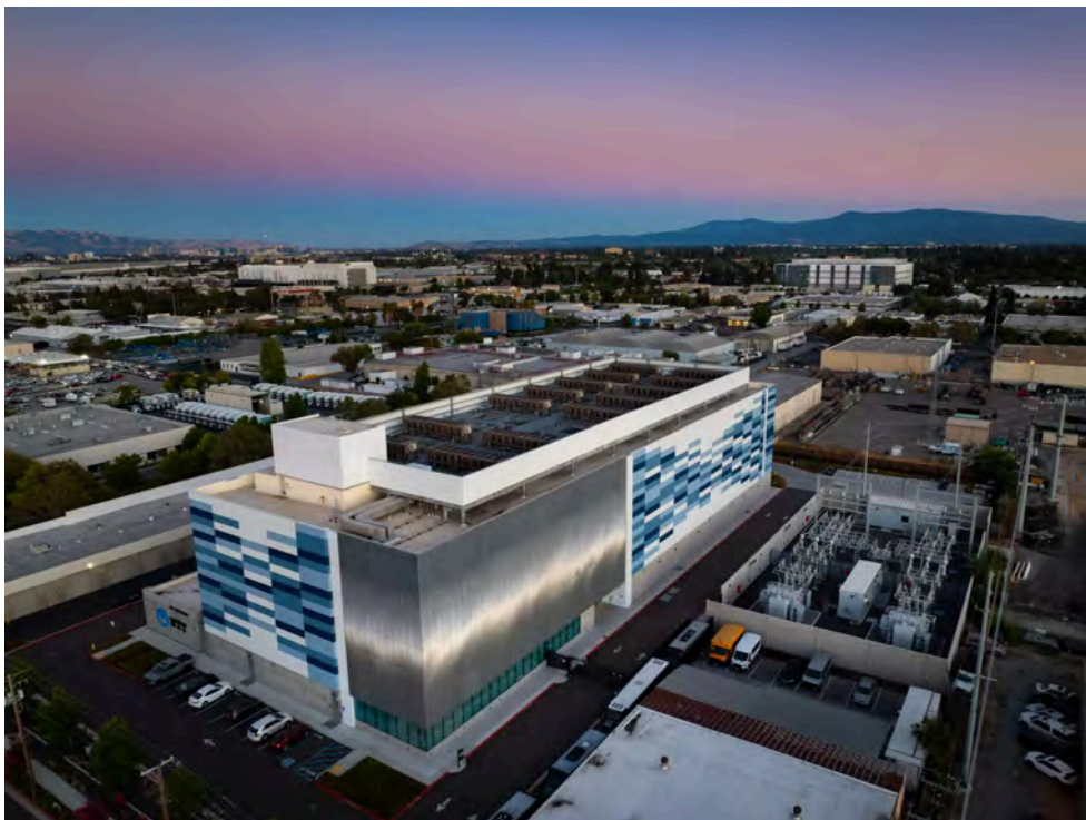
A large NTT data center rises in a Santa Clara neighborhood. (Paul Kuroda / For The Times)
