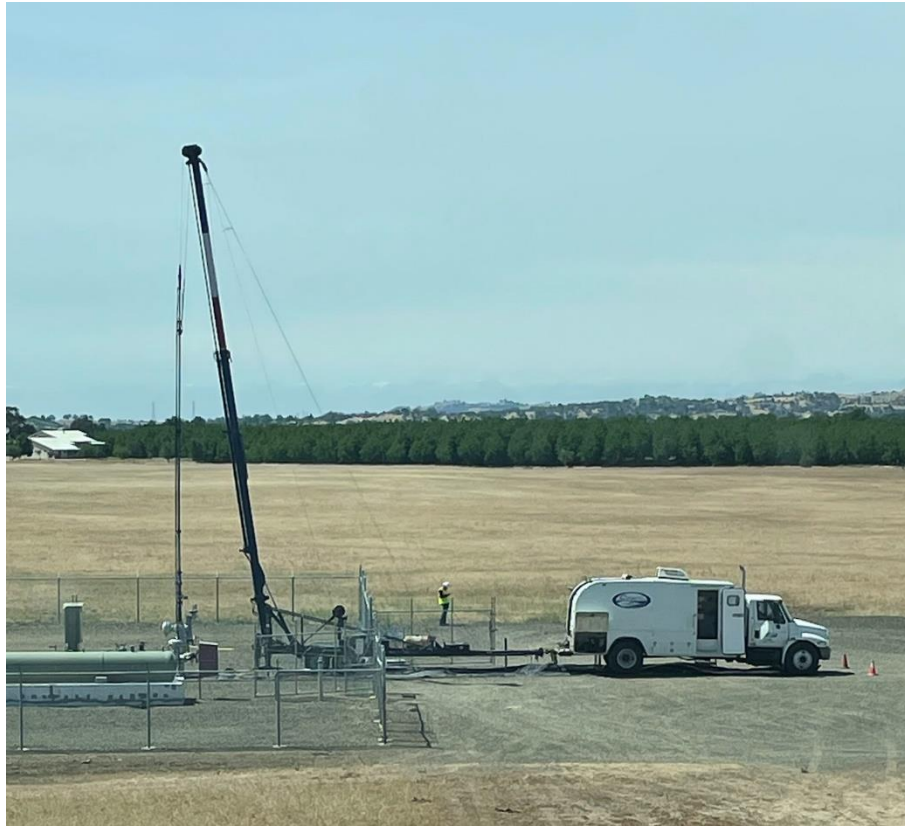
FIGURE 7-4 WIRELINE THRU-TUBING ON A WELL
