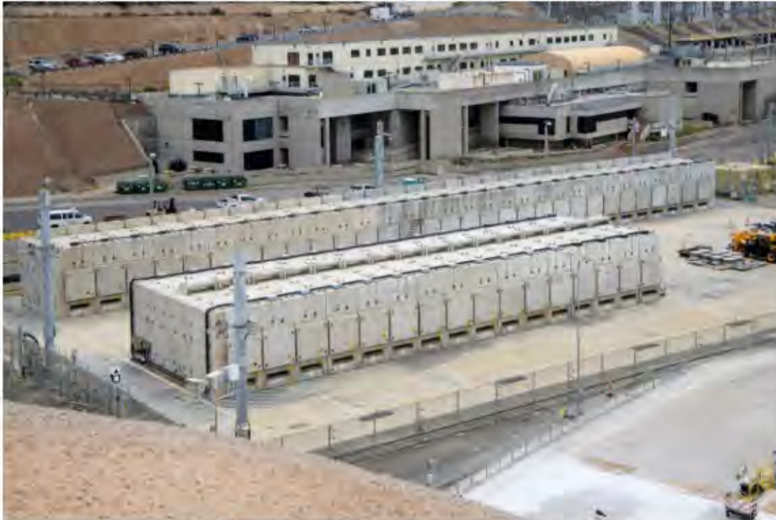
Figure 3.1 The Advanced NUHOMS® System at the SONGS TN ISFSI
