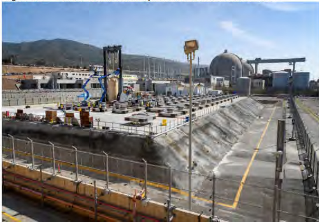
Figure 3.2 The HI-STORM UMAX System at the SONGS Holtec ISFSI
