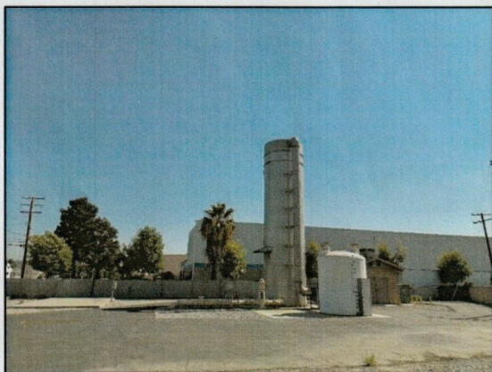
Existing Air Stripping Tower for Water Treatment and removal of VOCs.
