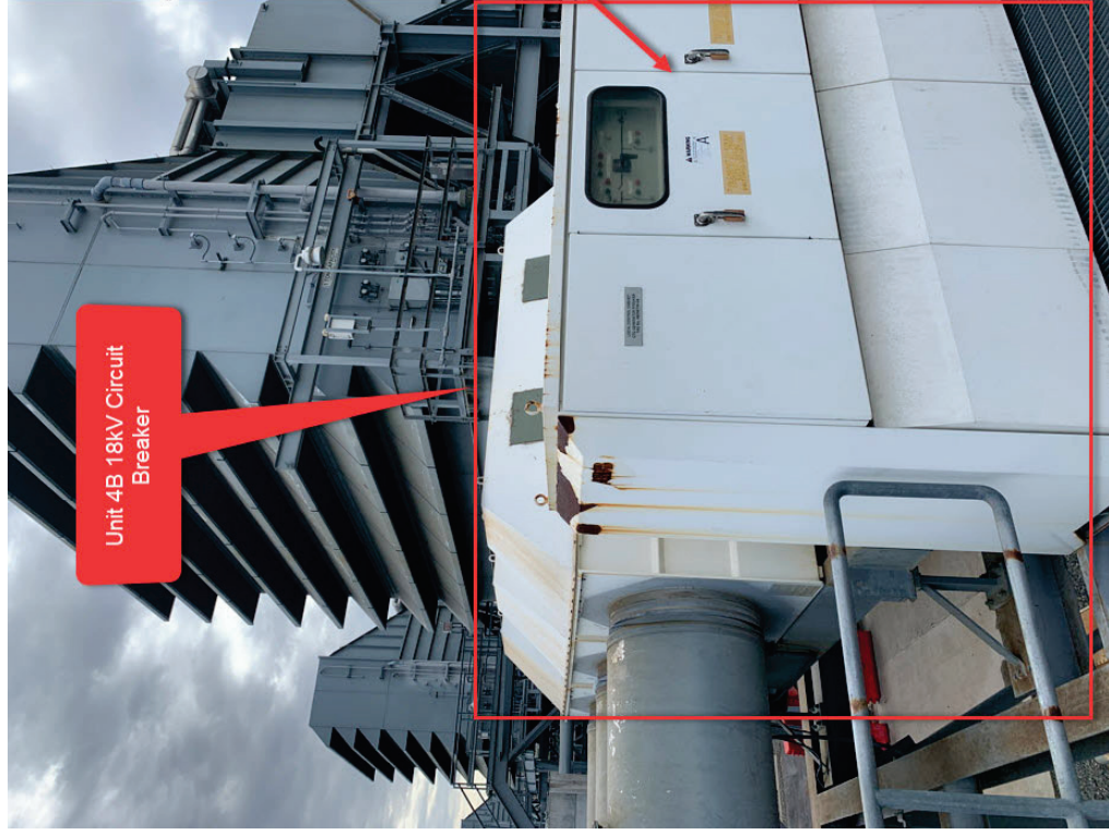
Figure 3-4 Photo of the Mountainview Station Unit 4B 18kV Circuit Breaker 177
