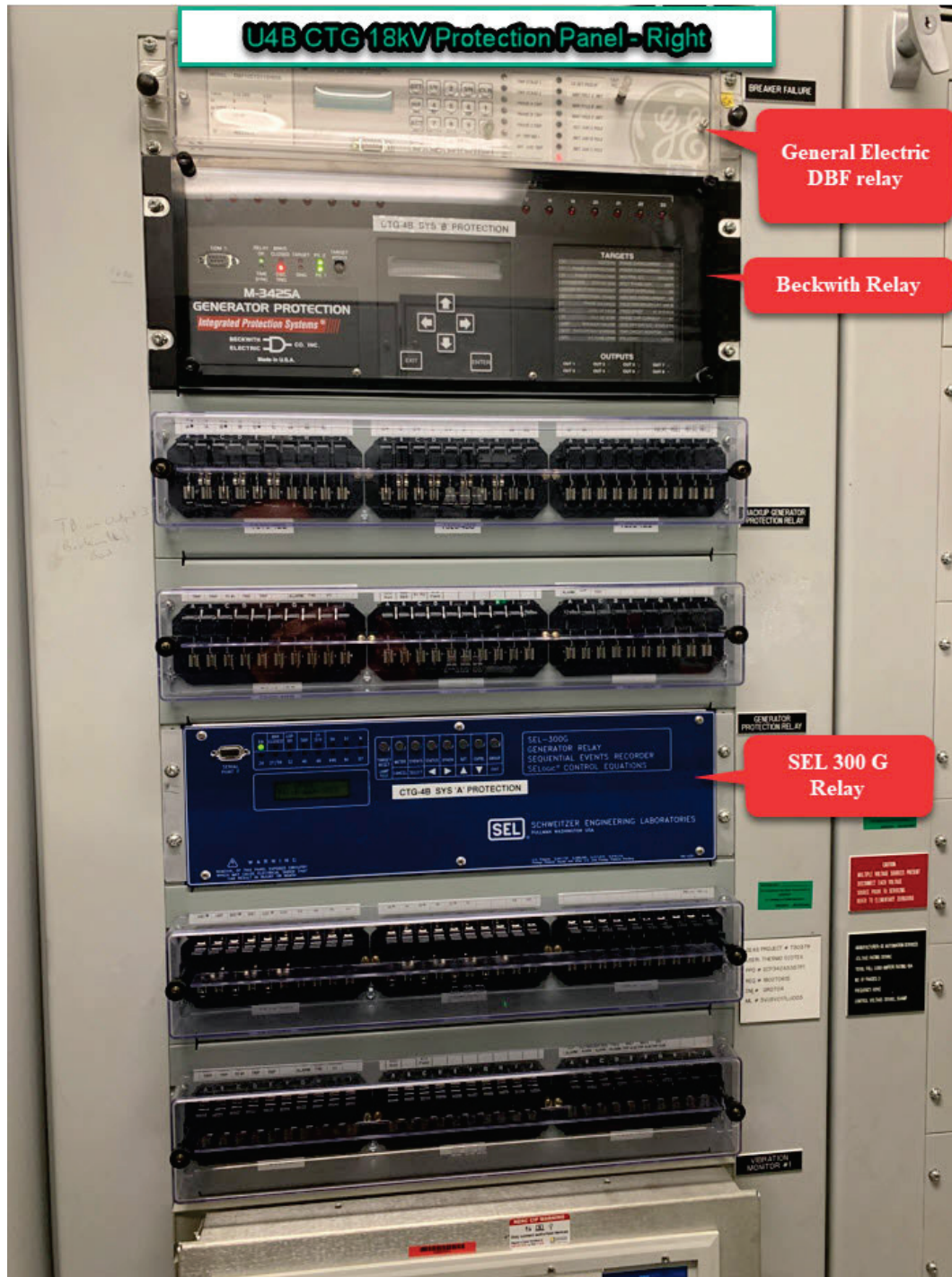
Figure 3-7 Photo of the Unit 4B 18 kV Protection Relay Left Panel Showing the GE, Beckwith and SEL 300G Relay 243
