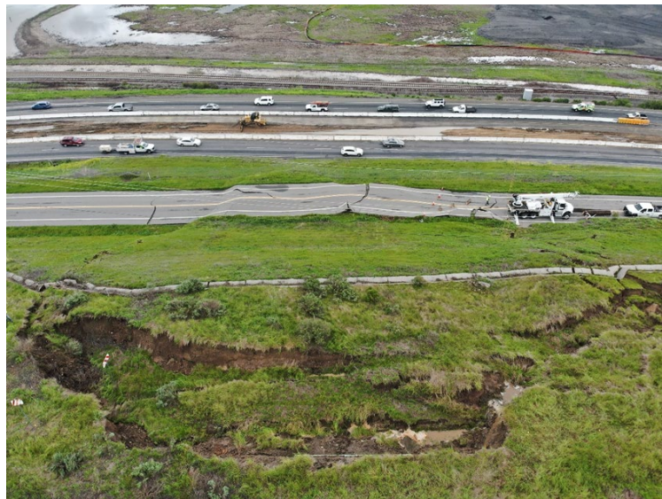
FIGURE 1-3 FIGURE L021G – NOVATO LANDSLIDE OVERVIEW
