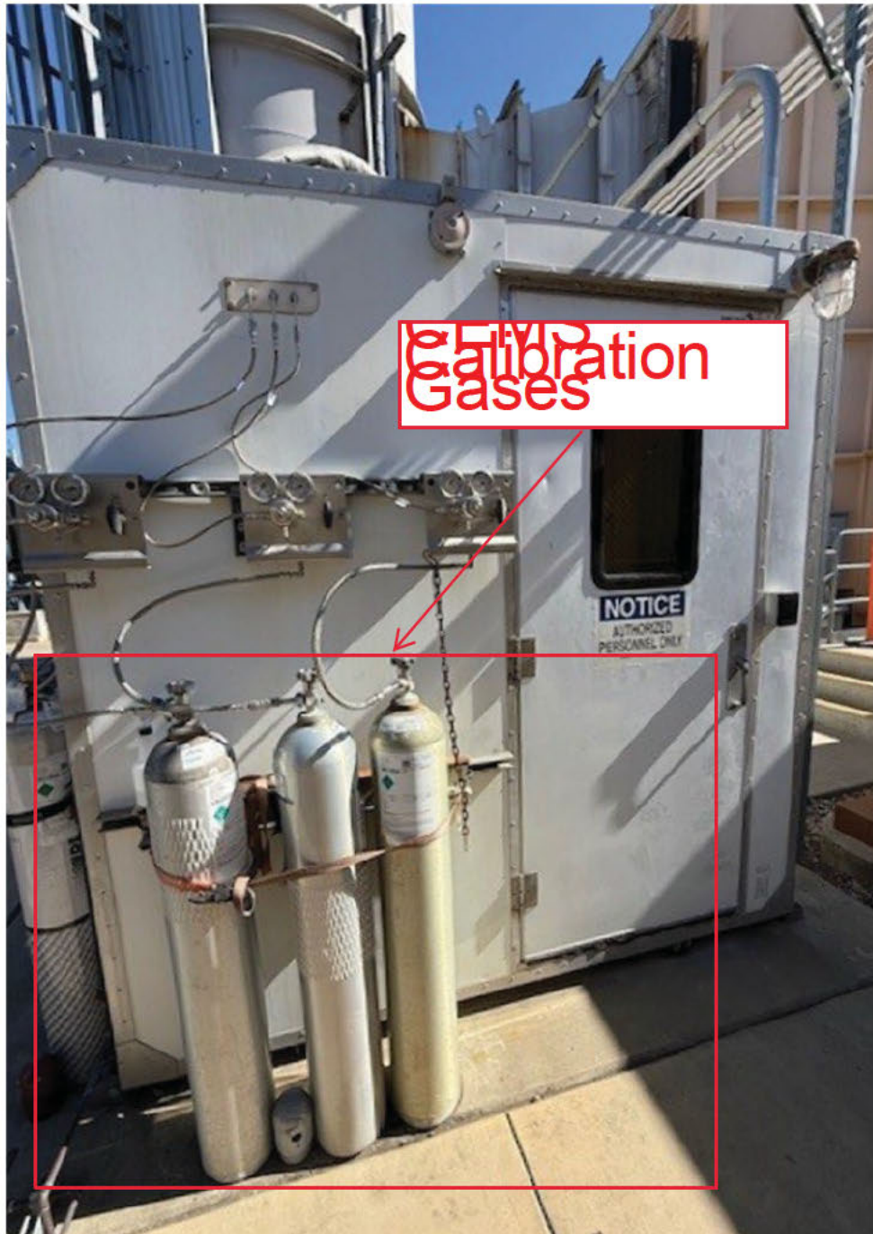
Figure 2.5 CPEP CEMS Location of Calibration Gases 165
