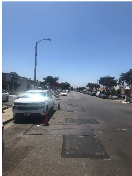
Figure 4. Recess Steel Plates over an Excavation
