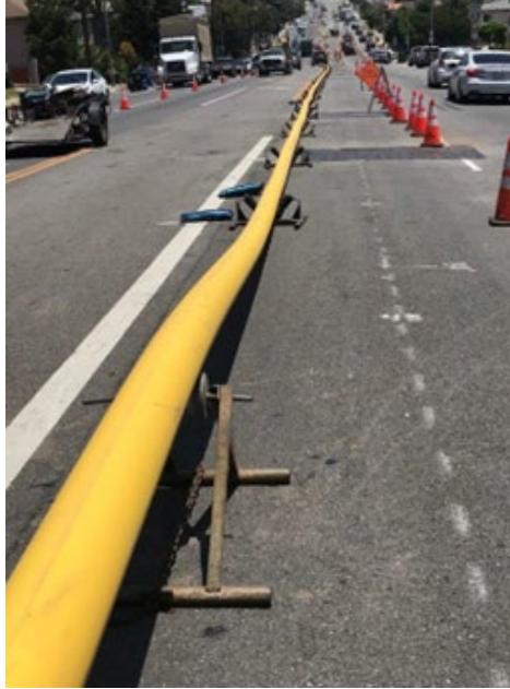
Figure 2. Trenchless Pipeline Installation Method
