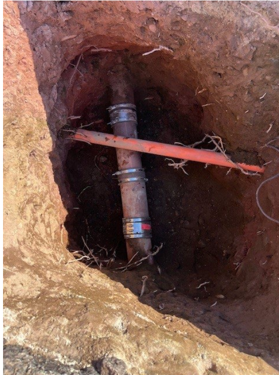
Figure 5. Repaired Cross Bore
