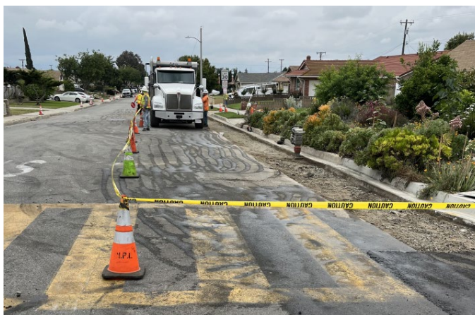
Figure 5. Removal of Asphalt During Paving
