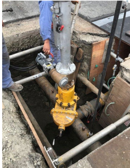
Figure 7. Installation of Pressure Control Fitting
