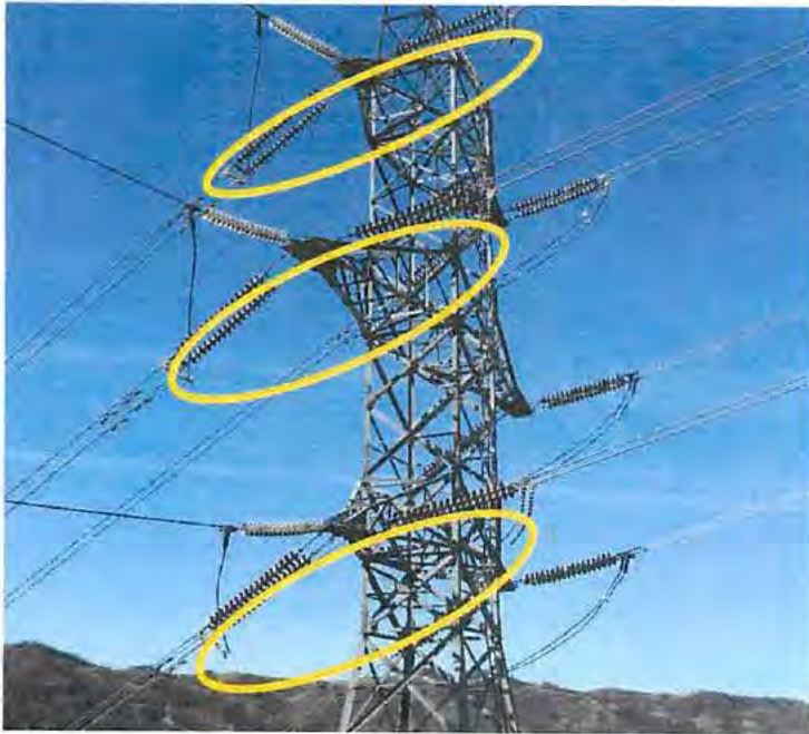
Figure 8(IMG1902.JPG.) Photo taken on May 5, 2020 by UBOLDI, G. The highlighted sections are where PG&E removed the conductor wires from tower 001/009 on the Geysers #9 – Lakeville electrical transmission line after the Kincade Fire.
