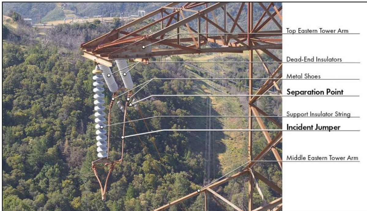
FIGURE 3A-3 TOWER 001/006 JUMPER CONFIGURATION
