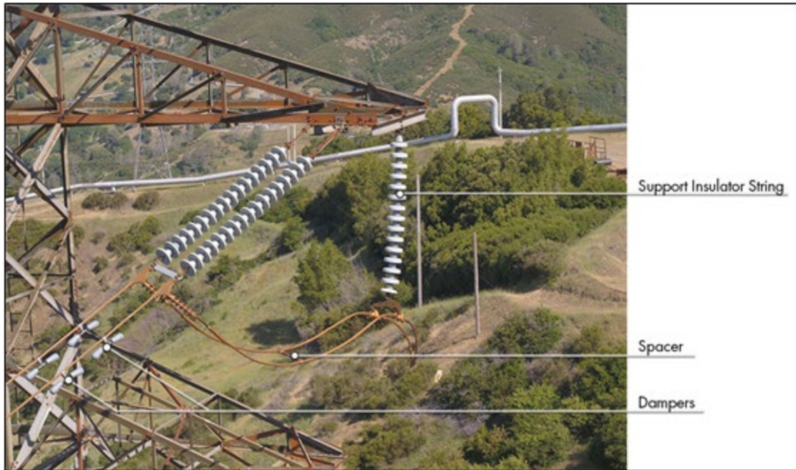
FIGURE 3A-7 WIND MITIGATIONS ON TOWER 001/006 AS OF MAY 2019
