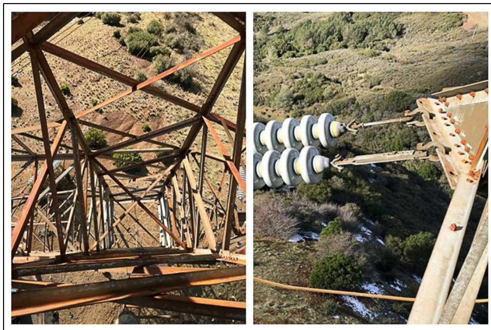
FIGURE 3A-10 ILLUSTRATIVE PHOTOGRAPHS FROM FEBRUARY 6, 2019 CLIMBING INSPECTION
