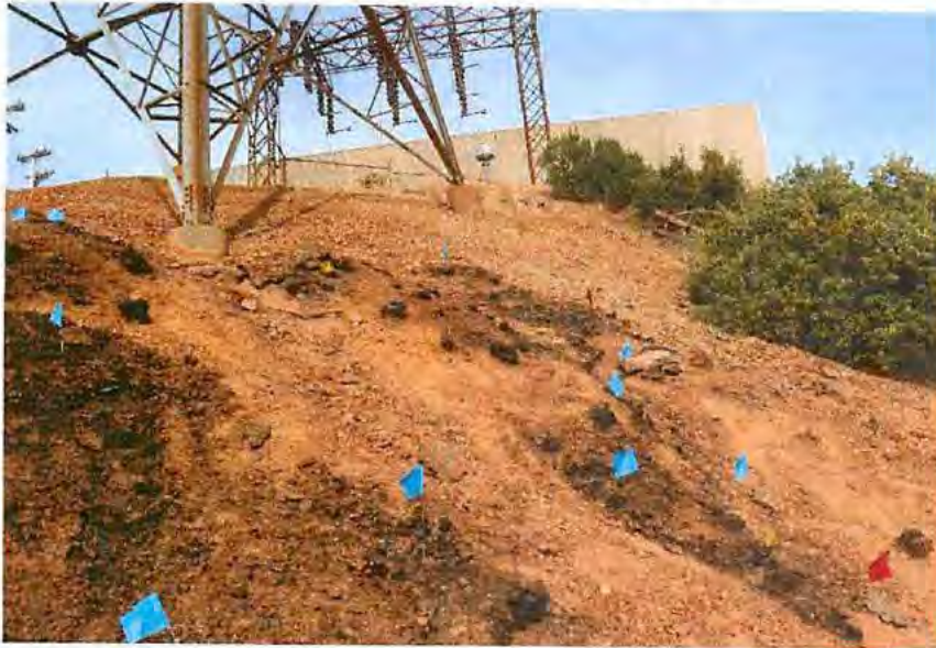
Figure 4.(IMG 1551.JPG) The general origin area (GOA) on south side of Tower 1-6 4/1/29/17
